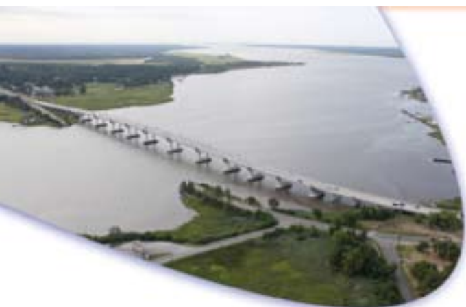
VTRC researchers contributed to the development of the Bulb-T girders on the new Route 33 bridge over the Mattaponi River at West Point.
