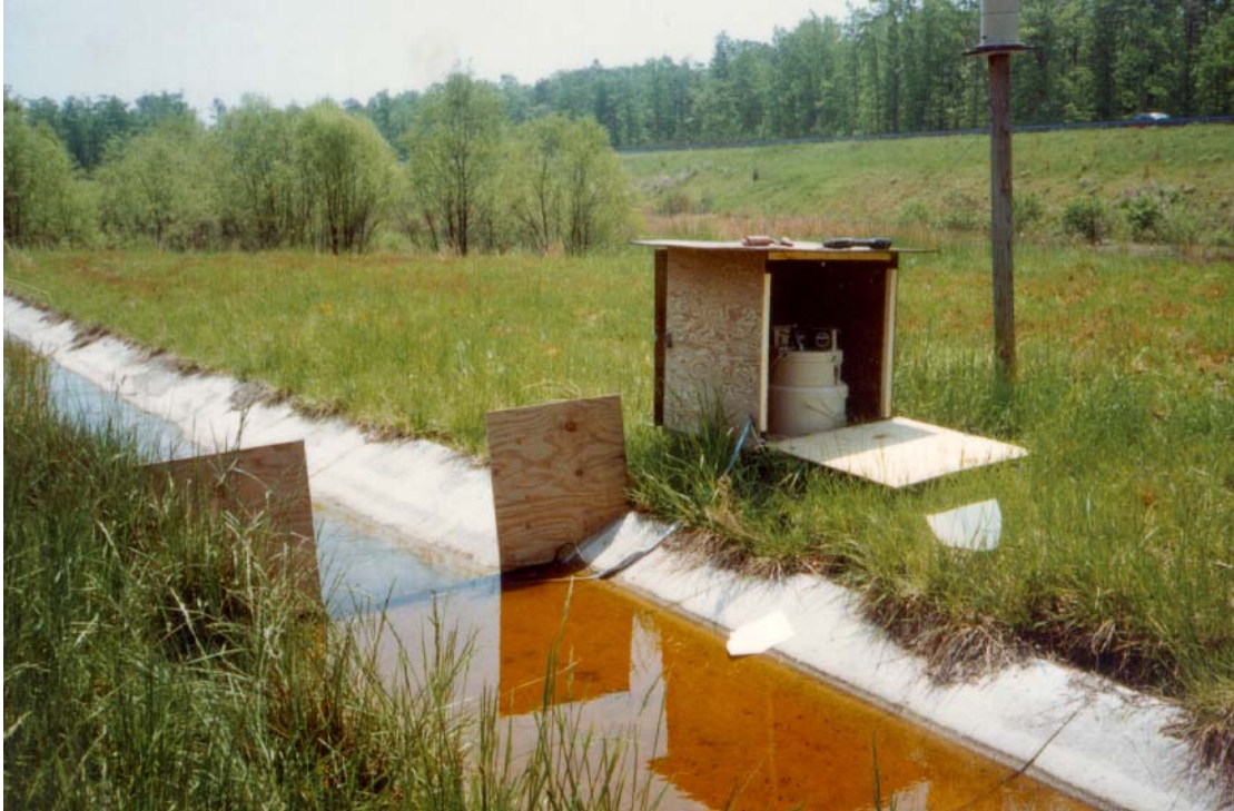
Figure 3. Inlet 1 Monitoring Station
