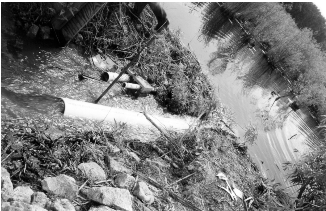
Figure 4. Outlet Pond Leveler
