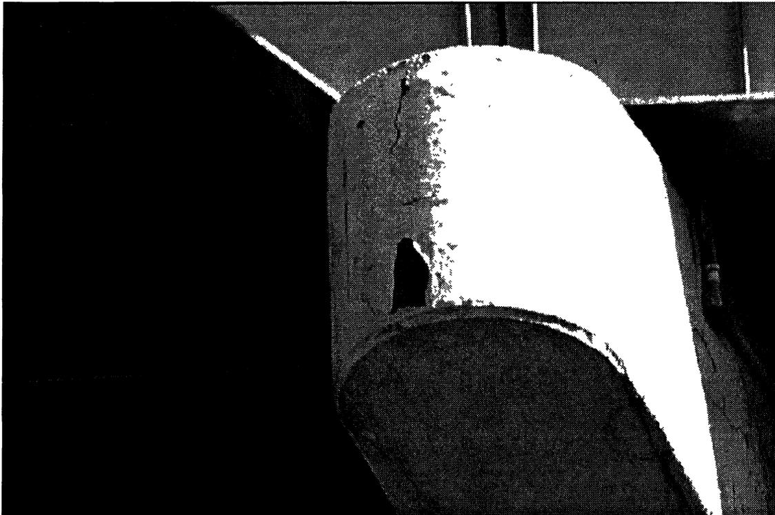
**Figure 16. Damage of Conductive-Paint Anode System at End of Pier Cap Protected by CP System 2**
