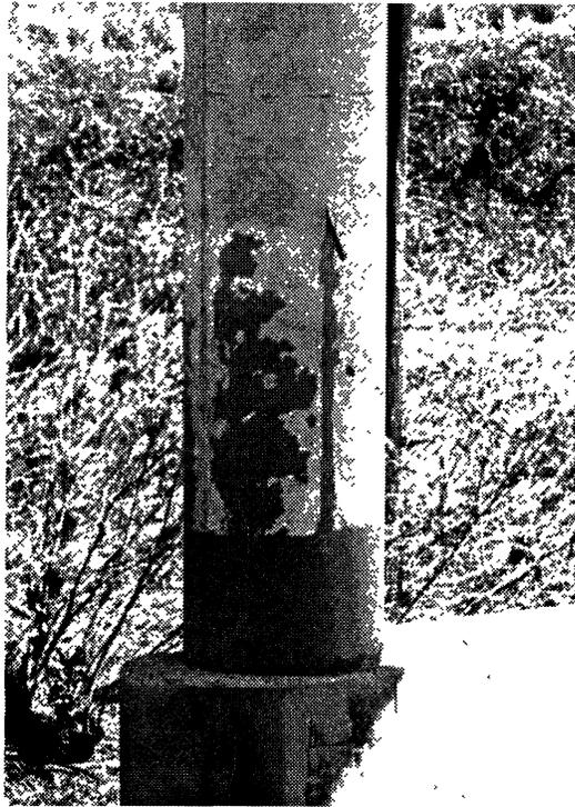
**Figure 14. Damage of Conductive-Paint Anode System on Footing of Pier Protected by CP System 1.**
