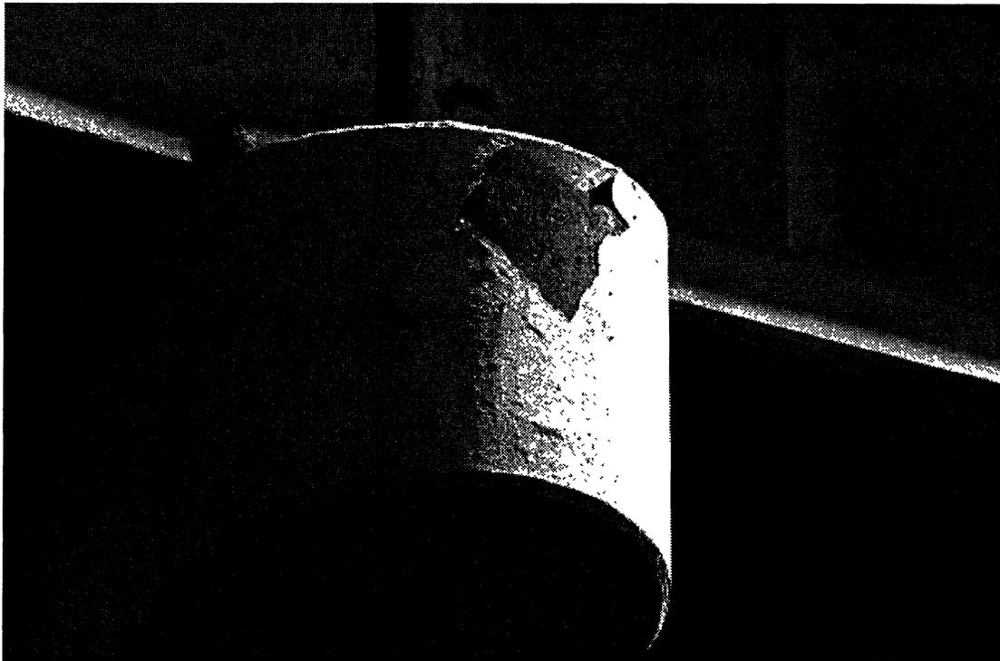
**Figure 15. Damage of Conductive-Paint Anode System at End of Pier Cap Protected by CP System 1**
