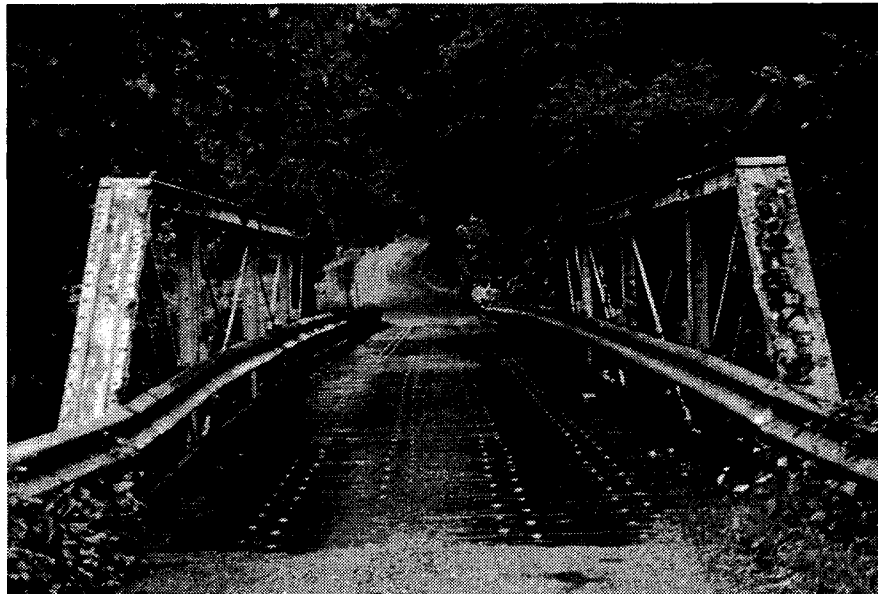
Figure B7. Rte. 671 bridge over Moormans River
