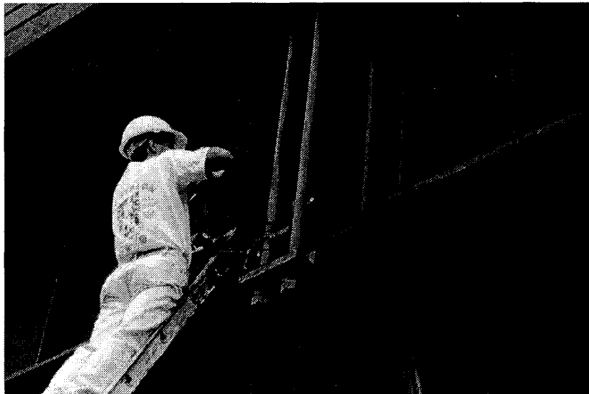
Figure B1. Pin and hanger connection, Rte. 460 bridge in Glenlyn, Virginia
