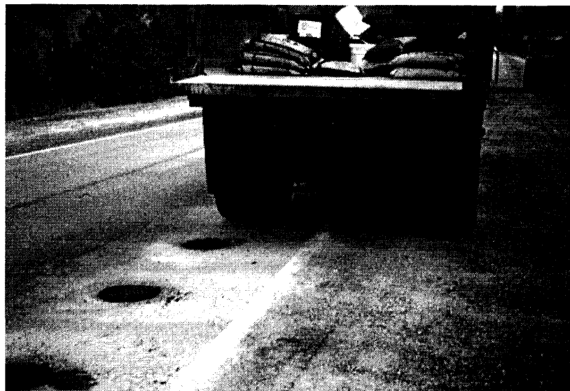
FIGURE 6. PATCHES BEING ROLLED WITH A DUMP TRUCK
