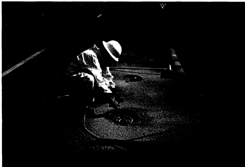
FIGURE 4. POTHOLE BEING CLEANED WITH COMPRESSED AIR
