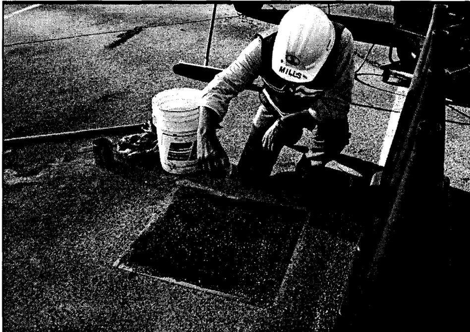
Figure 149. Silica sand is broadcast onto the final layer of epoxy of the test patch. The patches should be constructed with the same materials and equipment that will be used for the full scale overlay. Also, they should be constructed under the same conditions if practical.
