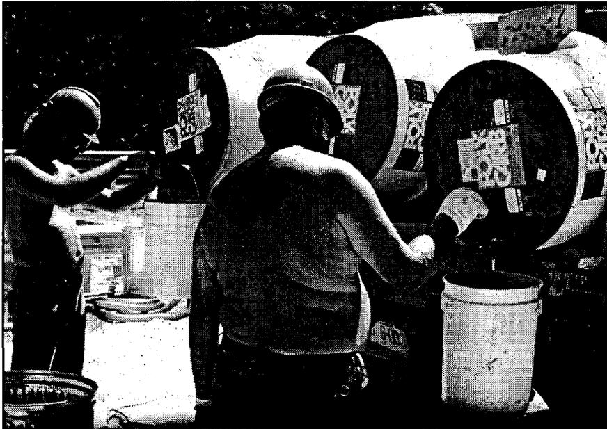
Figure 155. Binders for epoxy concrete overlays are usually 1 to 1 or 2 to 1 mixtures. Care should be taken to carefully measure out the desired quantities of component A and component B. Individual components should be mixed prior to being dispensed into calibrated containers. Protective clothing should be worn so that epoxy does not make contact with the skin.
