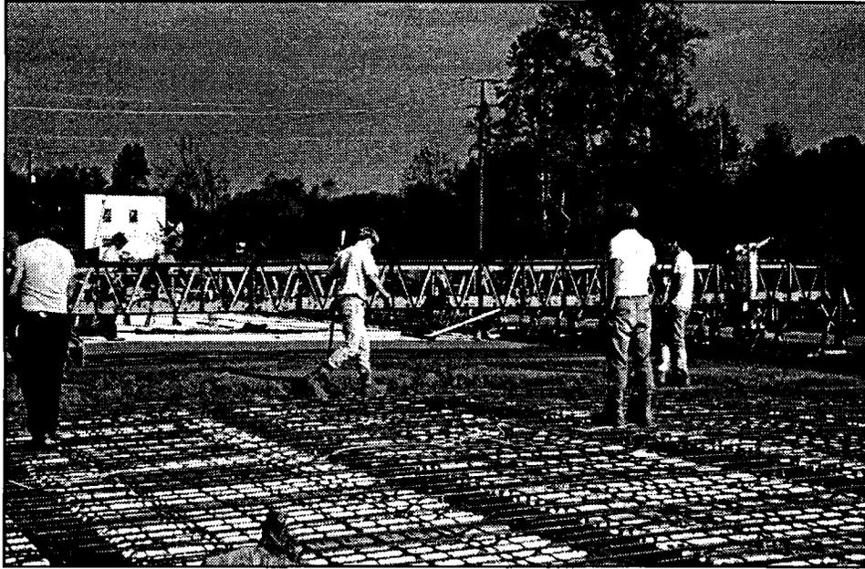
Figure 98. Placement of concrete to widen a bridge deck. Silica fume, fly ash and slag are being used in concrete to reduce the lifecycle costs, to obtain high early strengths (silica fume), and to utilize materials that might have to be placed in landfills.
