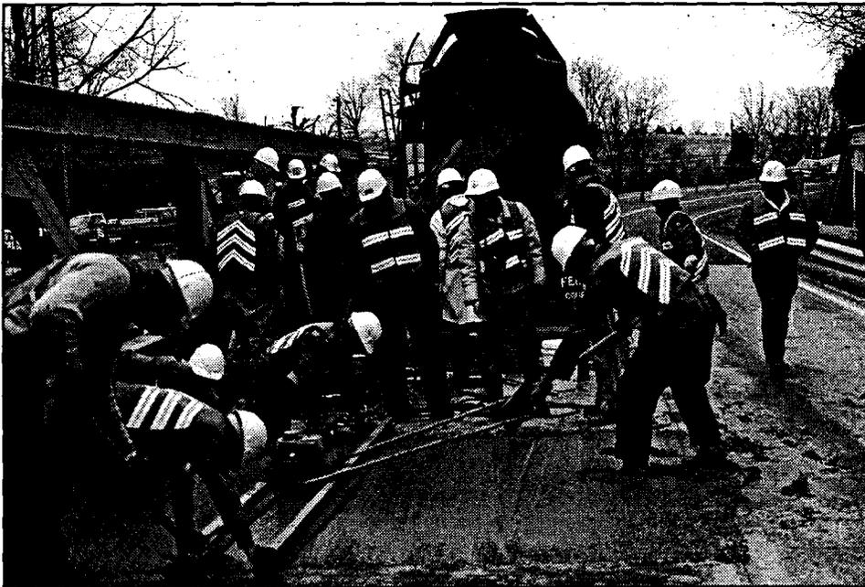
Figure 79. The hydraulic cement concrete shall be properly consolidated with internal vibrators and a vibrating screed may be used to strike off the surface.
