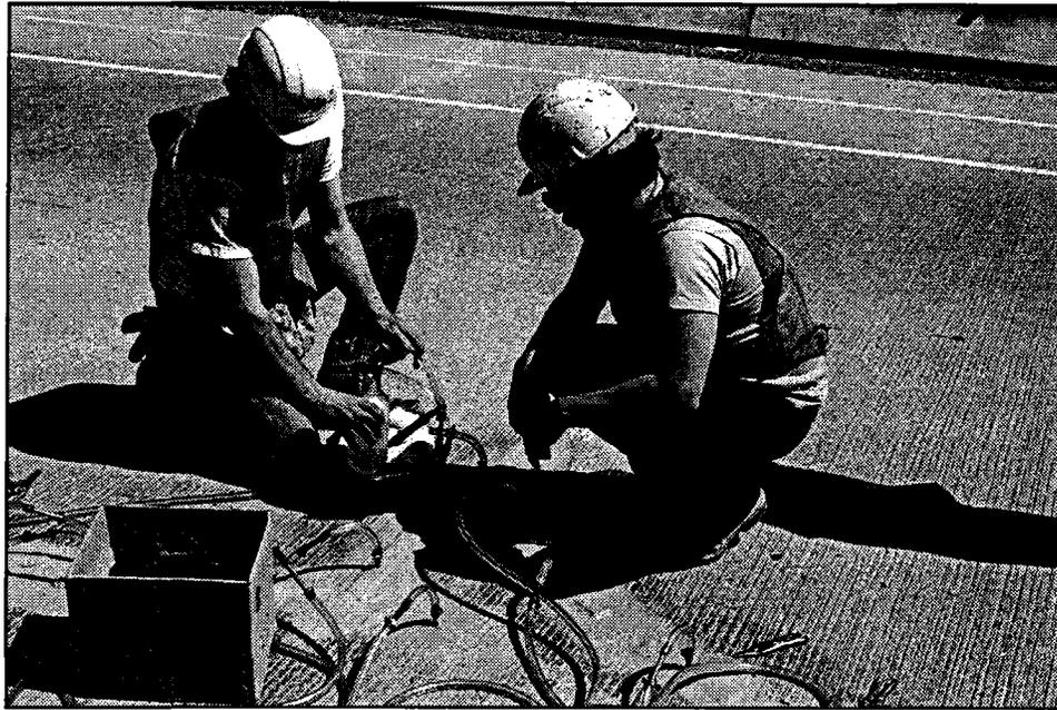
Figure 114. Vacuum injection can be used to fill cracks with a methacrylate resin. Prior to introducing the resin, steel entry ports should be placed on the crack surface, the cracks are covered above and below with a viscous paste-like epoxy, and a vacuum is applied to the cracks through the ports. The requirements for successful filling of a crack cited under Figure 107 are also generally applicable to vacuum injection.
