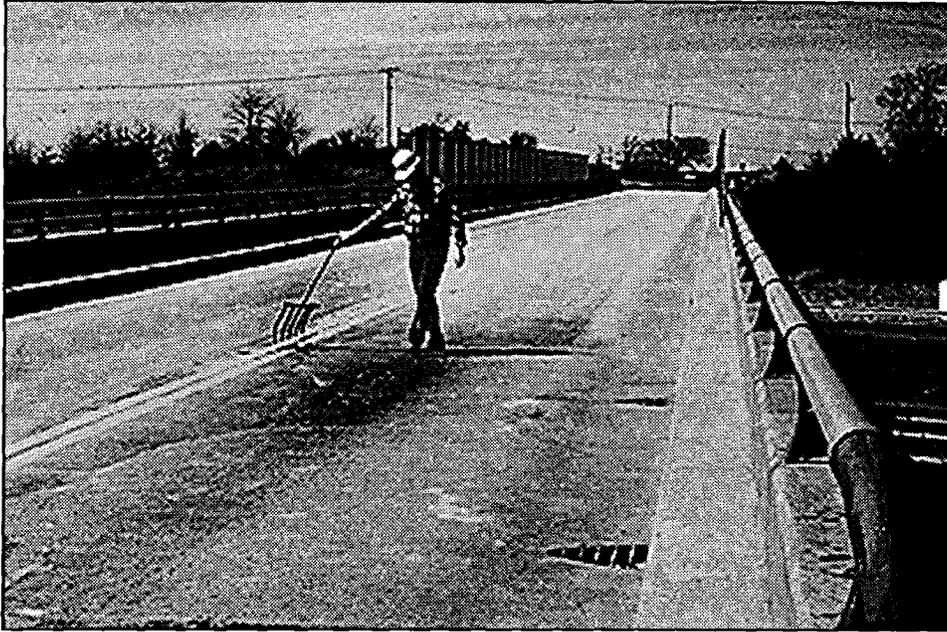
Figure 15. Several chains hanging from a pipe (chain drag) can be dragged over the deck surface to locate delaminated and very unsound concrete. Noise from traffic can interfere with the use of the chain drag.
