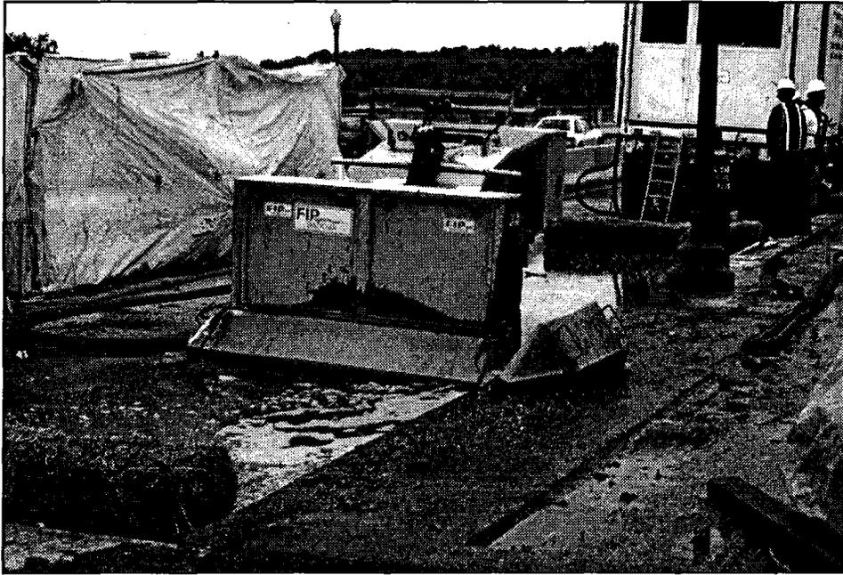
Figure 64. A high pressure water jet moves from left to right inside the blasting unit, thereby removing concrete with a strength that is lower than the pressure of the water. The jet must be calibrated to give the desired depth of removal.
