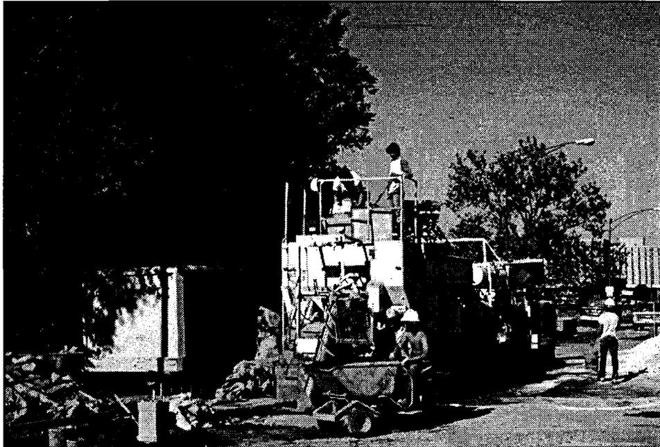
Figure 137. Low-slump concrete is batched at the job site like latex-modified concrete. The design slump is 0.75 in. with a maximum of 1.0 in.
