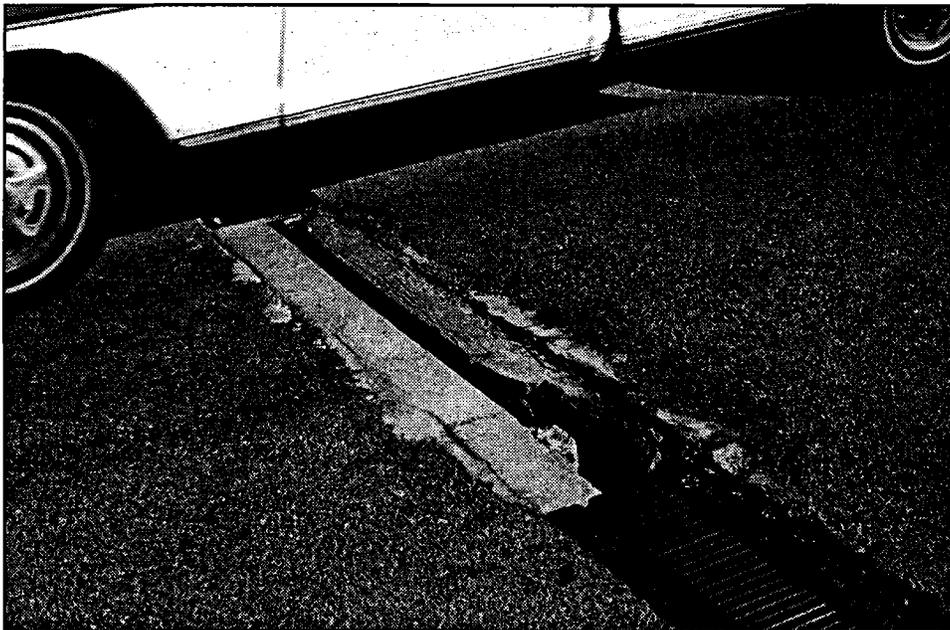
Figure 115. Joints in bridges must be repaired to prevent chlorides and water from reaching beams and substructure elements, to prevent incompressible materials from restricting movement, and to provide a smooth and safe riding surface.
