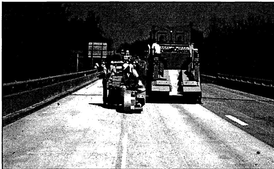
Figure 61. Shotblast equipment is available in a range of sizes. Units that blast a 9-in-wide strip and a 6-ft-wide strip are shown above.
