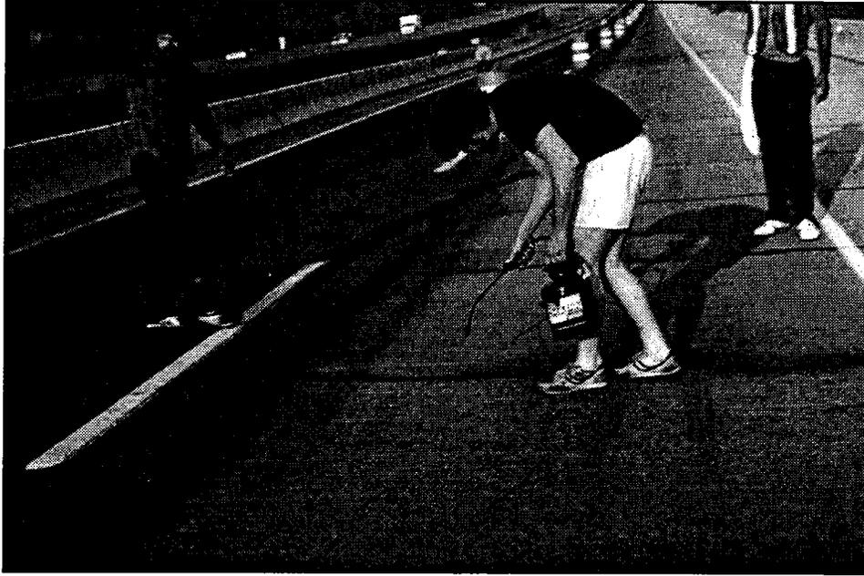
Figure 108. A pressurized spray can be used to apply high molecular weight methacrylate resin to a crack. For best results, a brush should be used to work the resin into the crack. Protective clothing should be worn to keep the resin off of the skin.
