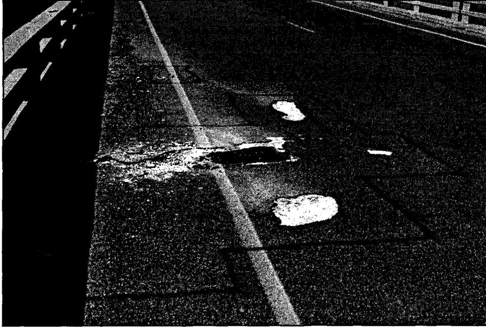
Figure 54. The area over which the concrete is to be removed should be "squared up" and marked with paint.
