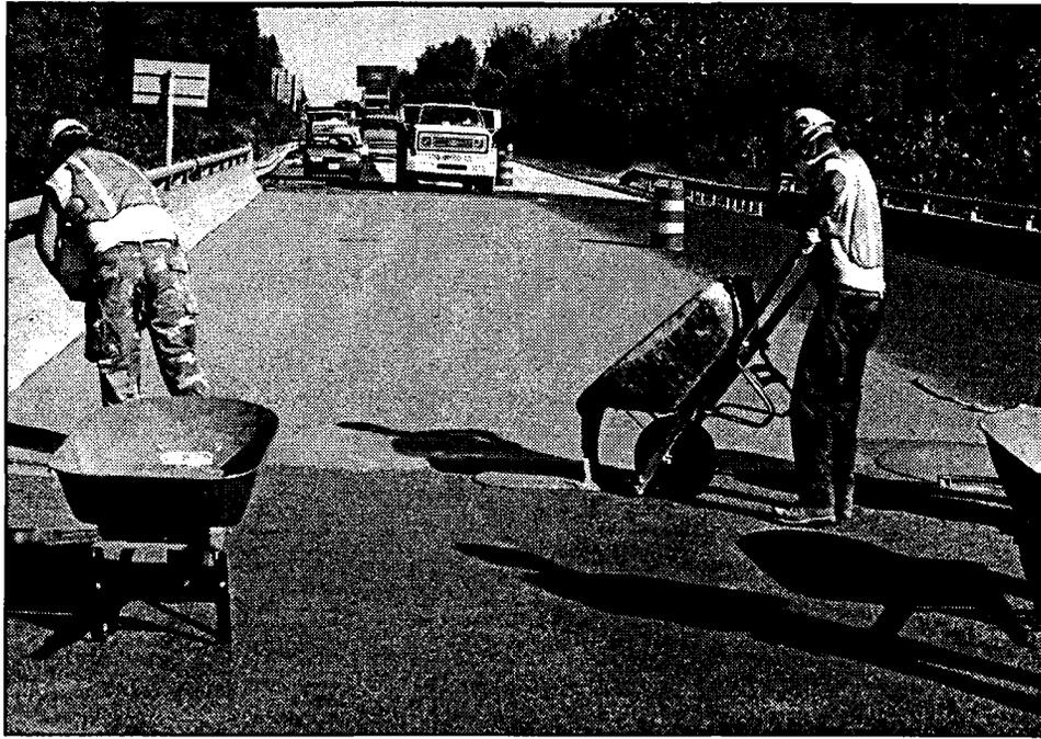
Figure 166. Methyl methacrylate aggregate slurry mixed with mortar mixers is here applied to shotblasted surface that was primed at least 1 hour earlier with a methyl methacrylate primer. The primer must be cured prior to placing the slurry.
