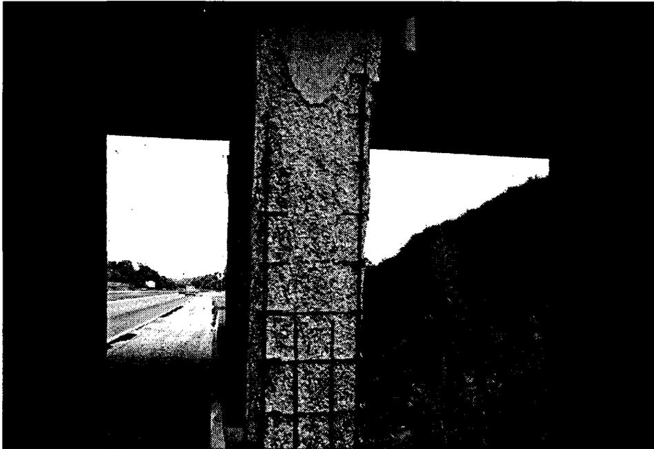
Figure 117. Corrosion induced spalling on a pier caused by chlorides leaking through a joint.
