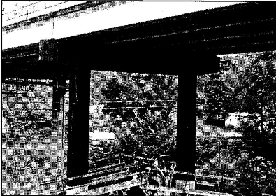
Figure 189. A conductive coating has been applied to the piers and bent to provide applied current cathodic protection.
