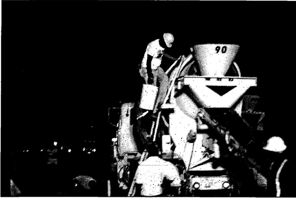
Figure 134. Silica fume concrete is typically batched at a ready-mix plant. The condensed silica fume is usually added to the mixer first so that it is dispersed over the inside of the drum. Water, aggregates, admixtures, and cement are added and mixed. Additional high range water reducing admixture is sometimes added at the job site to increase the workability of the concrete.
