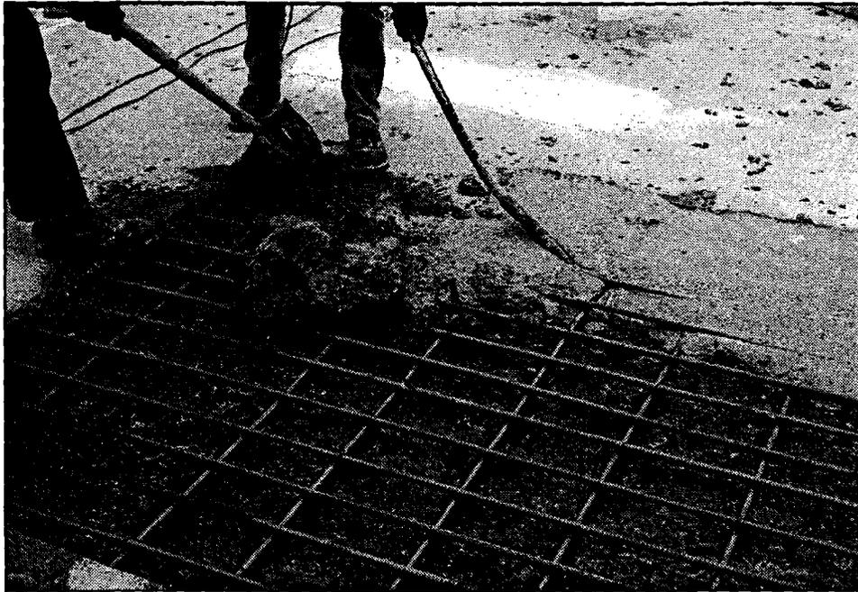
Figure 84. Very rapid hardening hydraulic cement concrete may appear stiff prior to being consolidated. Internal vibration rather than additional mix water should be used to achieve good consolidation of the concrete.
