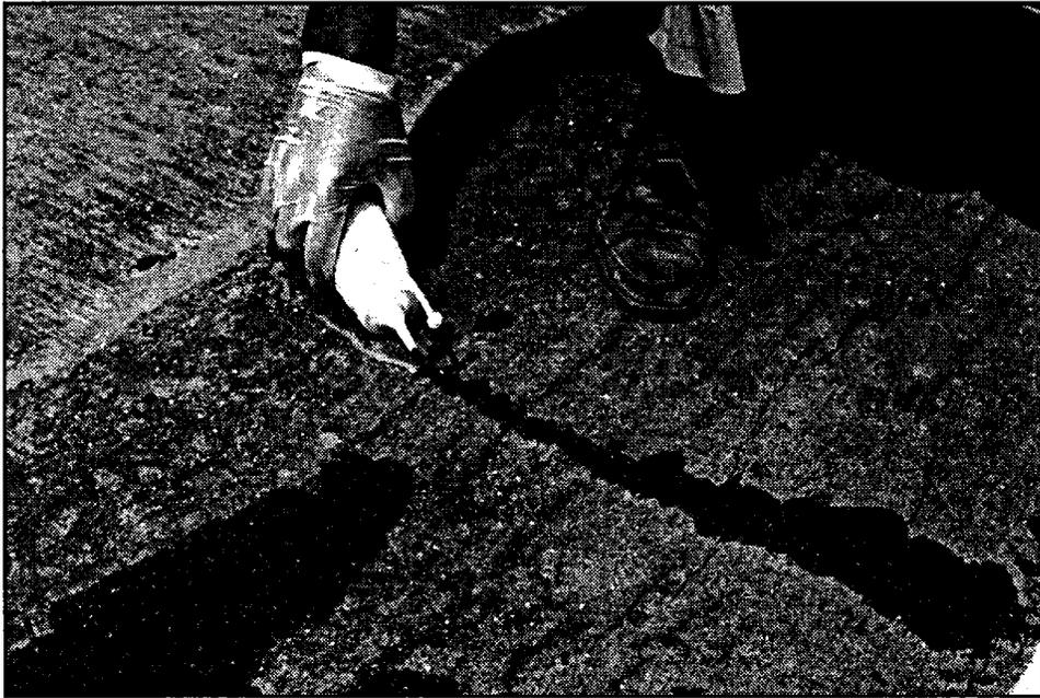
Figure 107. High molecular weight methacrylate can be applied to a crack. For satisfactory filling of the crack, it should be free of debris and wider than 0.1 mm. Also, best results can be obtained by filling cracks when they are open the widest at the surface (temperatures between 55°F and 70°F and between 1:00 a.m. and 10:00 a.m.). High molecular weight methacrylate will not cure satisfactorily at temperatures below 55°F.
