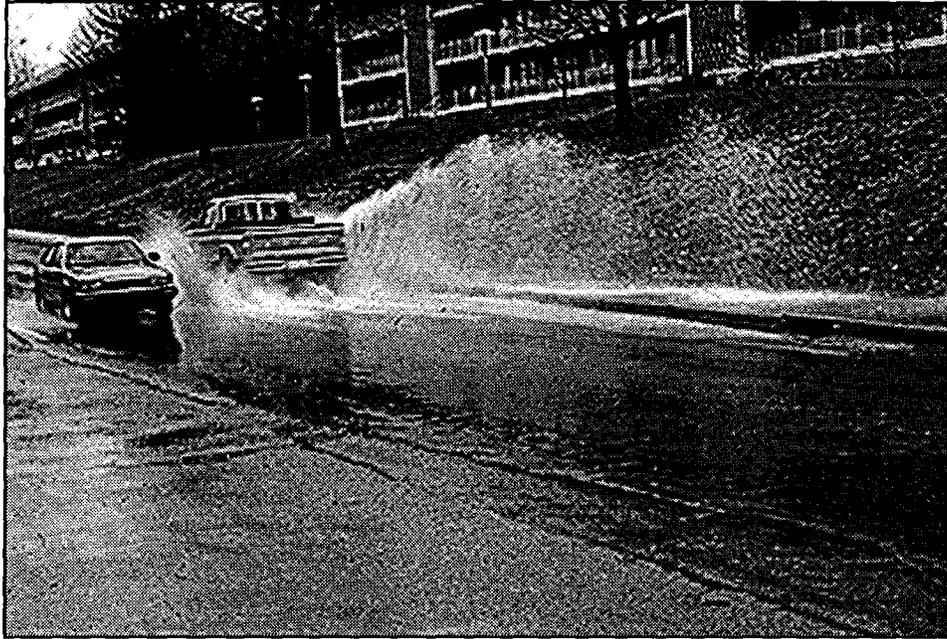
Figure 7. A plugged or improperly located drain (shown above) does not provide for proper drainage. Poor drainage allows water and salt to pond on the surface and to saturate the concrete, which provides ideal conditions for freeze and thaw damage in the concrete and creates high salt concentrations at the reinforcing steel.
