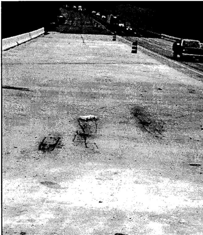
Figure 101. Concrete in the center span is cracked full depth because white pigmented liquid membrane curing material was not applied in sufficient quantities.
