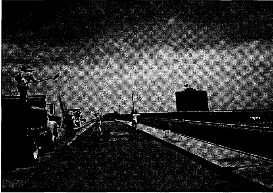
Figure 164. Basalt aggregate is broadcast from a dump truck in the adjacent lane as a multiple-layer epoxy overlay is constructed
