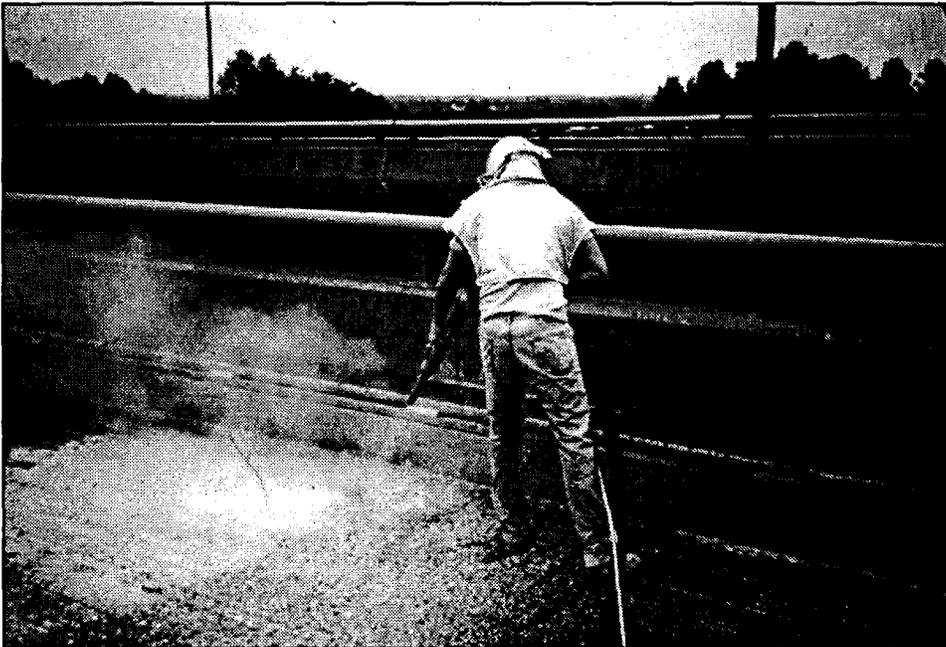
Figure 59. Sandblasting (typically with slag rather than sand) can be used to remove carbonation, laitance, weak surface mortar, and other materials that may be detrimental to the bonding of the overlay or the patching material.
