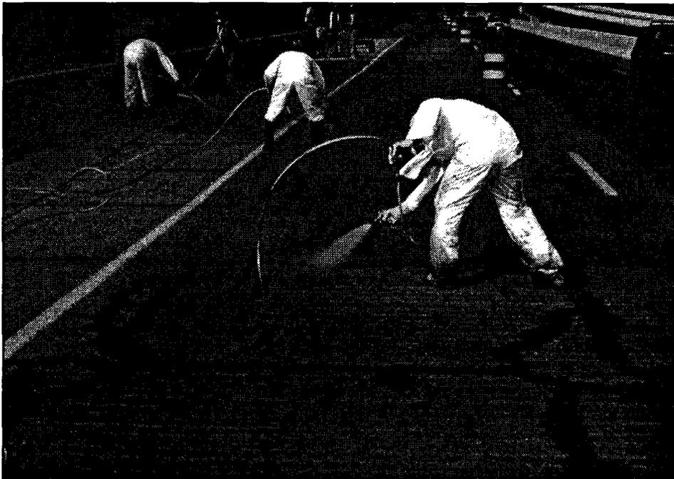
Figure 183. A sealer can be applied with an airless sprayer. Note that the spray gun operators are wearing impermeable boots, gloves, coveralls and canister masks. Care should be taken to protect traffic from the spray. Silanes and siloxanes are typically used to seal bridge deck concrete.
