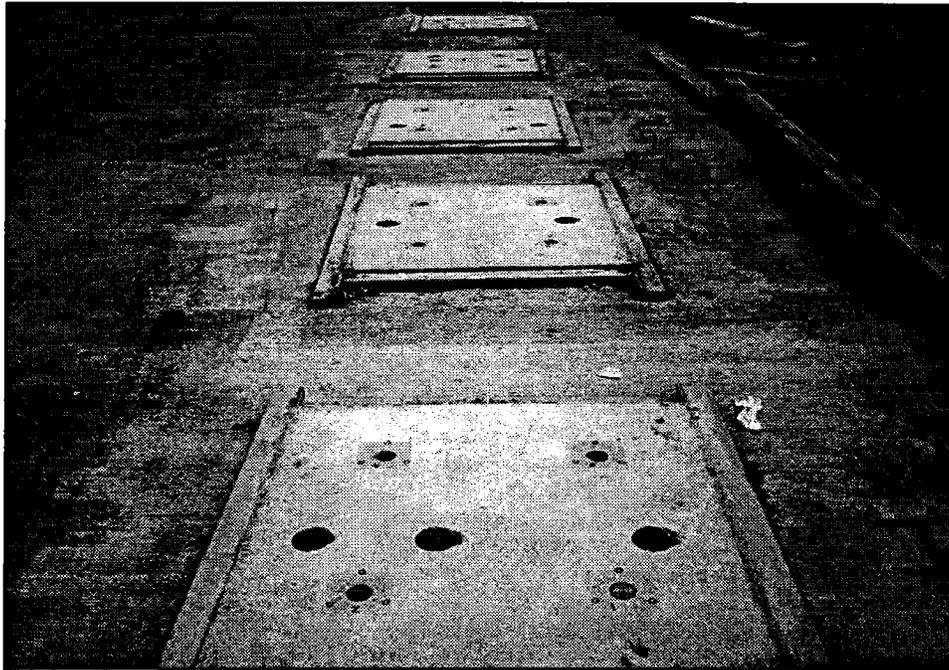
Figure 140. Prior to placing an overlay on a major bridge, test panels of candidate overlay mixtures should be installed so that problems with surface preparation, mixture proportions, placement, and curing procedures can be identified.
