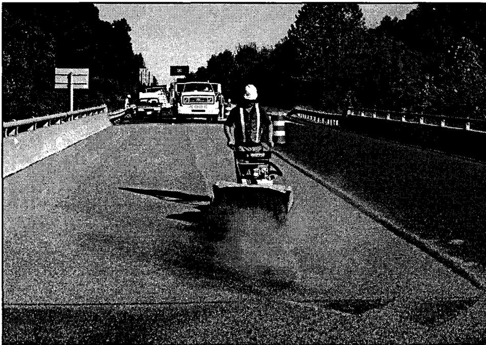
Figure 163. A mechanical sweeper can be used to remove excess aggregate prior to placing the second layer or opening the second layer to traffic.
