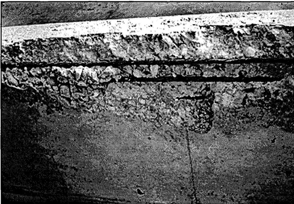
Figure 48. Prestressed strands are corroded and concrete is not properly consolidated in spalled areas of beam.
