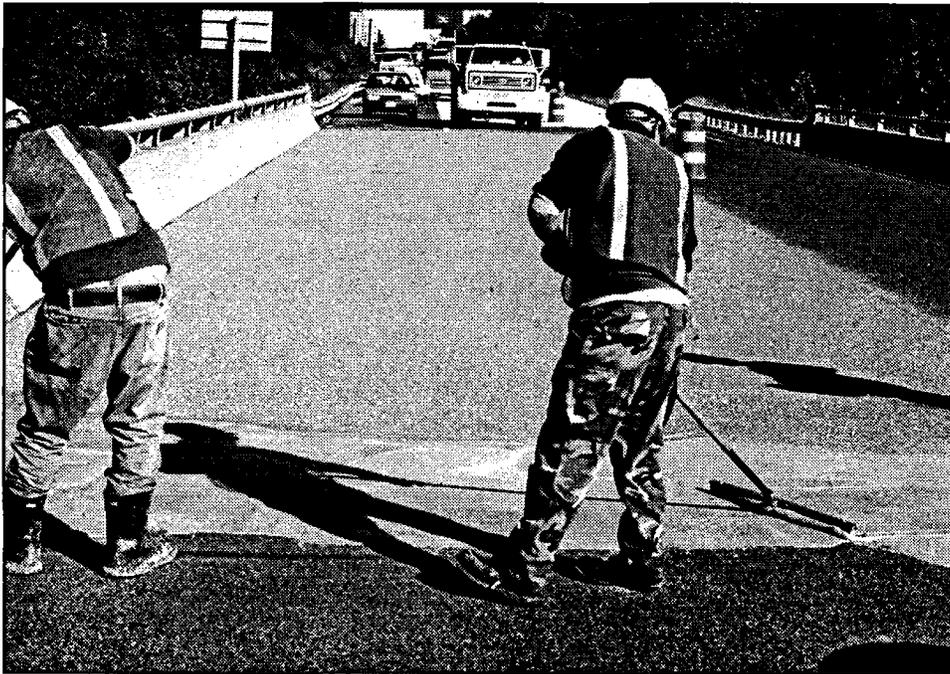
Figure 167. A methyl methacrylate slurry overlay should be struck off with gage rakes set to provide a  $3/16$  in thick layer of slurry.
