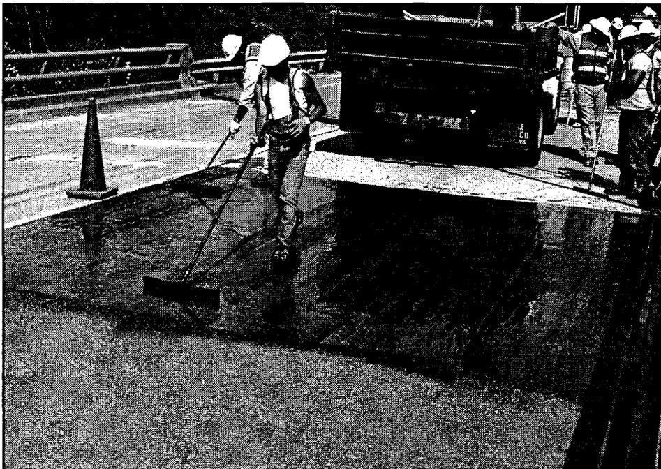
Figure 147. A multiple layer epoxy overlay consists of two layers of epoxy and aggregate. An epoxy mixture is here spread over the deck with notched squeegees. Basalt aggregate is here broadcast to excess from the back of a dump truck.
