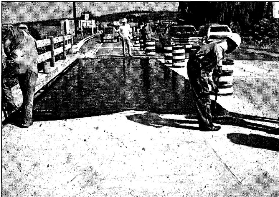
Figure 177. Squeegees can be used to apply a primer to a shotblasted deck prior to placing the prefabricated membrane for Class II waterproofing.
