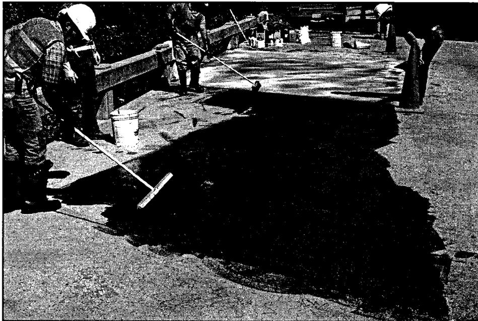
Figure 105. High molecular weight methacrylate resin can be applied to the surface of a bridge deck with brooms to fill random cracks such as those caused by plastic shrinkage. An effort should be made to brush the resin into the cracks until the cracks appear to be filled by the brooming action and the force of gravity.
