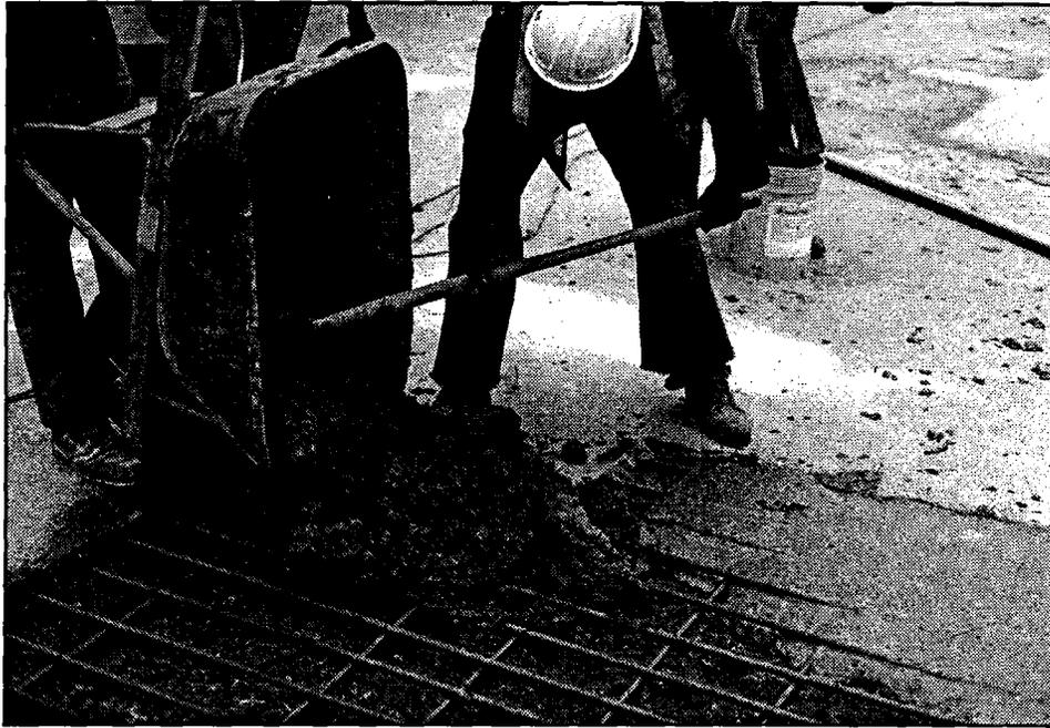
Figure 82. The mixed concrete is usually transported to the patch site with a wheelbarrow. Internal spud vibrators must be used to consolidate the concrete. The mixture should have a slump of 2 to 4 in. and should not segregate when consolidated. The hardened concrete surface should be wetted to achieve a saturated-surface-dry condition prior to placing the fresh concrete.
