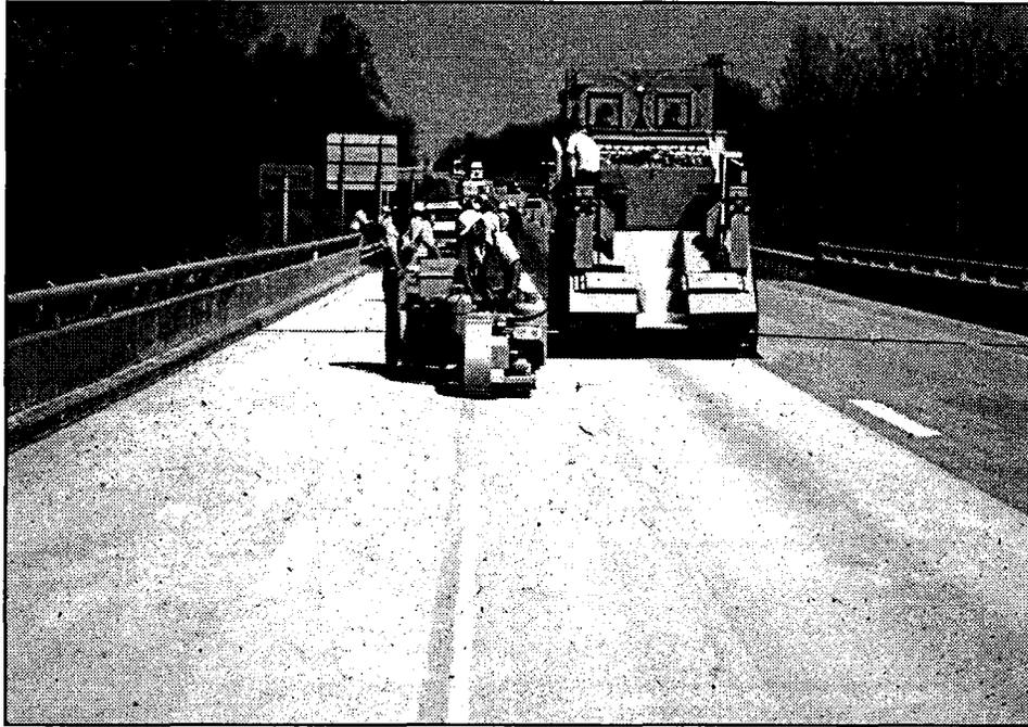
Figure 146. The first step toward the successful placement of a polymer concrete overlay is to shot blast the concrete surface. Shot blast equipment is available in a range of sizes. Units that blast a 9-in-wide strip and a 6-ft-wide strip are shown above.
