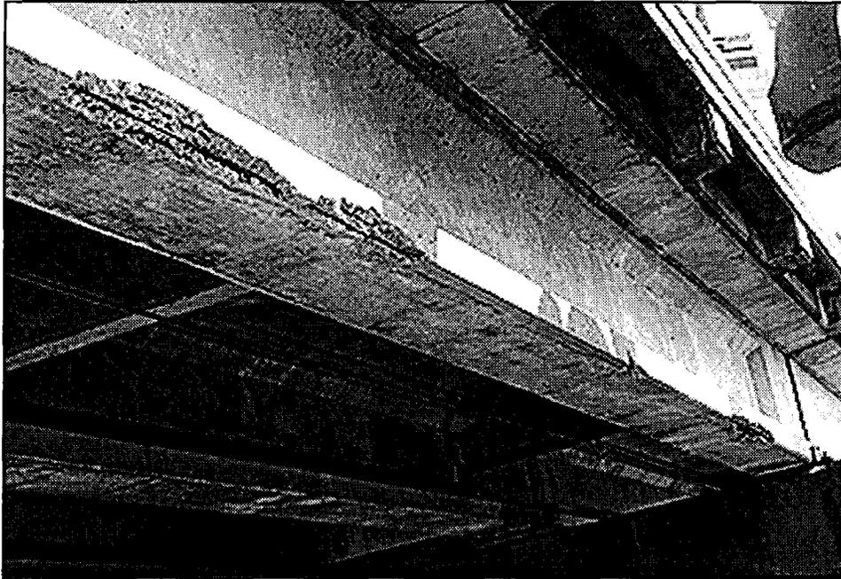
Figure 47. Spalling deterioration on a 30 year old prestressed concrete beam bridge.
