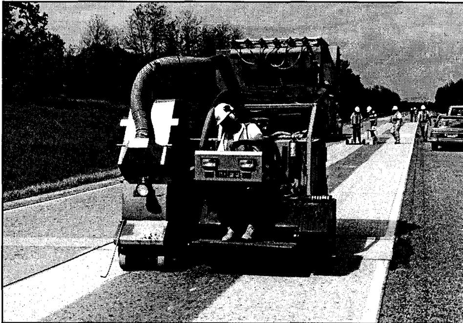
Figure 181. Sealers are sometimes applied to concrete to reduce the infiltration of water and chloride ions. Prior to placing the sealer, the concrete should be shot blasted to remove material that may interfere with the penetration, curing and bonding of the sealer.
