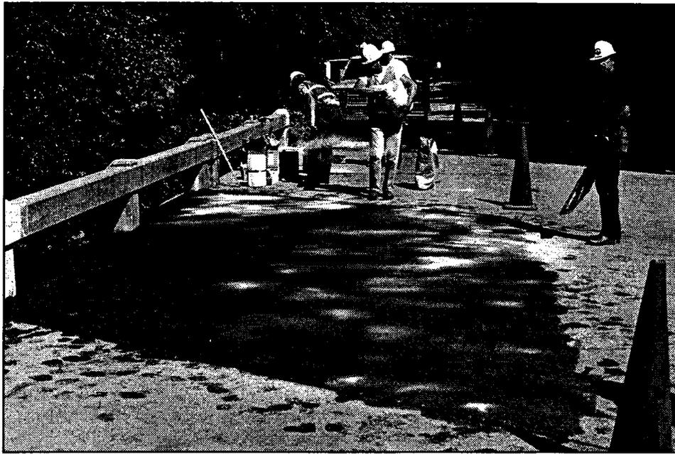
Figure 106. Sand must be broadcast onto the resin to provide an acceptable skid number. The sand may be omitted if the resin is applied to a grooved or tined surface, but care must be taken to ensure that the resin does not fill the grooves.
