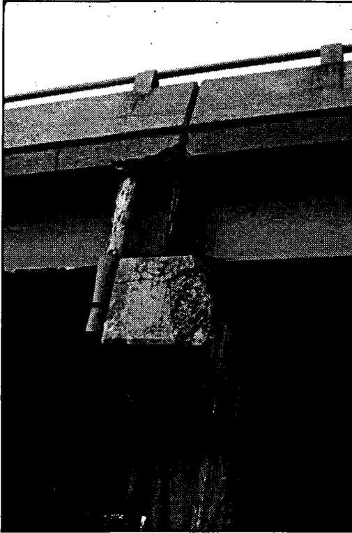
Figure 116. Deterioration of concrete caused by water and chlorides leaking through a joint.
