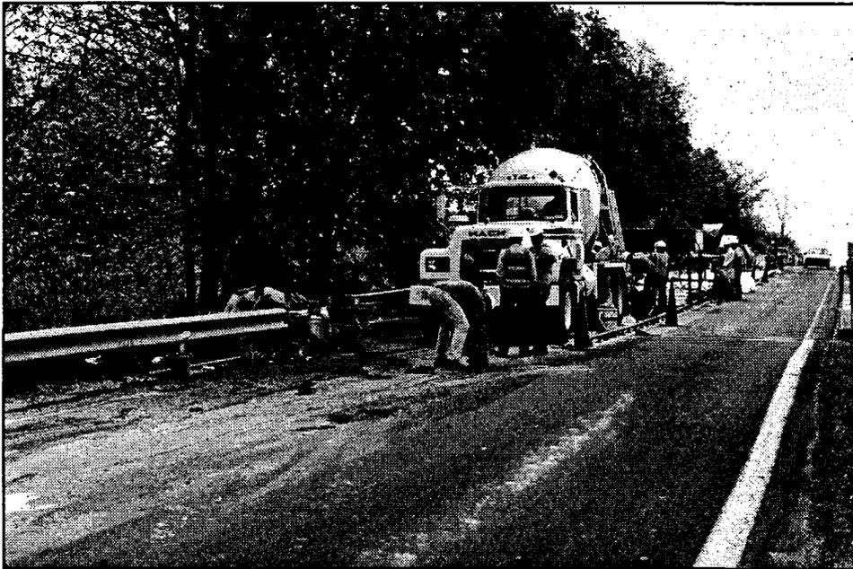
Figure 133. Silica fume concrete is mixed in a ready-mix truck and deposited onto a bridge deck surface that has been prepared the same way as the surface is prepared for a latex-modified concrete overlay (see Figure 125).
