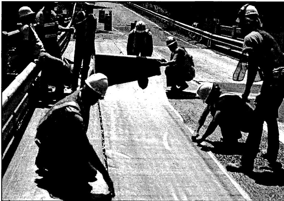
Figure 179. A prefabricated membrane which adheres to the shot blasted deck is here placed.
