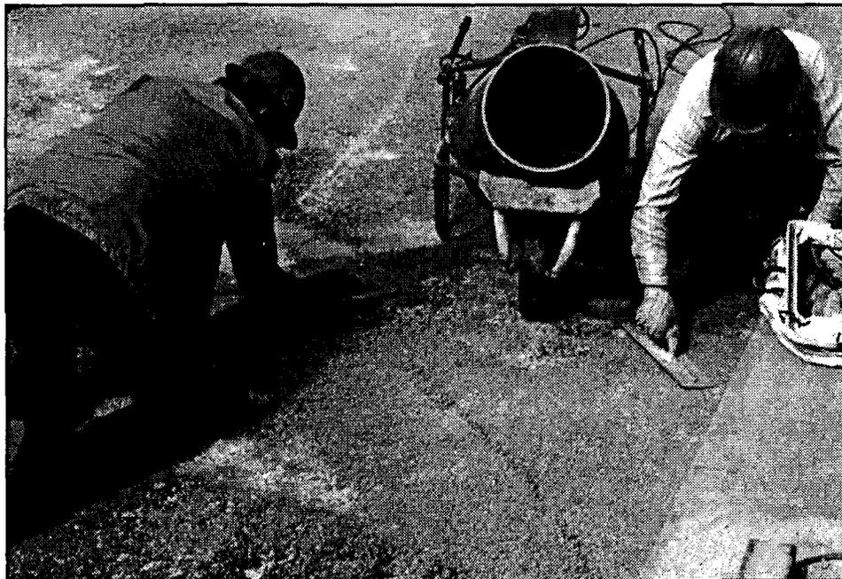
Figure 73. Areas to be patched with epoxy mortar shall be dry and shall be primed with neat epoxy prior to placing the mortar.
