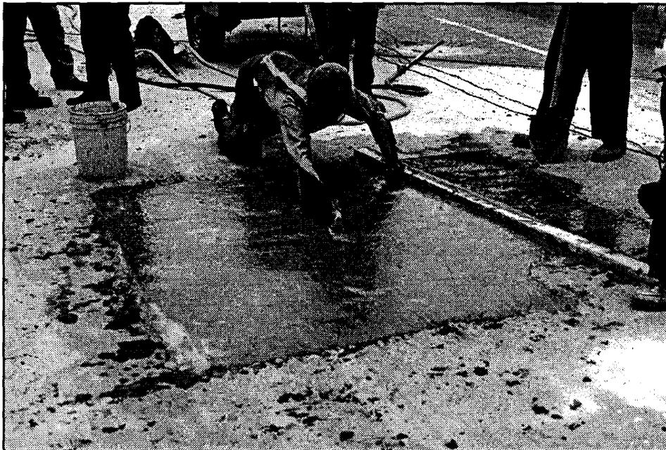
Figure 83. The concrete may be struck-off with a straight edge. When several batches are used to fill a large patch, the concrete should be struck off as each batch is placed.
