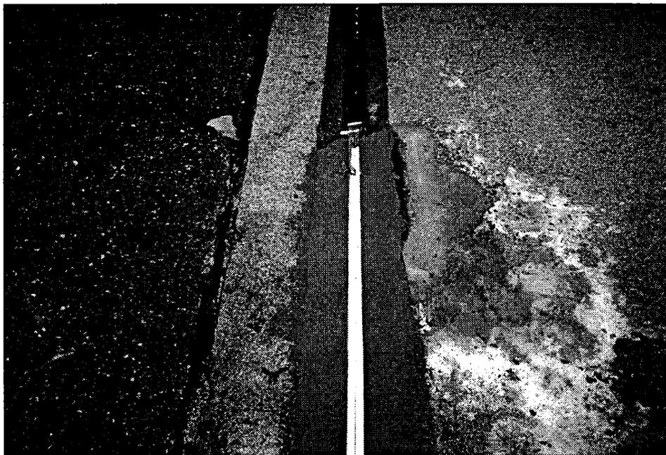
Figure 121. A joint is replaced with polymer concrete headers. Once the polymer concrete has cured the center styrefoam form is removed, adhesive is applied to the walls of the headers, and a pressurized joint seal is installed.
