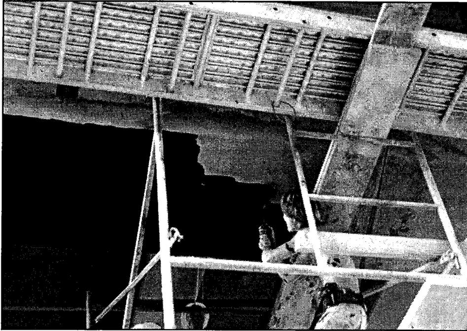
Figure 188. A conductive coating is here applied to the underside of a pier bent to provide applied current cathodic protection.
