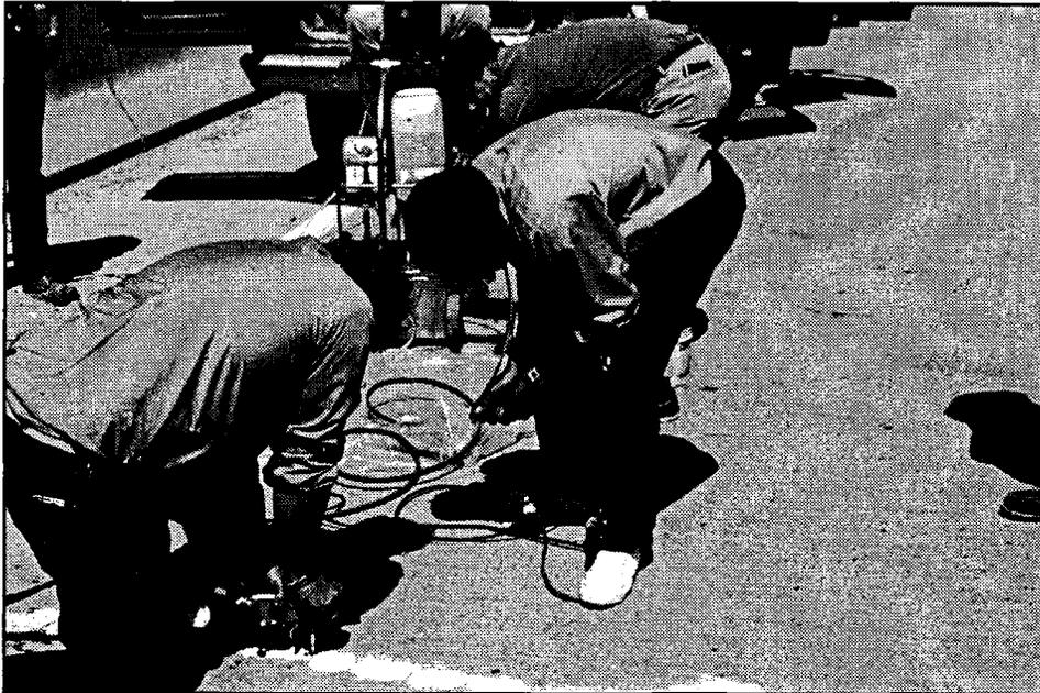
Figure 113. A two-component epoxy is here injected into a crack under pressure. Prior to injecting the epoxy, the crack should be covered above and below with a viscous paste-like epoxy and injection ports should be spaced at a distance equal to the depth of the crack to be injected. The requirements for successful filling of a crack cited under Figure 107 are also generally applicable to pressure injection.
