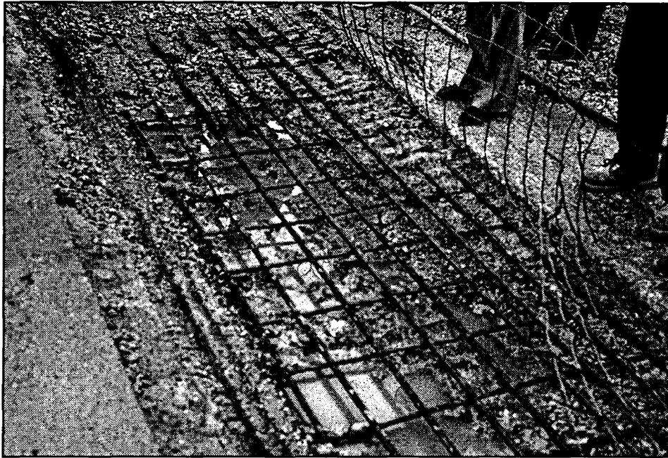
Figure 66. Concrete can be dislodged and reinforcement can be cleaned by hydro demolition. The dislodged concrete and water must be removed from the surface prior to placing the overlay or repair material. Vacuums, shovels, and air blasting have been used to remove contaminants. Proper containment and disposal of blast water and concrete rubble is necessary.
