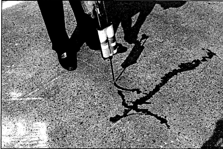
Figure 110. A two component, rapid curing, urethane, gravity fill monomer is applied to cracks using a double cartridge gun.
