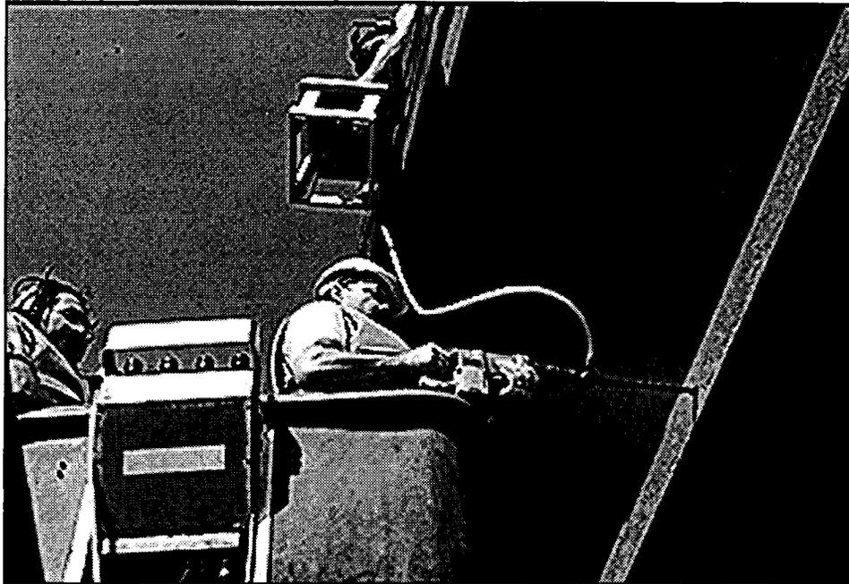
Figure 51. Vacuum chloride sampling equipment is used to take concrete samples from the side of the prestressed concrete beam.
