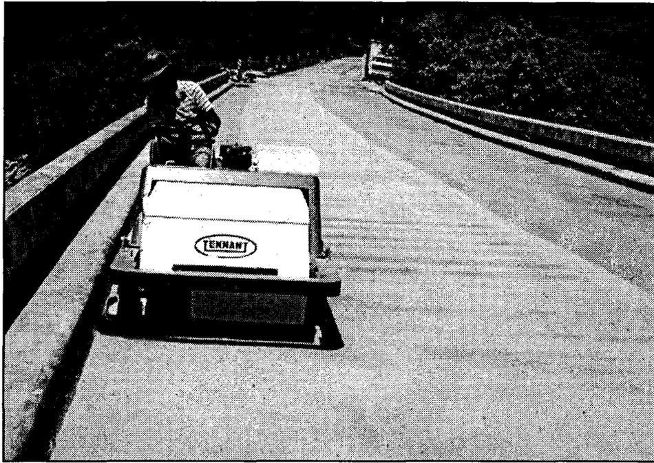
Figure 162. A sweeper-broom type vacuum truck can be used to remove excess aggregate prior to placing the next layer of a multiple-layer epoxy overlay.
