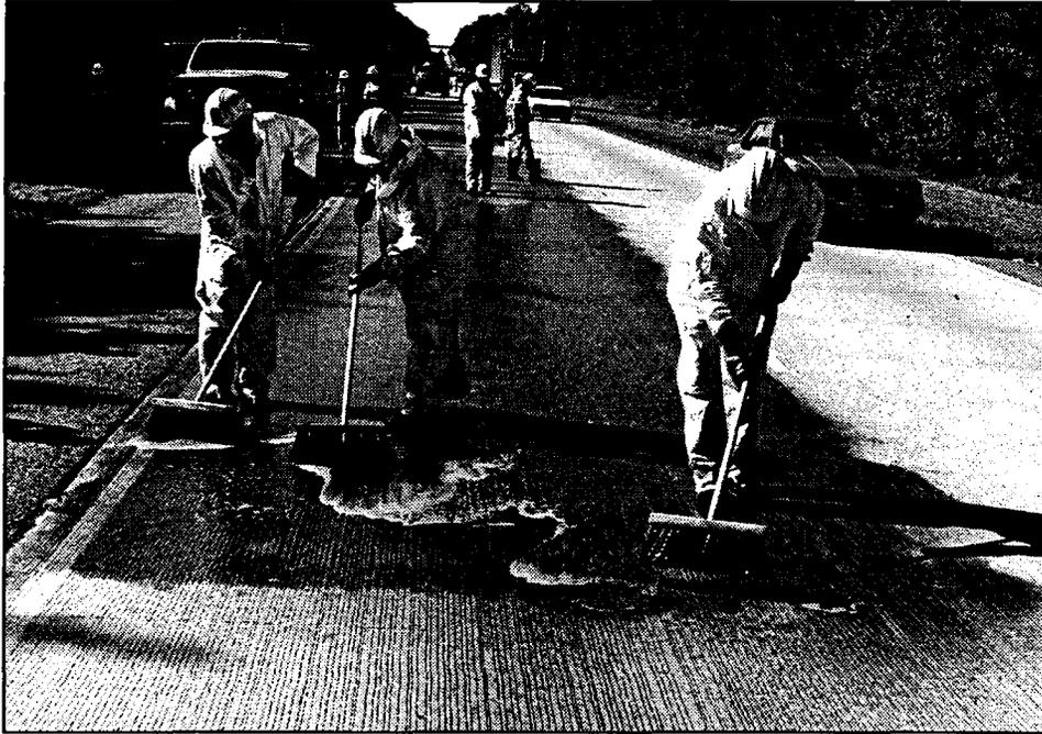
Figure 184. Typically a sealer is applied to a surface with brooms at the recommended application rate.
