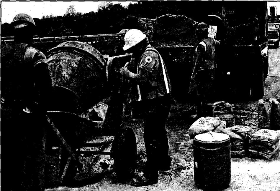
Figure 81. Prepackaged, very rapid hardening hydraulic cement concrete materials are typically used for small Type A and Type B patches. A small concrete mixer can be used to mix the cement, fine and coarse aggregate, and water. Calibrated containers should be used to measure out the required weight of each ingredient.
