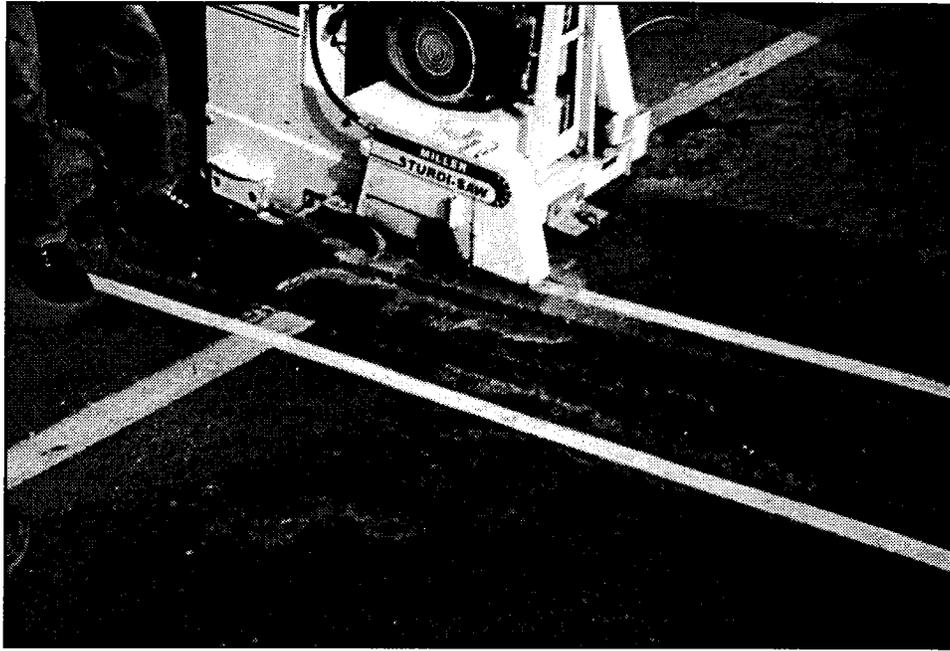
Figure 118. The first step in a joint repair is to sawcut the concrete on both sides of the joint so that the joint and adjacent concrete can be removed.
