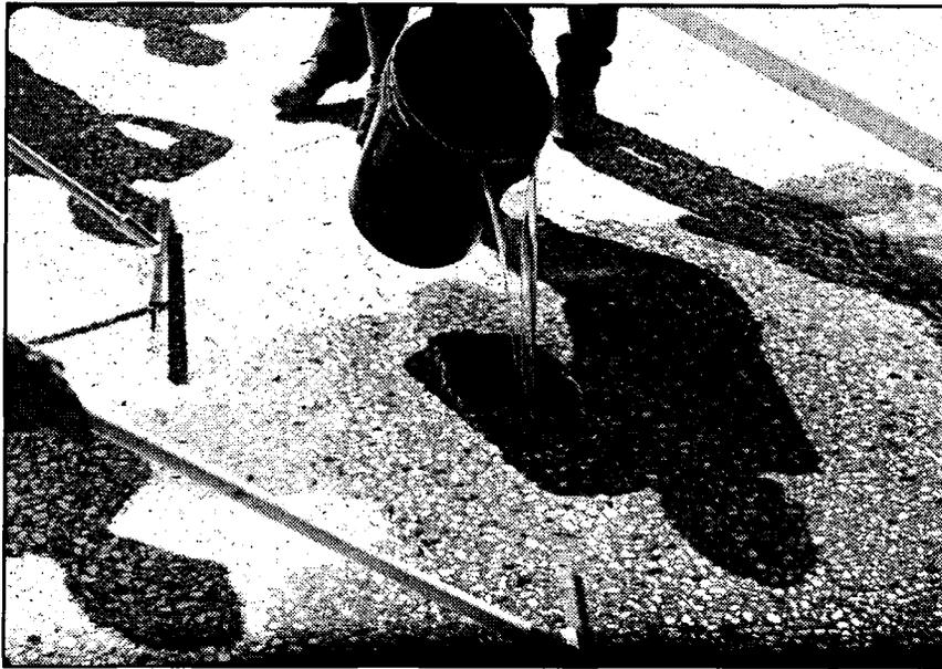
Figure 158. Epoxy should be applied to the deck surface immediately after it is mixed and spread over a premarked area with notched squeegees to insure a uniform application at the specified application rate. Prior to placing the epoxy overlay, or any type of polymer overlay, the surface should be shotblasted to remove oil, carbonation, laitance, weak surface mortar, and other materials that can interfere with the bonding of the overlay (see Figure 146).
