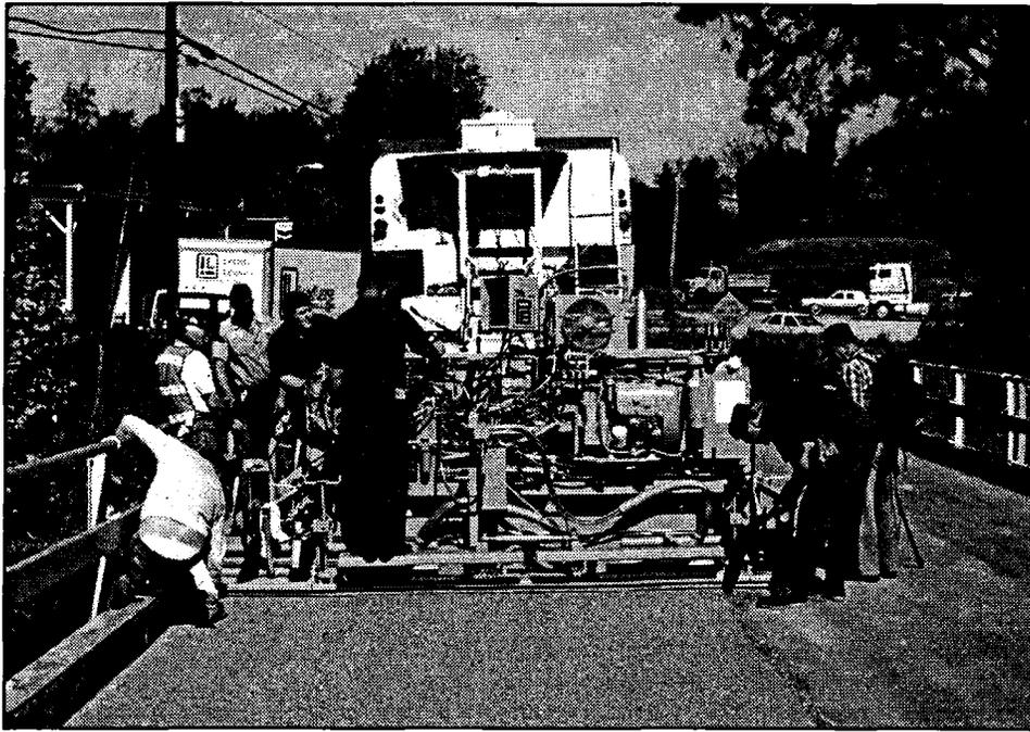
Figure 174. A vibrating slip form paver can be used to apply a premixed polyester styrene concrete overlay to a deck that has received a polyester styrene primer approximately 1 hr earlier. A mobile concrete mixer can supply freshly mixed concrete to the paver.
