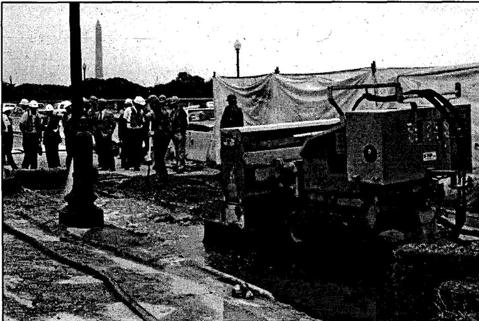
Figure 65. View of the forward end of the hydrodemolition equipment.
