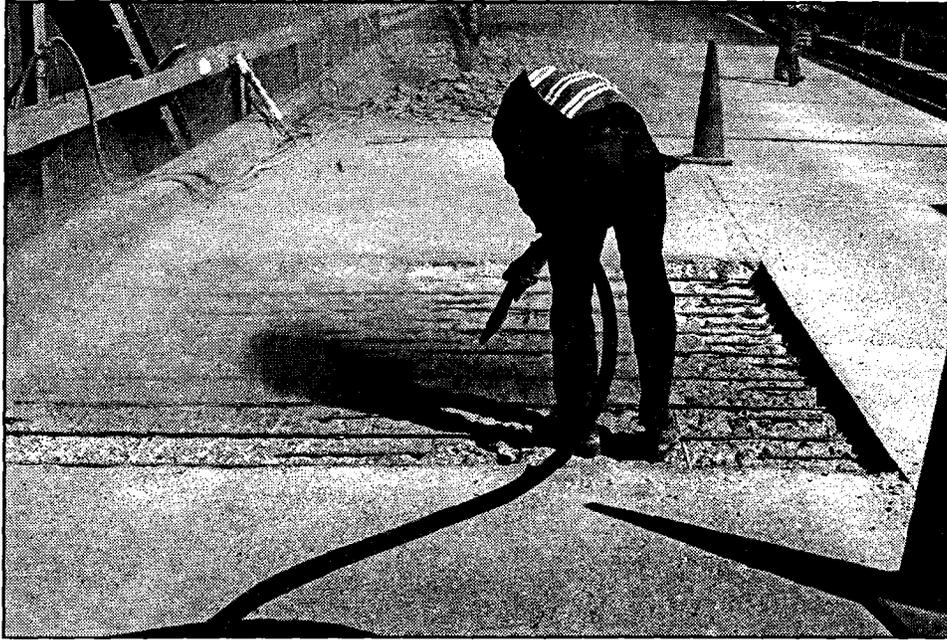
Figure 78. Prior to placing the hydraulic cement concrete patching material, the hardened concrete surfaces and reinforcing steel shall be grit blasted to remove carbonation, laitance, rust and other materials that may be detrimental to the bonding or curing of the fresh concrete.
