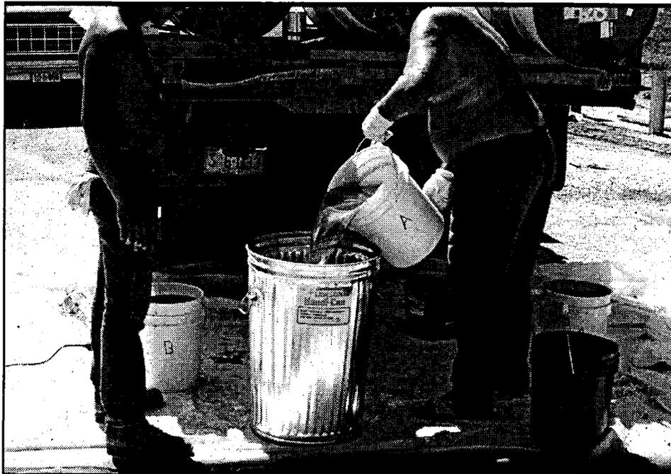
Figure 156. Component A and component B should be added to a mixing container and mixed with a paddle type mixer for several minutes (or as recommended by the manufacturer) to insure complete mixing.
