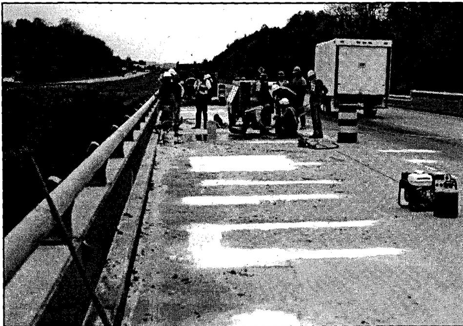
Figure 85. A typical Type B patching operation. When practical, patches should have four sides rather than random shapes.
