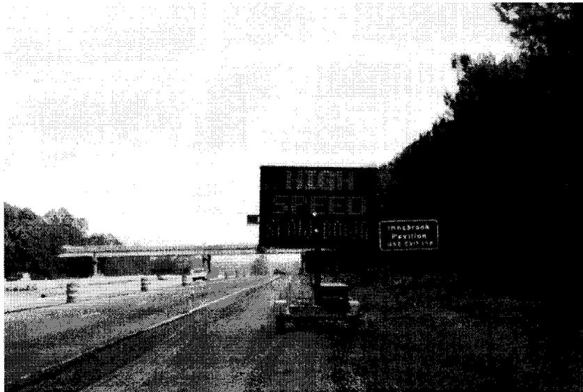
Figure 5. Changeable message sign with radar unit.
