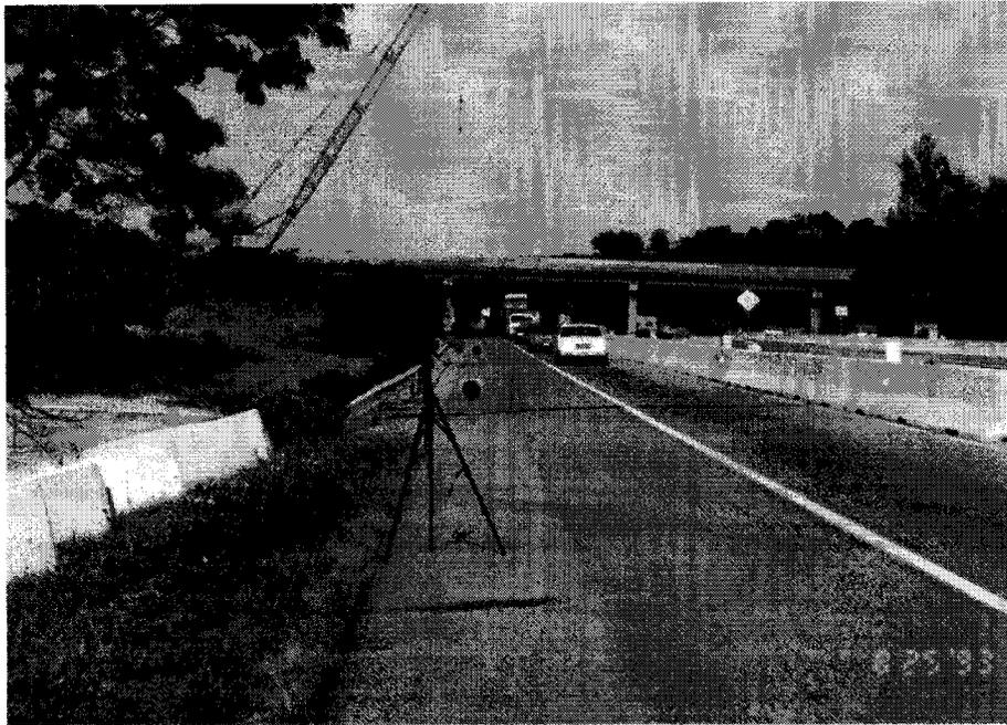
Figure 7. Placement of cameras with respect to 150-foot study area.
