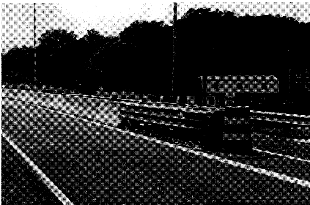
Figure 8. Type 1 attenuator: Guardrail Energy Absorbing Terminal.
