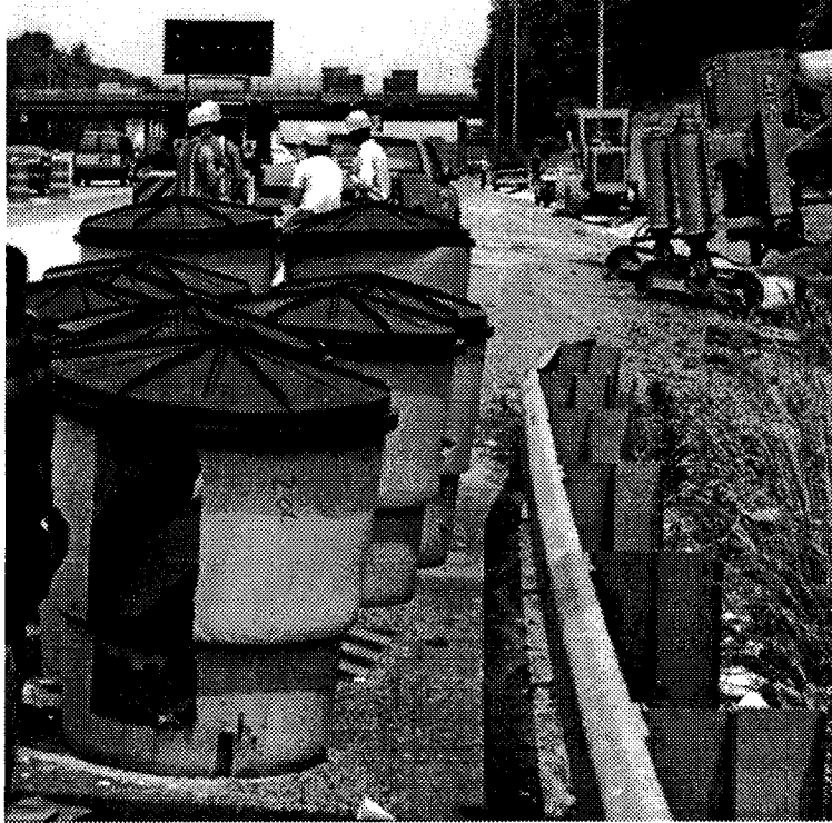
Figure 9. Type 2-11 attenuator: sand barrels.
