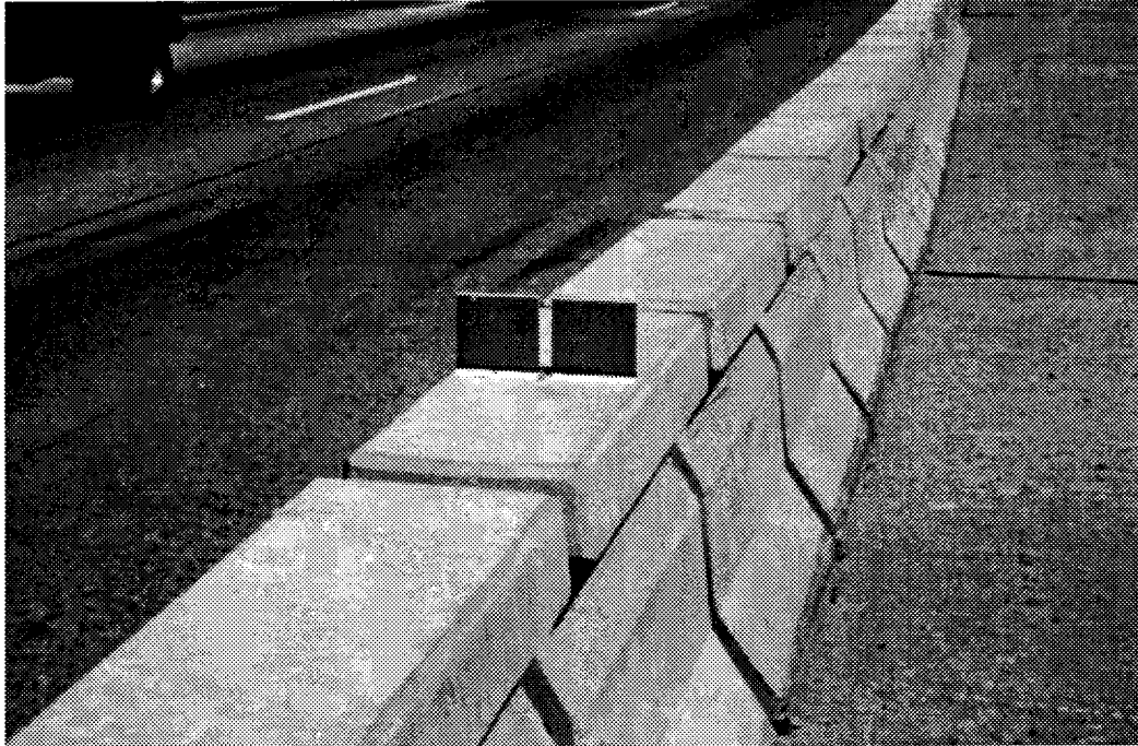
Figure 4. Yellow reflective-sheeting panels mounted on the MCB.
