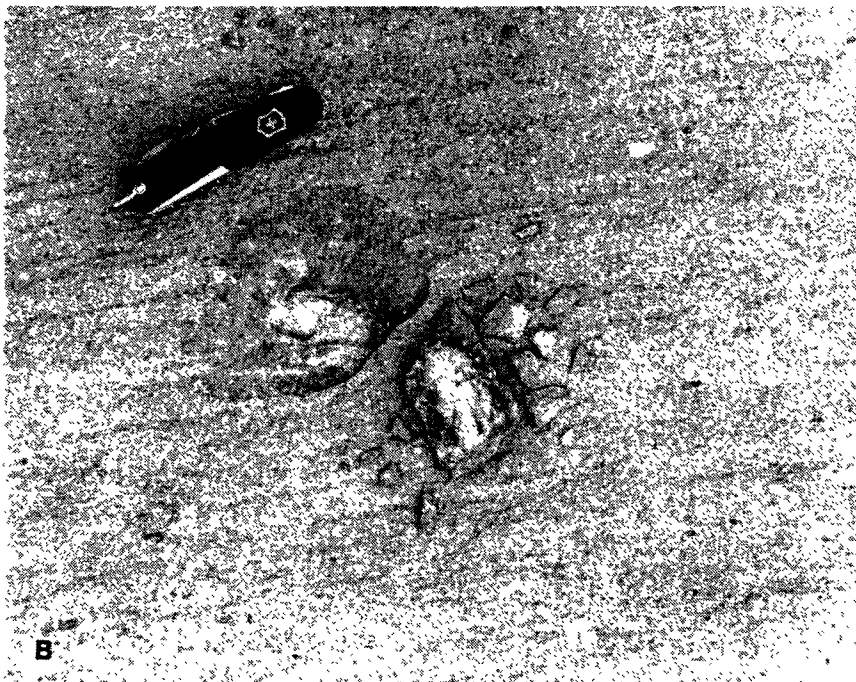
Figure E-1 SHALY PARTICLE SHAPE. A. Particle shape of a crushed slate aggregate. B. Pavement surface with a flaw caused freezing and thawing of water trapped under a particle of the aggregate shown in A.
