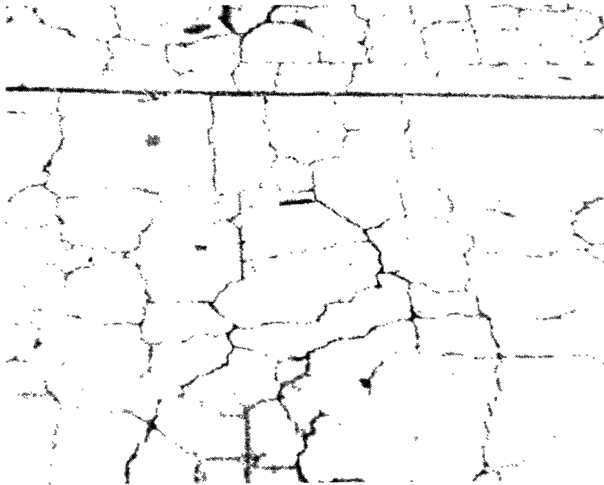
Figure 10-15 DESTRUCTIVE ALKALI-CARBONATE REACTION IN WALKWAY PAVEMENT. In Kingston, Ontario, Canada.
