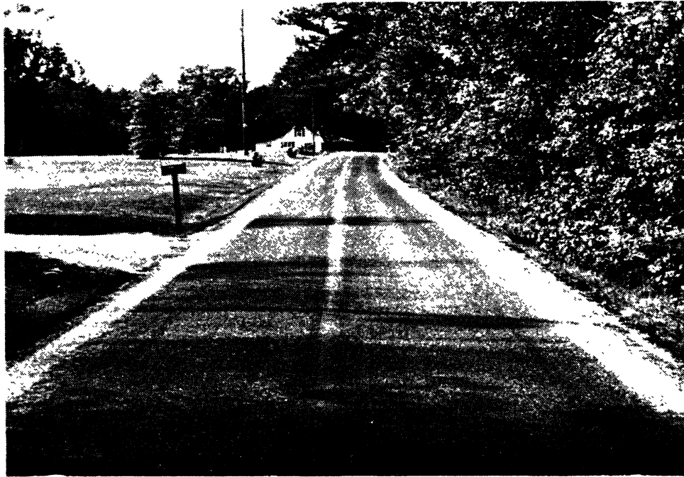
Figure 14. One-month-old modified surface treatment (sand on sides of the road).
