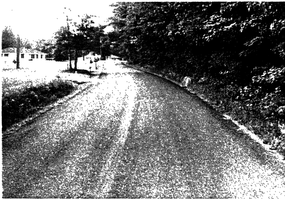
Figure 15. One-year-old modified surface treatment (same road and treatment as in Figure 14).
