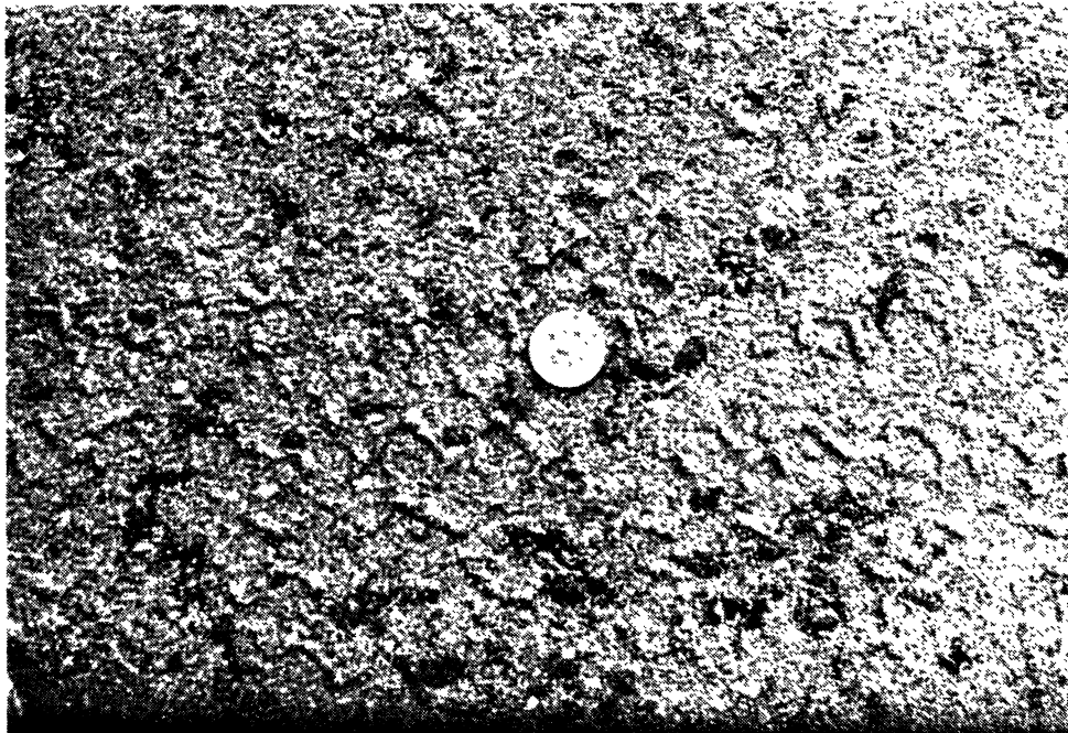
Figure 11. Close-up of modified seal treatment using natural sand for the choke material.
