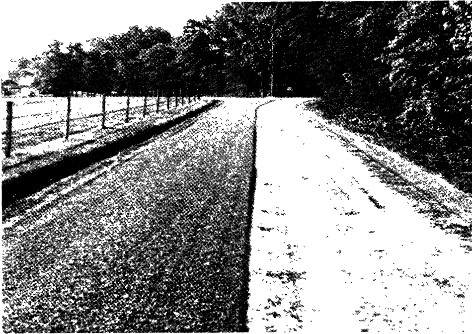
Figure 10. A modified seal treatment under construction (one side has been choked, one side has not).
