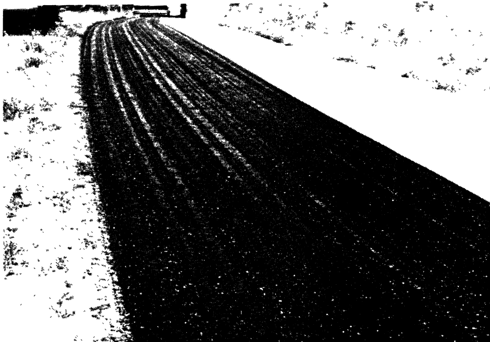
Figure 4. A roadway that is streaked because nozzles of the wrong size were used.
