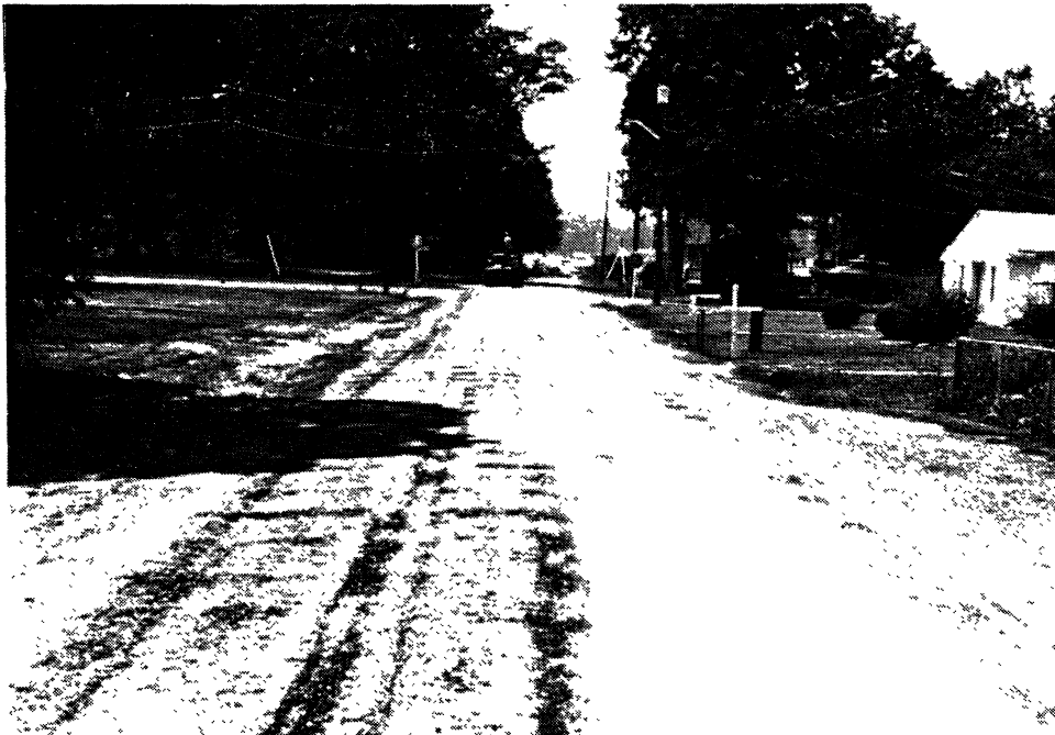
Figure 6. Nonuniform coverage of choke material.
