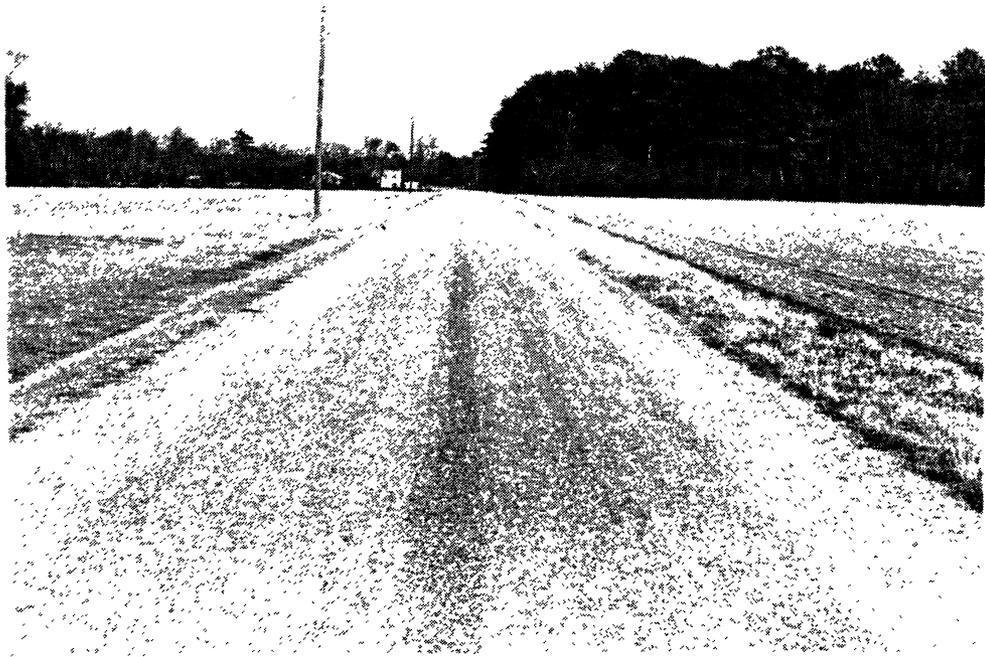
Figure 5. Crushed stone surface treatment performing well.
