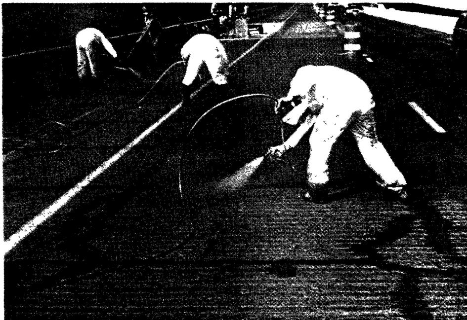
Figure 3. Airless spray guns are used to apply HMWM resin to the surface of the deck on I-81 over the New River in May 1988. Note that the work crew is wearing rubber boots and gloves, impermeable coveralls, and canister breathing masks.
