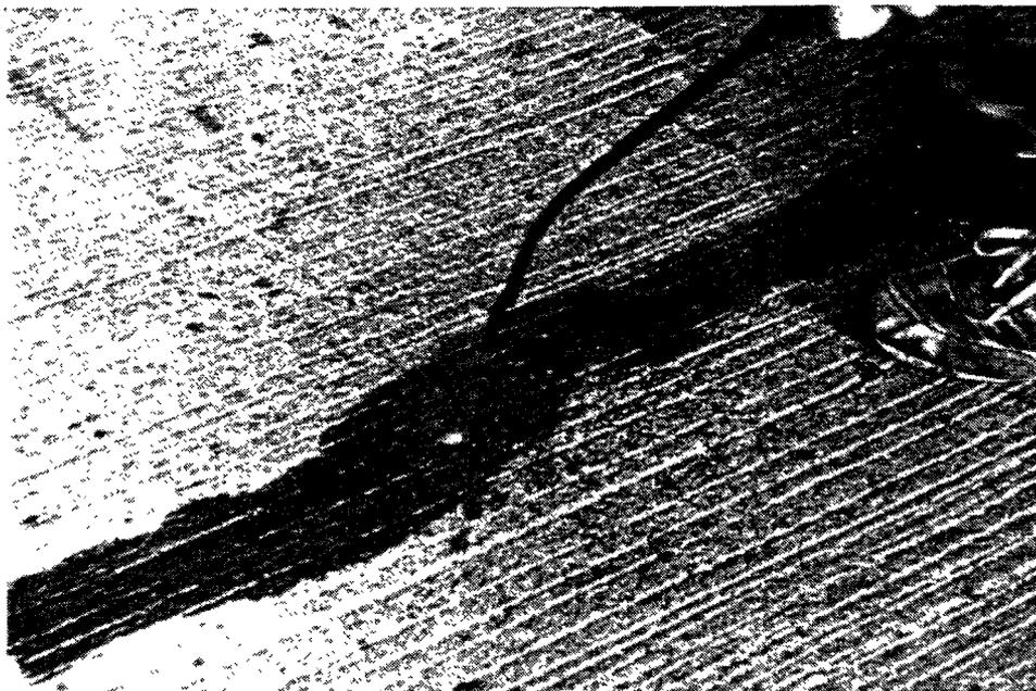
Figure 2. HMWM monomer is applied to cracks in deck on I-81 over the New River. To maintain a good skid number, excess resin in valleys must be broomed over the deck surface before it gels.
