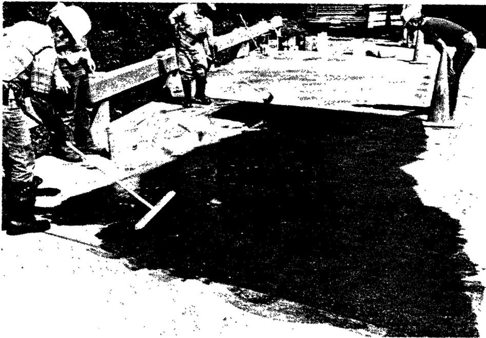
Figure 9. HMWM monomer is applied to the deck surface (no tined texture) to fill cracks. Sand is broadcast into the monomer to provide adequate skid resistance (Rte. 601 over Polecat Creek, Caroline County, June 1986).
