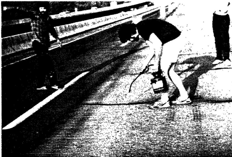
Figure 1. HMWM monomer is applied to cracks in deck on I-81 over the New River in May 1988.
