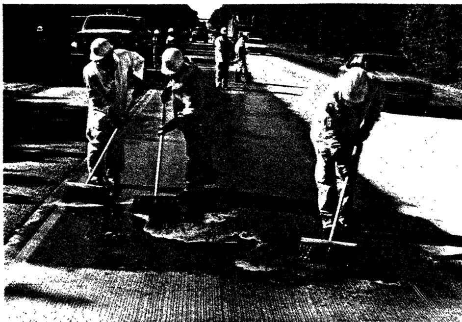
Figure 11. HMWM monomer is applied to pavement on I-64 in New Kent County in October 1989 to reduce spalling caused by alkali-silica reaction.
