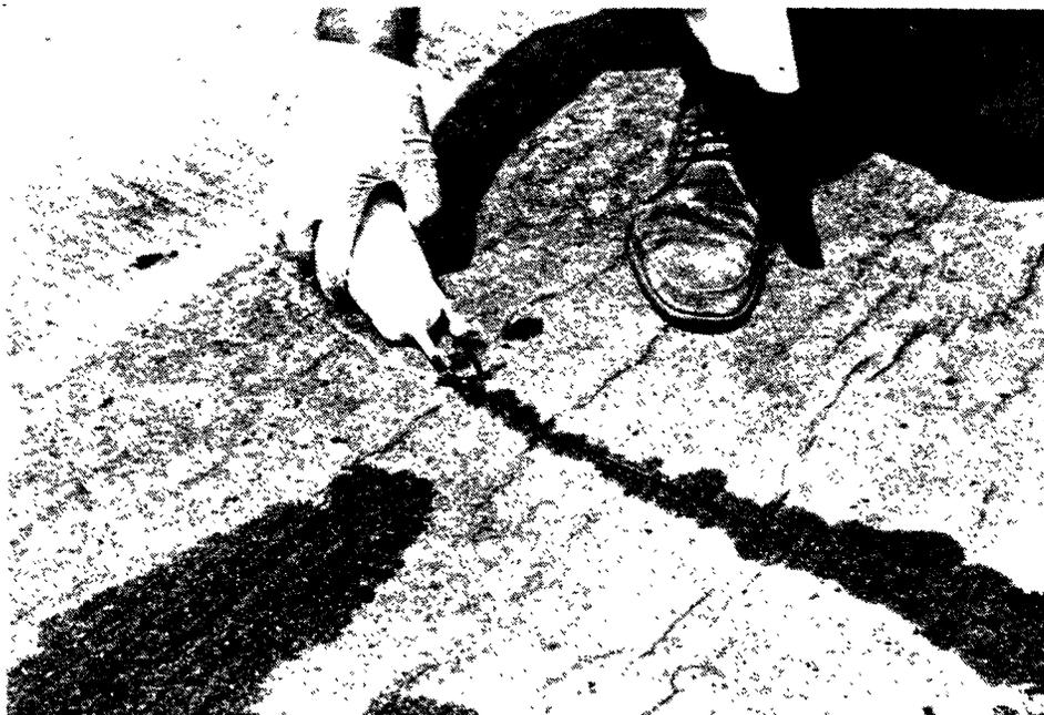
Figure 10. A squeeze bottle is used to apply HMWM monomer to a crack on I-64 in Louisa County in June 1986.
