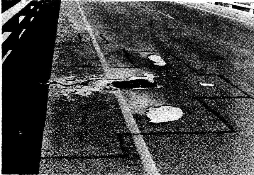
Figure 9. The area over which the concrete is to be removed should be "squared up" and marked with paint.
