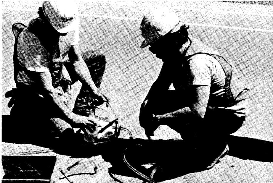
Figure 16. Vacuum injection can be used to fill cracks with a methacrylate resin. Prior to introducing the resin, steel entry ports should be placed on the crack surface, the cracks are covered above and below with a viscous paste-like epoxy, and a vacuum is applied to the cracks through the ports. The requirements for successful filling of a crack cited under Figure 12 (pg 2-7) are also generally applicable to vacuum injection.
