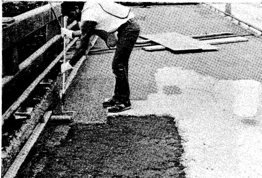
Figure 32. Polyurethane primer can be applied with roller approximately 1 hour prior to placing a premixed polyester amide para resin concrete overlay. The primer must cure prior to the placement of the overlay.
