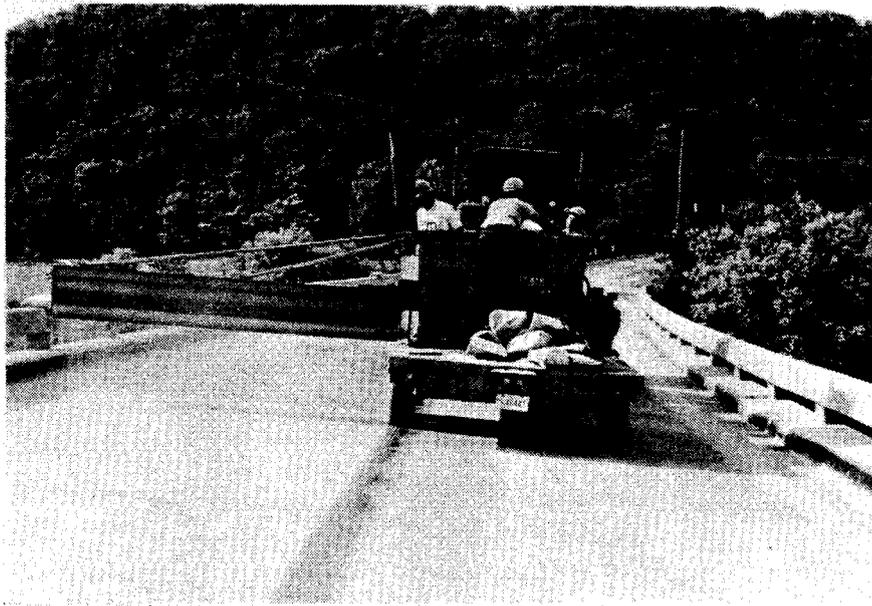
Figure 22. Aggregate can be applied to excess using a wing spreader.
