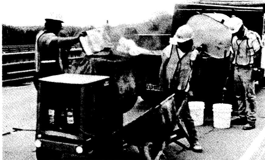
Figure 6. Prepackaged rapid hardening cementitious materials are usually used for Type A, Type B, and small Type C patches. A mortar mixer (shown here) may be used if coarse aggregate is not used to extend the mixture. The rapid-hardening materials are very sensitive to the quantity of water used. The calibrated containers shown here should be used to measure out the required weight of water.
