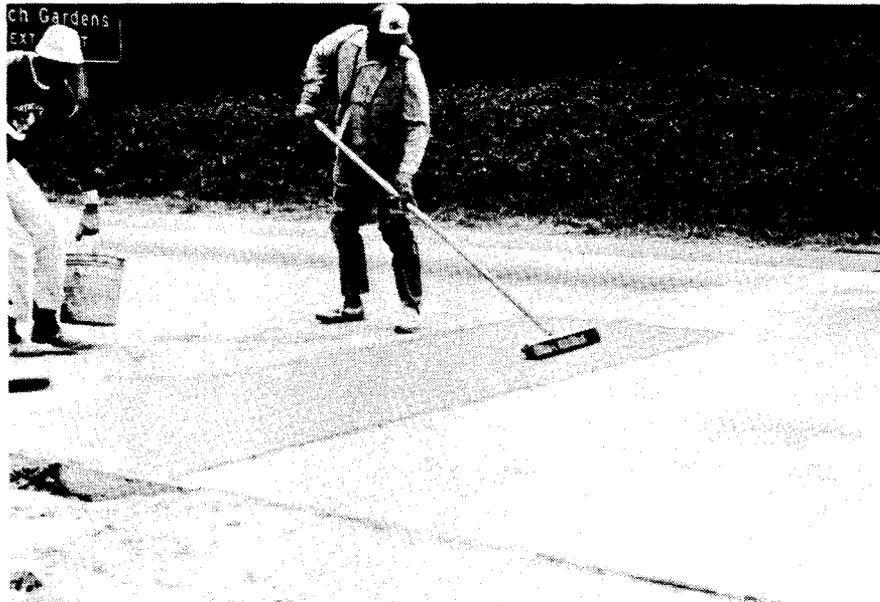
Figure 5. The ready-mix concrete should be consolidated with internal vibrators, struck off, textured with a broom as shown here (other textures may be specified) and covered with burlap and polyethylene or liquid membrane curing material. When the patches must be opened to traffic in much less than 24 hrs, the ready-mix concrete is usually made with Type III cement and accelerating admixtures or special high early strength blended cements.
