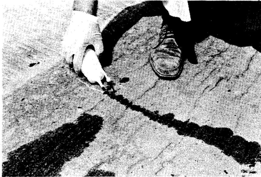
Figure 12. High molecular weight methacrylate can be applied to a crack. For satisfactory filling of the crack, it should be free of debris and wider than 0.1 mm. Also, best results can be obtained by filling cracks when they are open the widest at the surface (temperatures between 55°F and 70°F and between 1:00 a.m. and 10:00 a.m). High molecular weight methacrylate will not cure satisfactorily at temperatures below 55°F.
