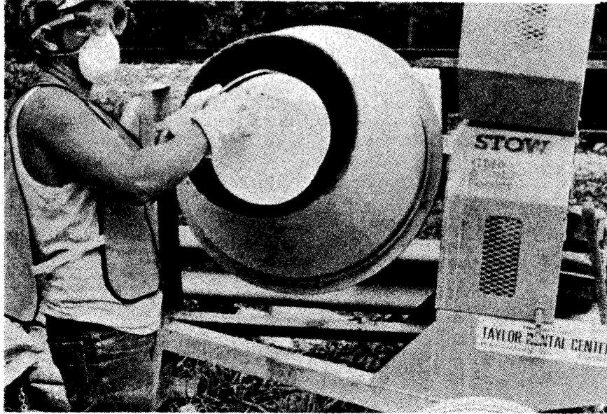
Figure 33. Polyester amide para resin is here added to the concrete mixer.
