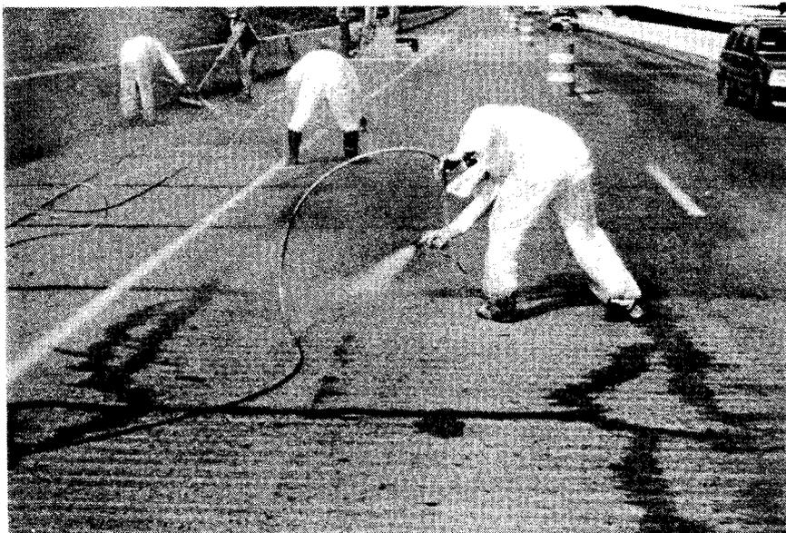
Figure 50. High molecular weight methacrylate coating can be applied with an airless sprayer. Note that the spray gun operators are wearing impermeable boots, gloves, and coveralls and canister masks.
