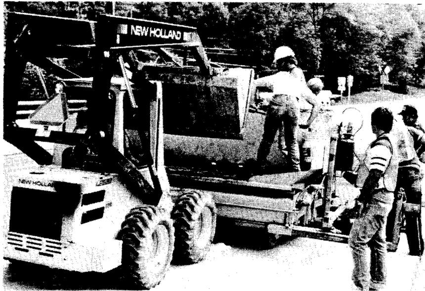
Figure 39. A front-end loader can be used to fill the slip form paver with premixed conductive polyester styrene resin concrete for conductive polymer overlay.
