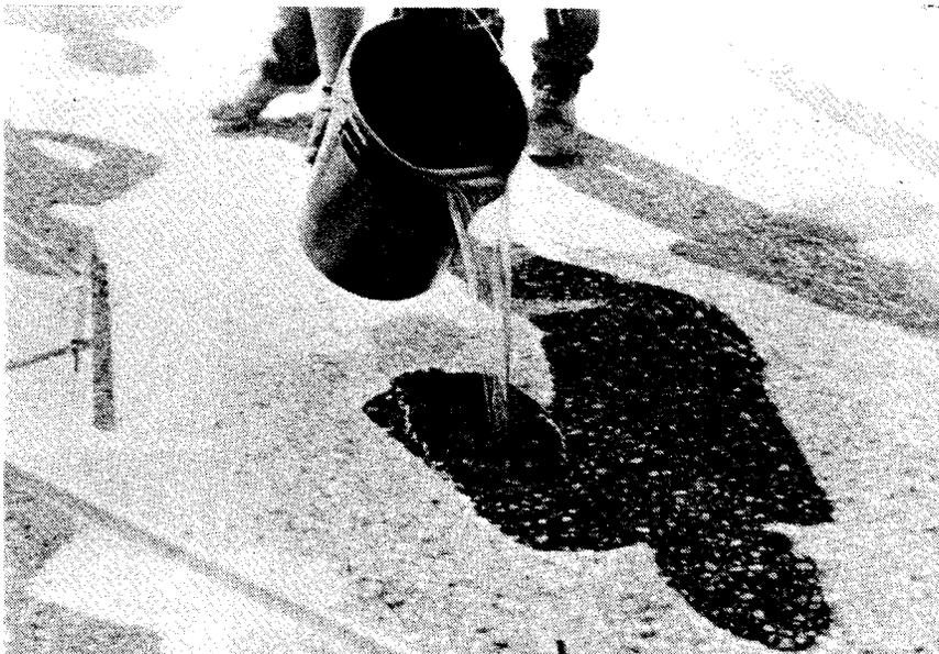
Figure 16. Epoxy should be applied to the deck surface immediately after it is mixed and spread over a premarked area with notched squeegees to insure a uniform application at the specified application rate. Prior to placing the epoxy overlay, or any type of polymer overlay, the surface should be shotblasted to remove oil, carbonation, laitance, weak surface mortar, and other materials that can interfere with the bonding of the overlay (see Figure 15, pg. 1-8).
