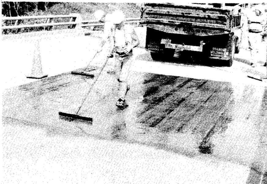
Figure 17. An epoxy urethane mixture is here spread over the deck with notched squeeeges. Basalt aggregate is here broadcast to excess from the back of a dump truck.
