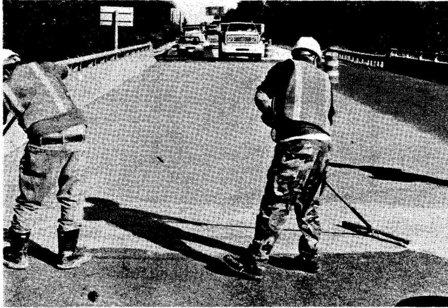
Figure 29. A methyl methacrylate slurry overlay should be struck off with gage rakes set to provide a  $\frac{3}{16}$  in thick layer of slurry.
