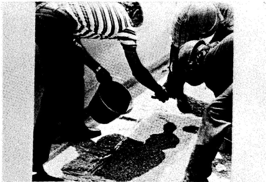
Figure 22. Aggregate should be broadcast onto resin.
