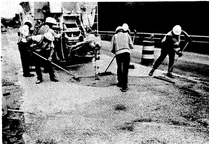
Figure 11. A latex modified slag slurry overlay may be applied to a bridge deck to increase the skid resistance. Brooms should be used to brush the slurry into the shotblasted surface.
