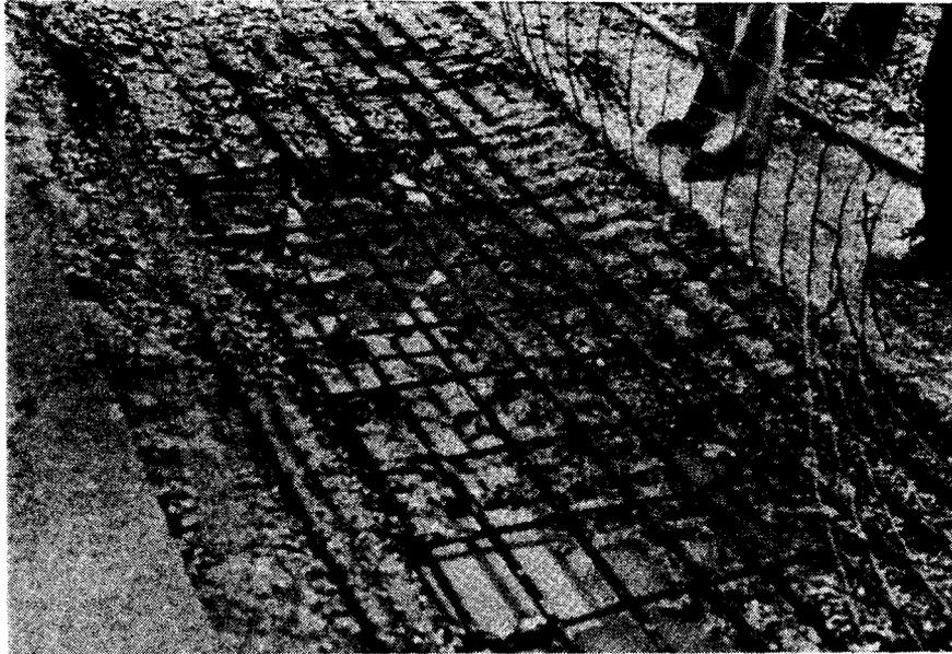
Figure 19. Concrete can be dislodged and reinforcement can be cleaned by hydro demolition. The dislodged concrete and water must be removed from the surface prior to placing the overlay or repair material. Vacuums, shovels, and air blasting have been used to remove contaminants. Proper containment and disposal of blast water and concrete rubble is necessary.
