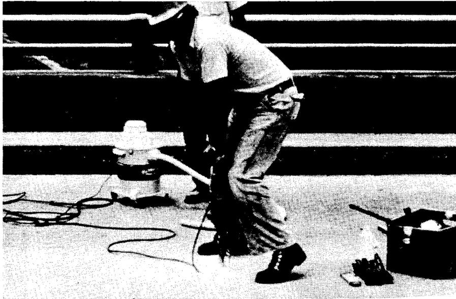
Figure 7. Chloride content measurements can be made on samples of pulverized concrete taken in the vicinity of the reinforcement. A pacometer can be used to locate and to provide an indication of the depth of cover over the reinforcement. A drill should be used to remove the concrete above the sample down to within approximately 1/2 in. of the reinforcement. A vacuum can be used to remove concrete from the drill hole.
