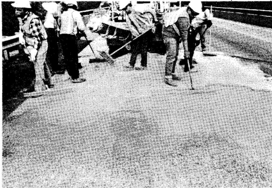
Figure 12. The latex modified slag slurry should be struck off and pulled forward with gage rakes set to provide a  $3/16$  in to  $1/4$  in thick slurry. For increased skid resistance slag should be broadcast onto the struck off surface. The slurry should be protected from drying by prompt application of wet<sub>2</sub> burlap and polyethylene when the evaporation rate exceeds  $0.05 \text{ lb/ft}^2/\text{hr}$ .
