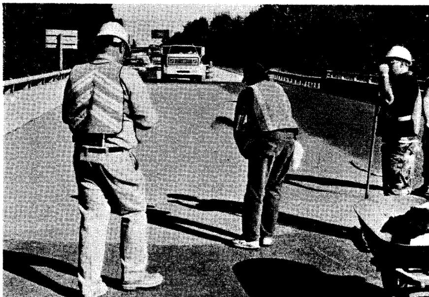
Figure 30. Aggregate should be broadcast to excess onto the slurry within 5 minutes after the slurry is placed.
