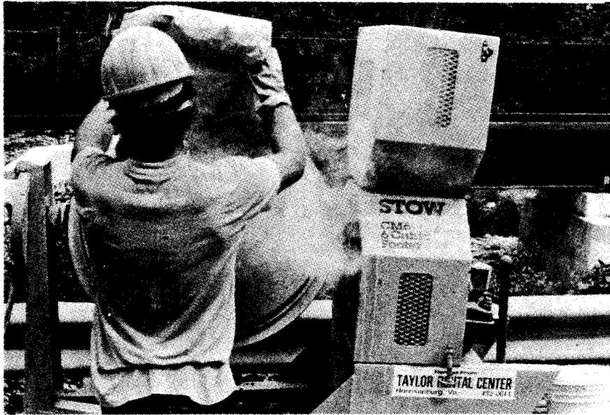
Figure 35. Prepackaged aggregate is here added to concrete mixer.
