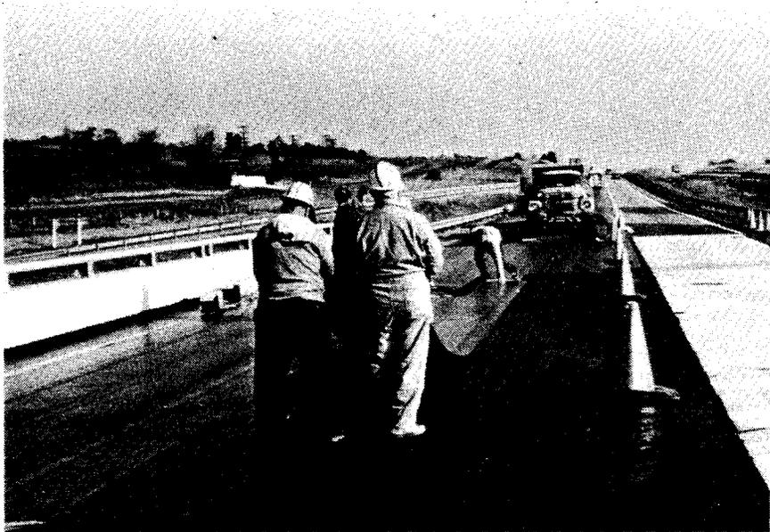
Figure 44. A prefabricated membrane should be placed on the primer. Care must be exercised to lap the joints to minimize wrinkles in the membrane and to eliminate air pockets under the membrane.
