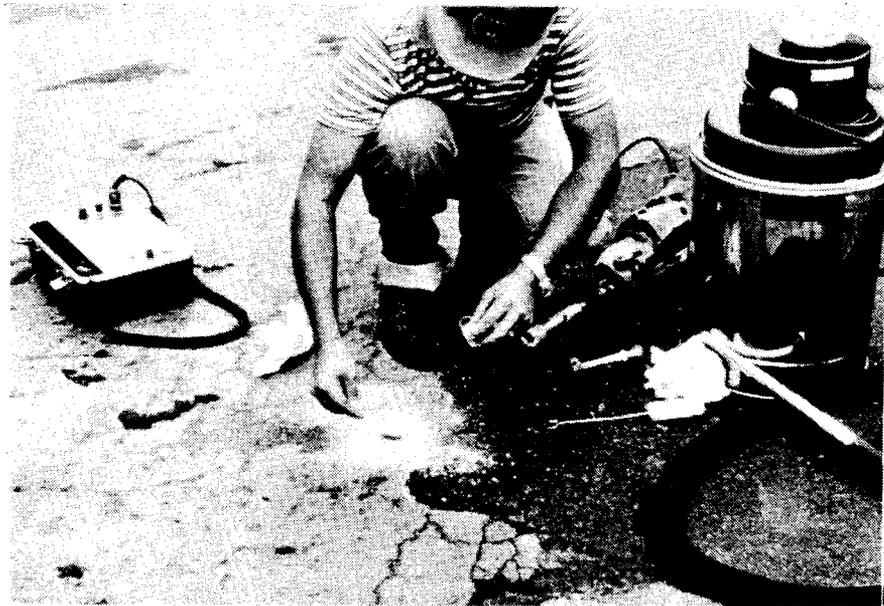
Figure 8. The drill should be returned to the hole, and the sample in the vicinity of the reinforcement should be pulverized. A spoon can be used to collect the sample. A chloride content  $\geq 2$  lb/yd<sup>3</sup> can cause corrosion.
