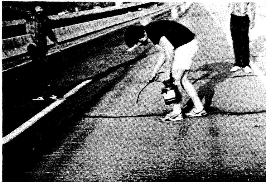
Figure 13. A pressurized spray can be used to apply high molecular weight methacrylate resin to a crack. For best results, a brush should be used to work the resin into the crack.
