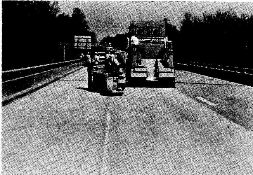
Figure 15. Shotblast equipment is available in a range of sizes. Units that blast a 9-in-wide strip and a 6-ft-wide strip are shown above.
