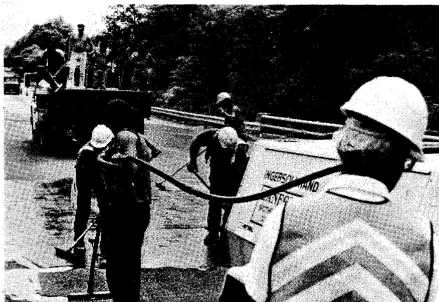
Figure 24. An epoxy urethane binder that has been blended with positive displacement pumps and mixed with an in-line static mixer is here deposited onto the surface with a wand. Squeegee can be used to spread the resin over the required area and aggregate can be broadcast to excess with shovels from the back of a dump truck.
