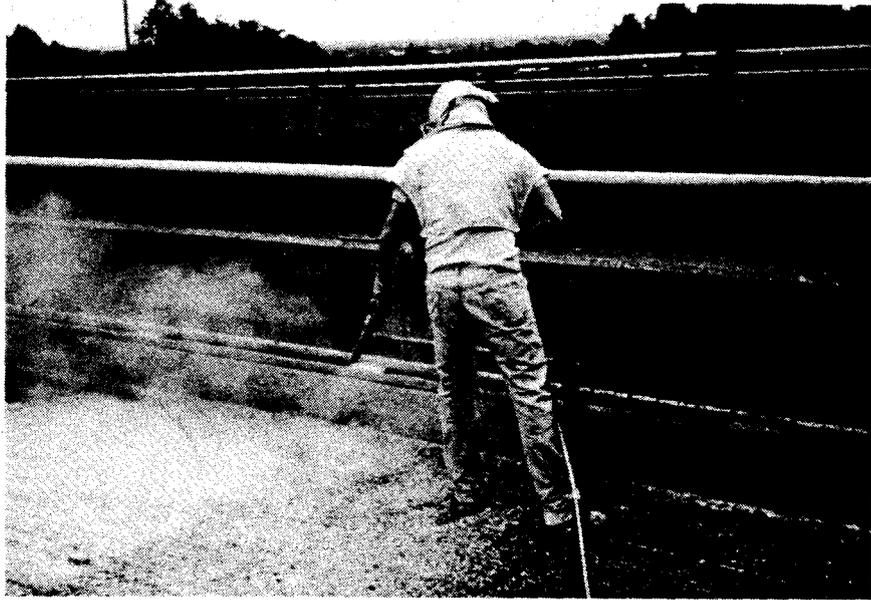
Figure 13. Sandblasting (typically with slag rather than sand) can be used to remove carbonation, laitance, weak surface mortar, and other materials that may be detrimental to the bonding of the overlay or to the repair material.
