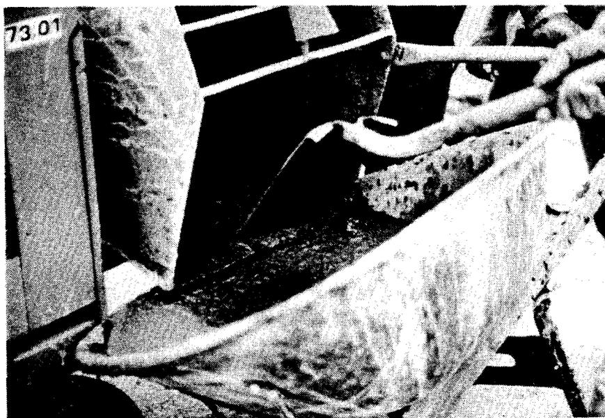
Figure 7. A wheelbarrow is usually used to transport mixed ingredients a short distance to the patch site.
