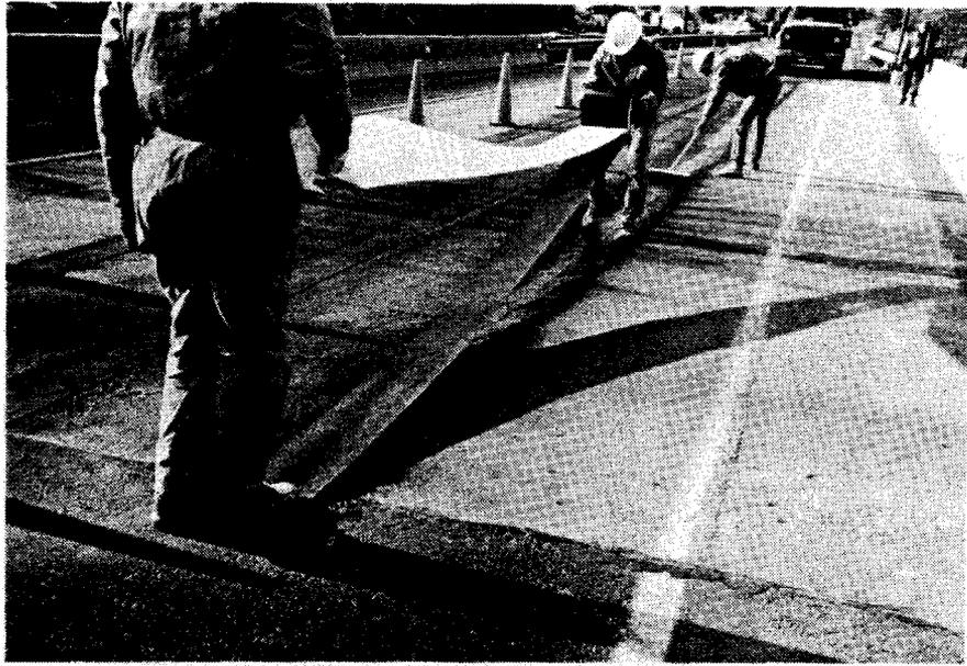
Figure 47. A 12-in wide sheet membrane can be placed on the primer to protect the keyways between precast concrete slabs. The entire deck surface should be covered with a tac coat and a bituminous concrete overlay.
