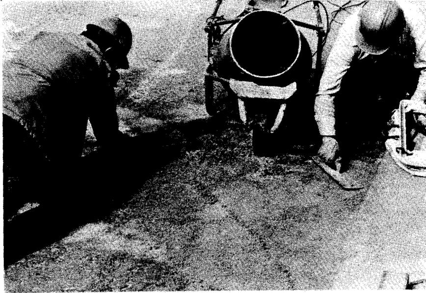
Figure 3. Type D patches (epoxy mortar) are used for shallow repairs ( $\leq 3/4$  in deep). Areas to be patched shall be dry and shall be primed with neat epoxy prior to placing the mortar.
