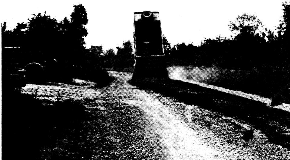
Figure 11. Tailgate spreading of slate with slight necking of the distribution pattern at arrows.
