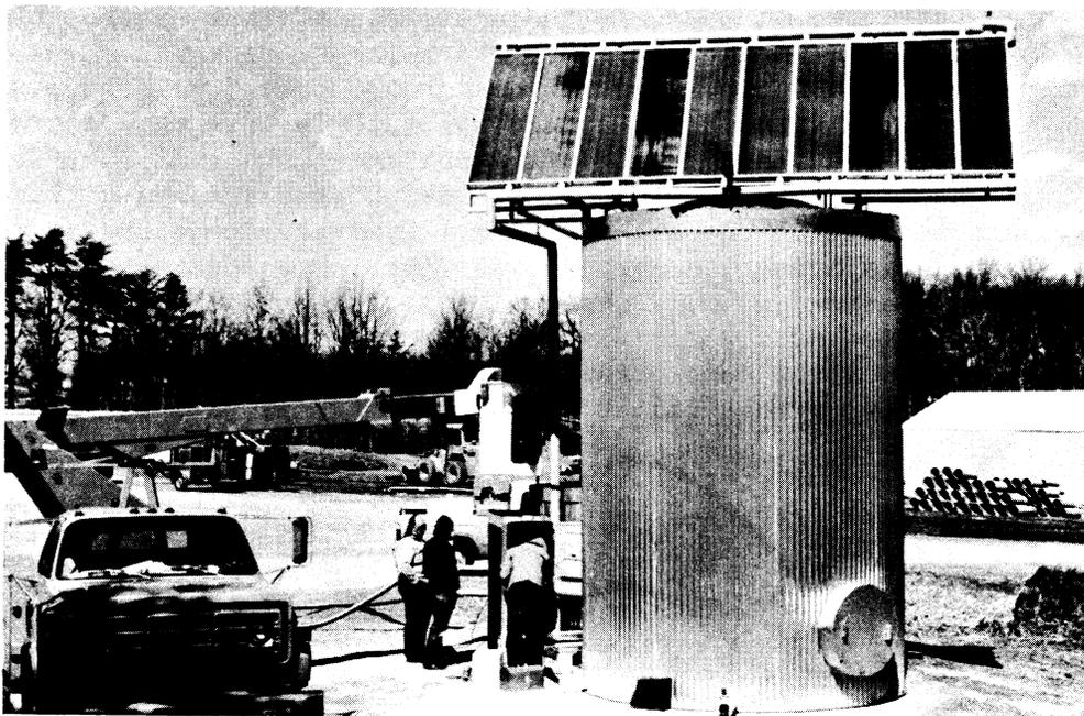
Figure 2. View of completed solar heated asphalt storage tank.
