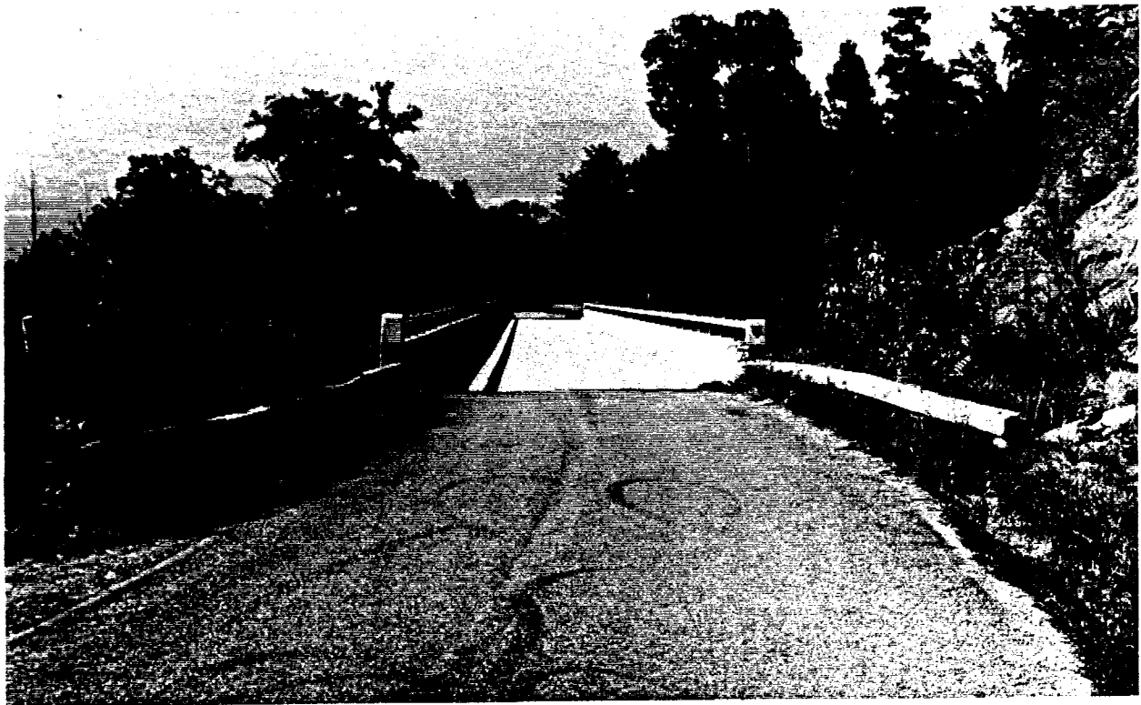
Figure 10. Low-volume service road bridge provides access to residence and orchard.
