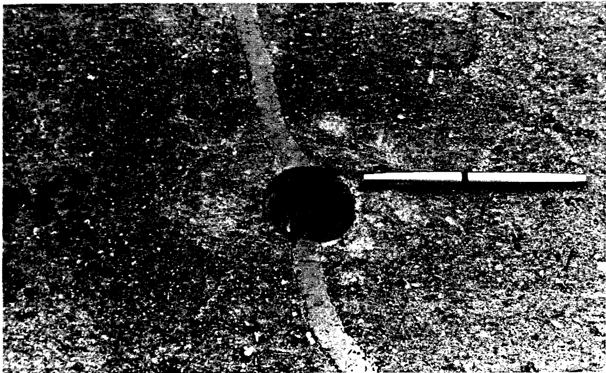
Figure 12. Cracks routed to a depth of 1/2 in and sealed.
