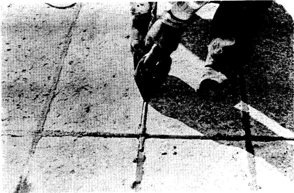
Figure 6. Filling slots with conductive polymer concrete.
