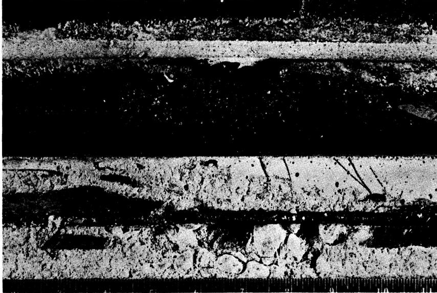
Figure 7. Deterioration at beam/sealant interface.
