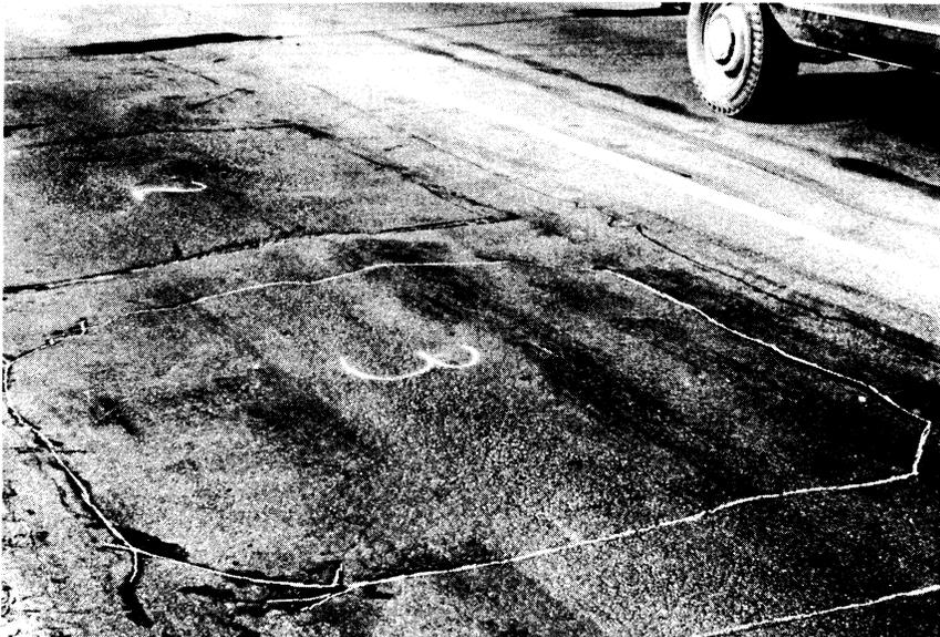
Figure 1. Loop distortion at site of Demonstration #1.
