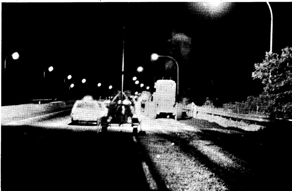
Figure 15. Auxiliary lighting for night operations in New York.
