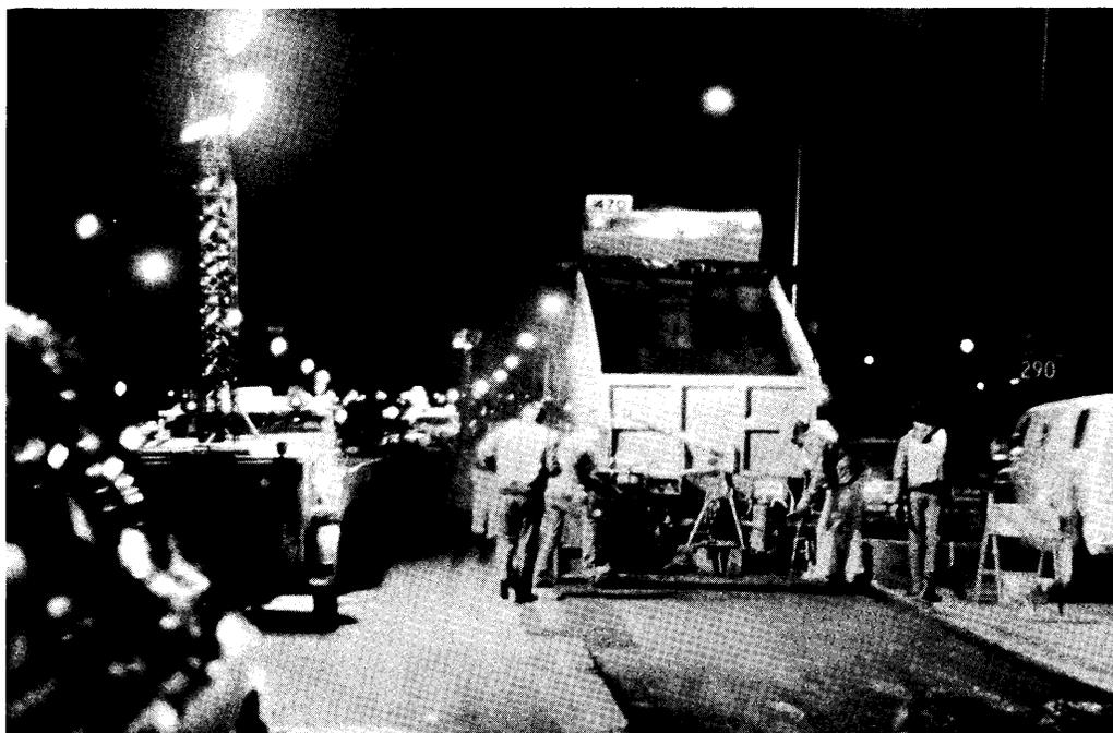
Figure 14. Auxiliary lighting for night operations in Chicago.
