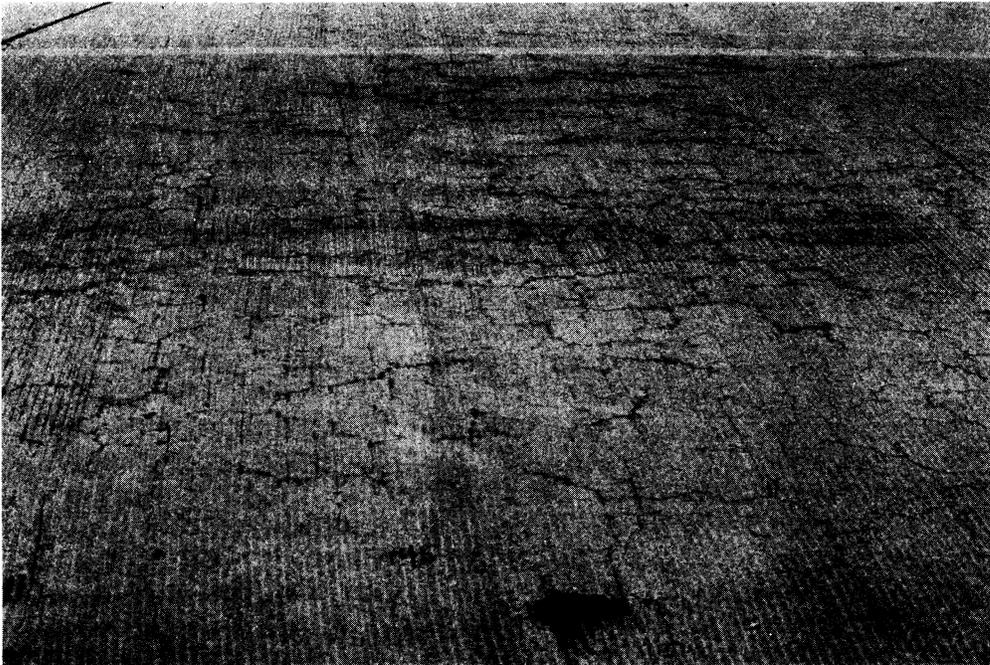
Figure 7. Plastic shrinkage cracks in LMC overlay.
