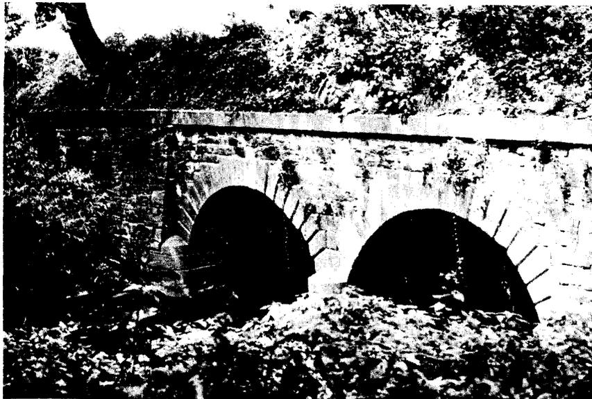
Figure 22. This two-span stone masonry bridge originally carried the James River and Kanawha Canal over Owens Creek. It is located in Nelson County and now carries Rte. 606 over the creek.
