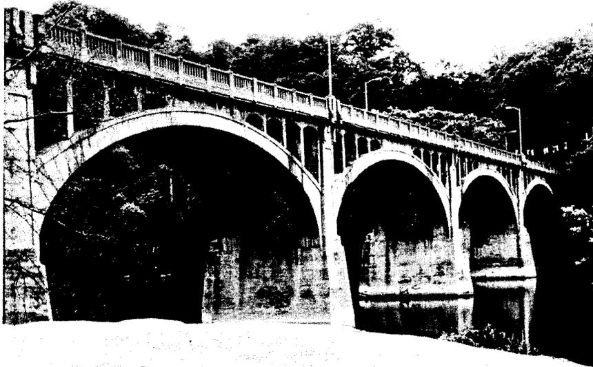
Figure 30. The Memorial Avenue Bridge in Roanoke was built in 1926. This ornamented, monumental metropolitan highway bridge is constructed with three heavy arch ribs.
