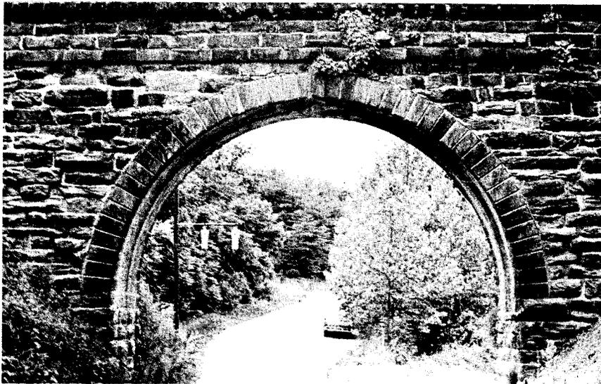
Figure 17. This large circular stone arch, located in Campbell County, was probably built by the Southside Railroad, later part of the N & W system.
