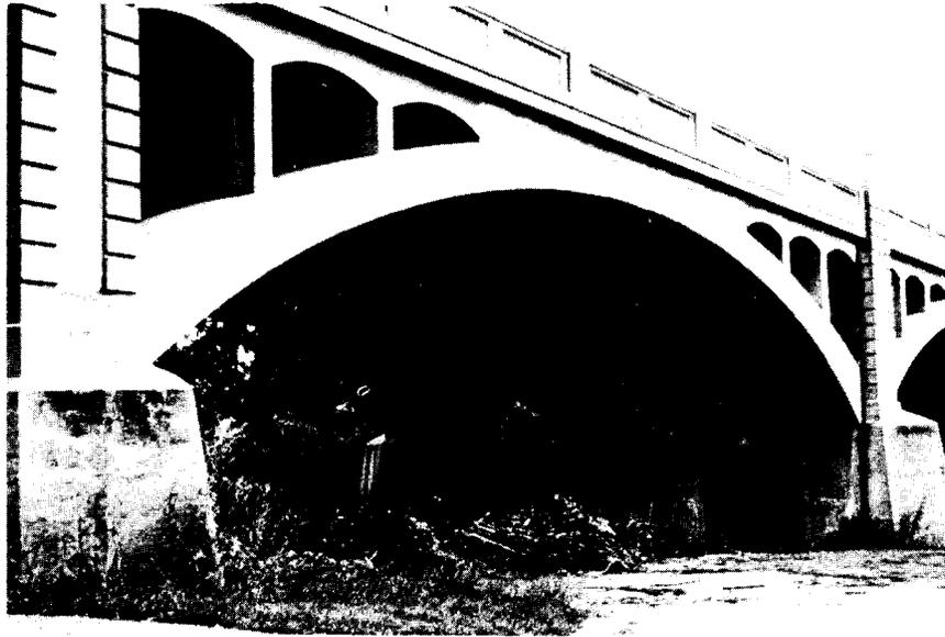
Figure 26. This open spandrel arch bridge was built in Lynchburg between 1916 and 1918. It carries Rte. 29 across the James River.
