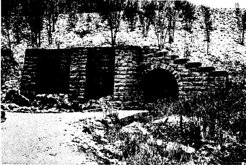
Figure 12. This asymmetrical, massively buttressed railroad underpass was built at Honaker by the N & W Railroad between 1887 and 1889 on its Clinch River Extension, which tapped rich coal fields.
