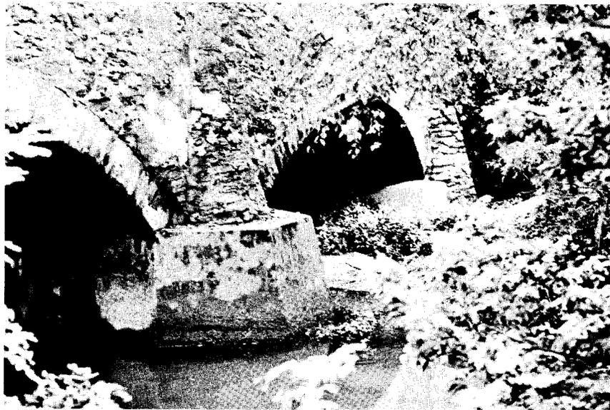
Figure 4. Two-span stone arch bridge on the nineteenth century Snicker's Gap Turnpike corresponds to the construction types in Figures 2 and 3, and could have been built by the same mason.
