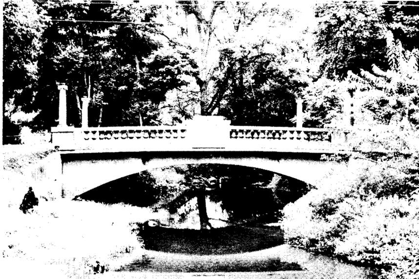
Figure 24. The single-span barrel arch with decorative elements added constitutes Luten's "park bridge." This Luten bridge is located in Bland, Virginia.
