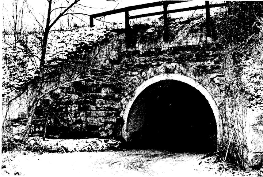
Figure 19. This stone underpass was built by the N & W Railroad in Giles County. It was later widened and modified with concrete. Note the concrete lining inside the barrel.
