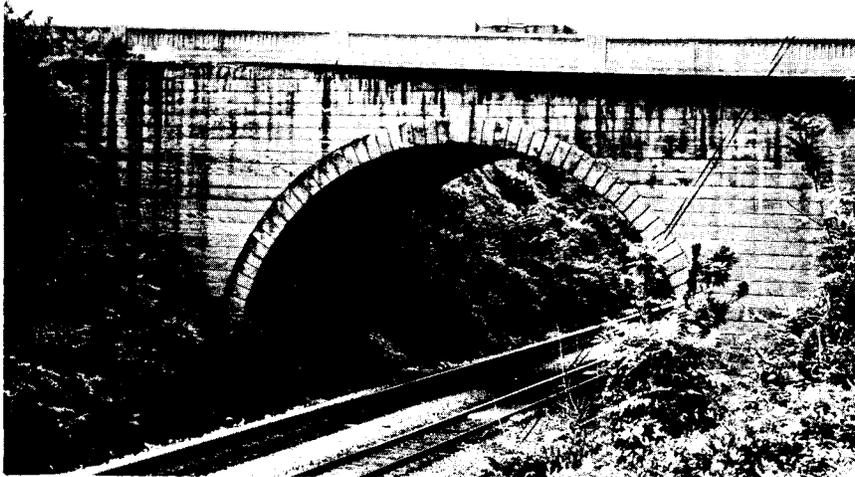
Figure 27. Concrete arch bridge built in Bedford in 1907. The surface was treated to roughly imitate stone.
