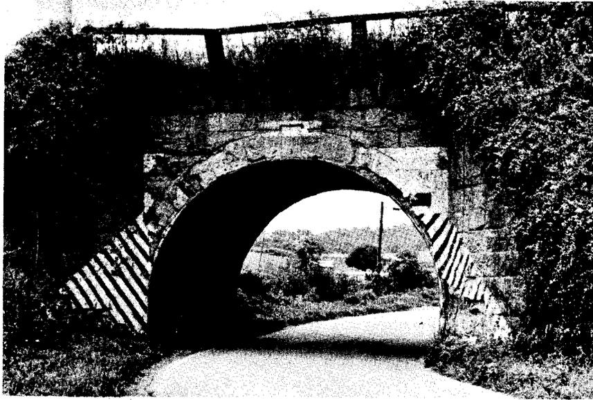
Figure 16. The keystone carving of 1901 on this N & W Railroad underpass dates this arch to an era of very late solid masonry construction.
