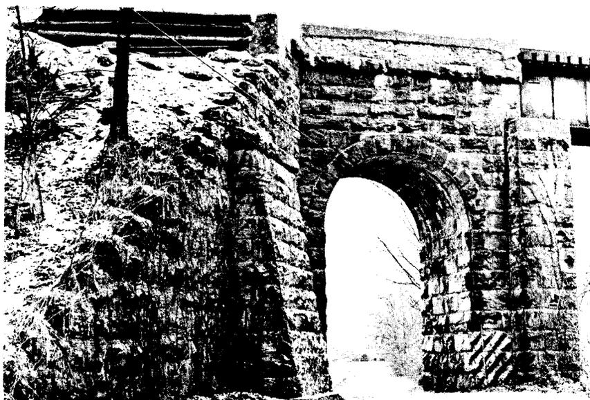
Figure 15. This Roman arch was constructed in 1896 in Smyth County. The arch acts as an underpass for this bridge which carries the N & W Railroad across the Holston River.
