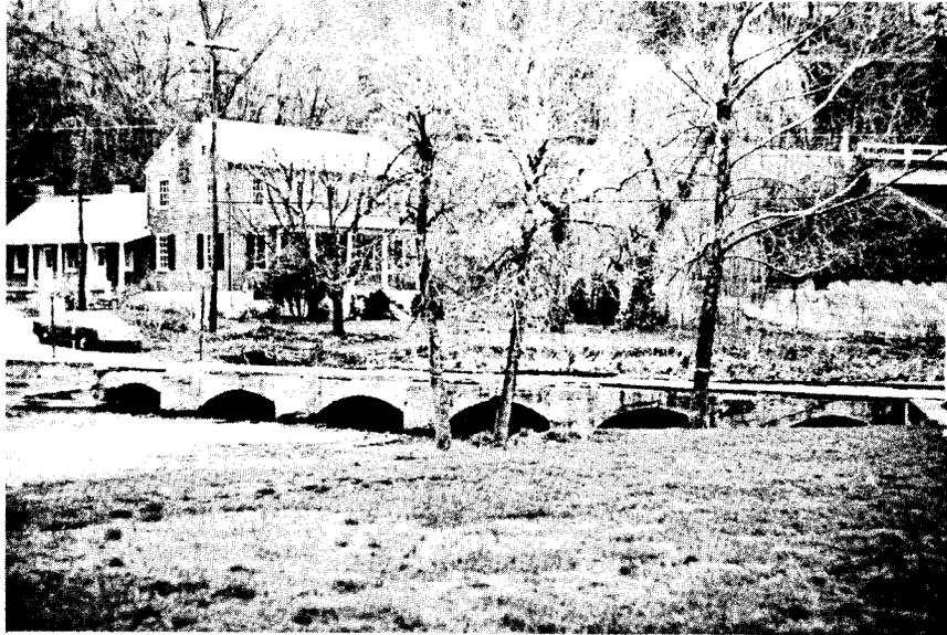
Figure 32. Regional diversity also is illustrated by a series of low multiple arches built in Shenandoah County.
