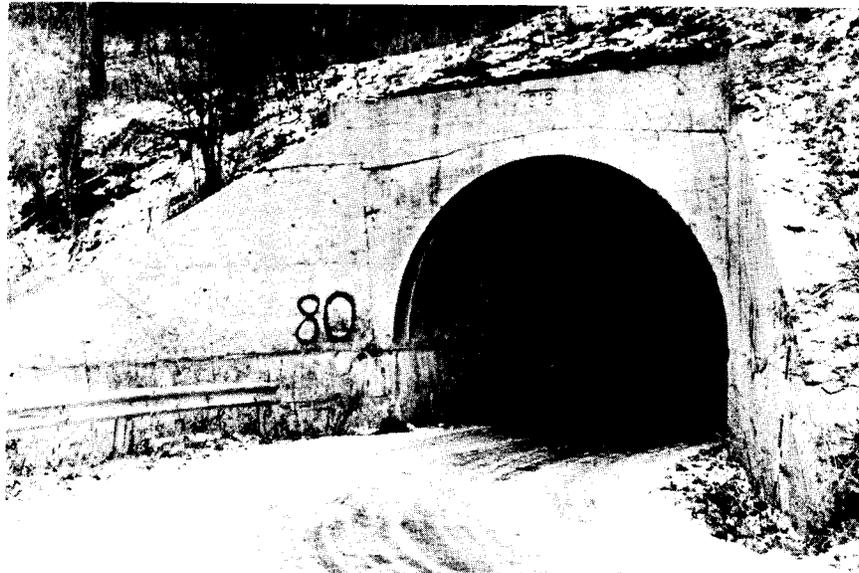
Figure 20. The stone arch in Figure 19 is completely encased in concrete on its opposite approach. It appears to be a concrete structure from this side.
