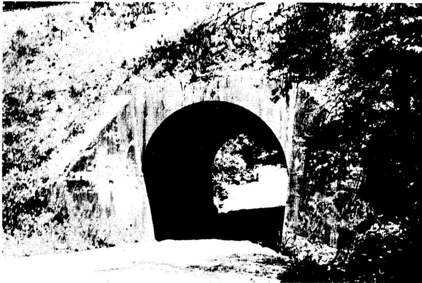
Figure 31. Concrete arch underpass, constructed in Montgomery County, illustrates the regional diversity found in Virginia arch types. This "horseshoe arch" was built only in Montgomery County.
