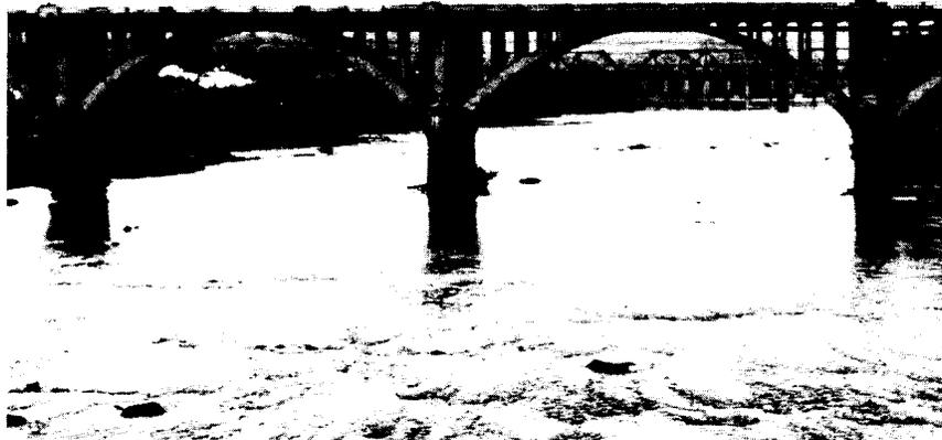
Figure 25. A long-span, open spandrel arch bridge designed by Daniel B. Luten for Danville, Virginia, in 1927. Luten designed arch bridges of filled, closed, and open spandrel types.
