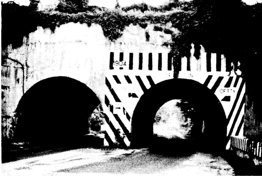
Figure 28. The earliest surveyed concrete arch bridge was this double arch underpass, built in 1904 in Stafford County.
