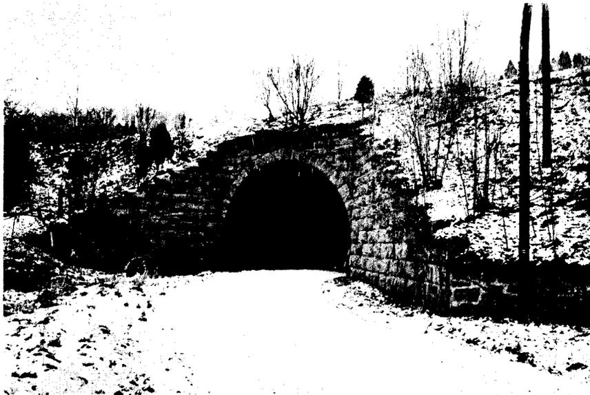
Figure 13. Also built at Honaker for the N & W's Clinch River line, this stone arch underpass exhibits mason's marks and is of typical late nineteenth century masonry construction.
