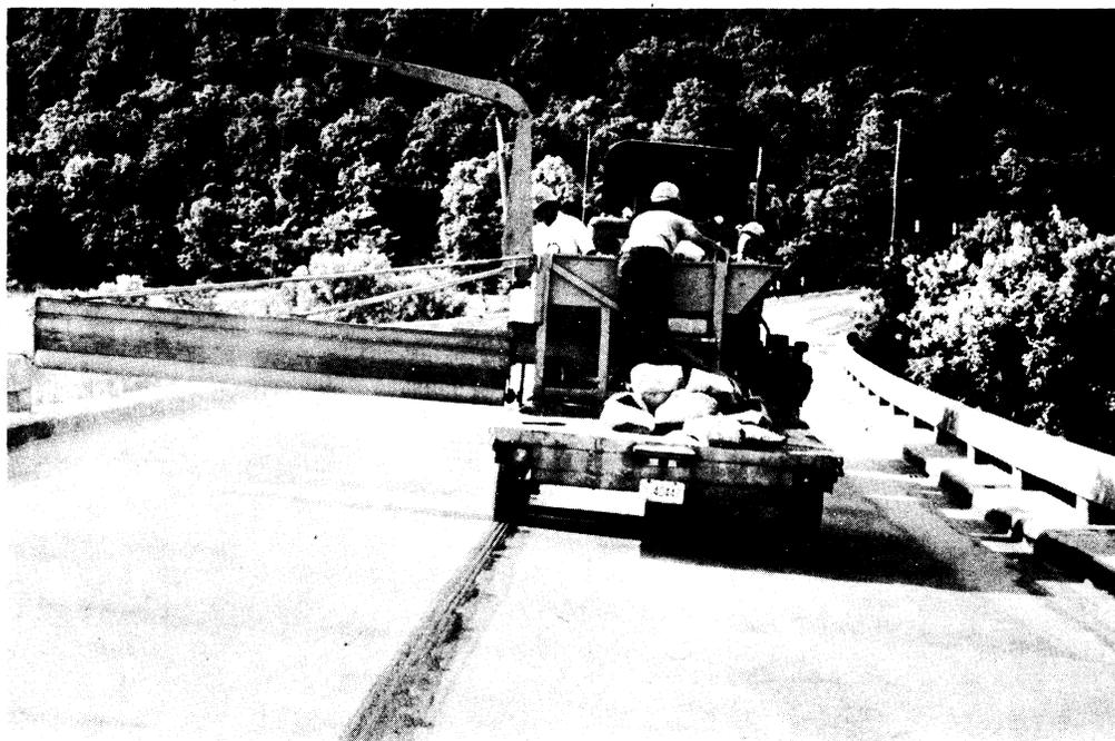
Figure 1. Application of resin and aggregate.
