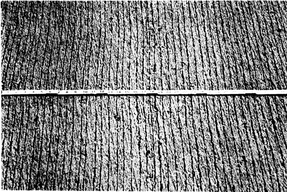
Figure 3. Deck surface texture with Bidwell tines.
