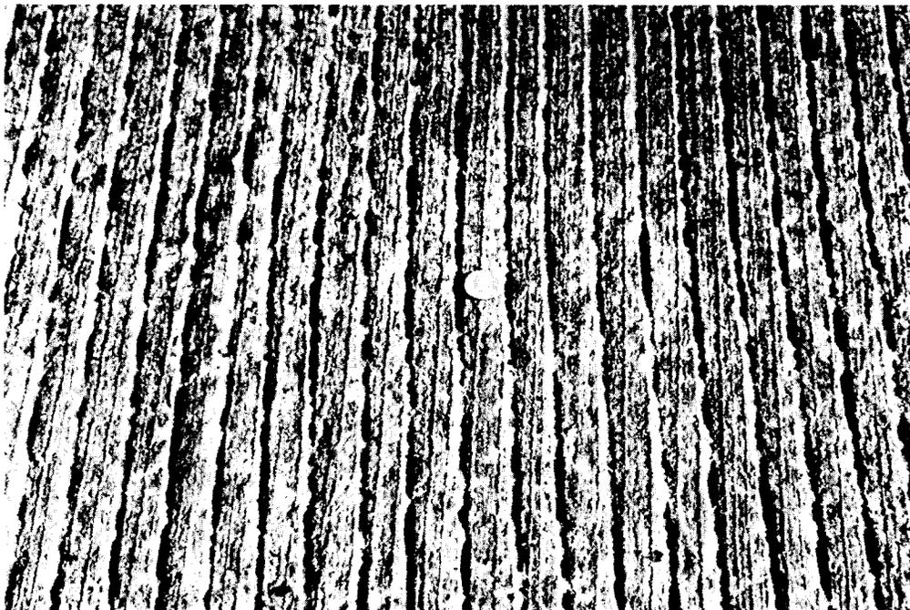
Figure 6. Deck striated with leaf rake.
