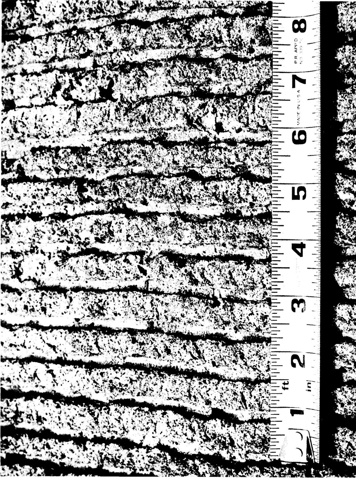
Figure 13. Full-size view of deck surface of the Pedlar River bridge on Route 60 is an example of a deck finish meeting the Virginia specification.
