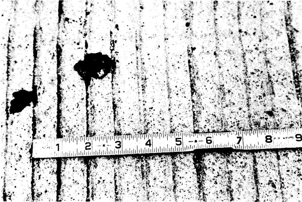
Figure 9. Striations produced by the tines shown in Figure 8.
