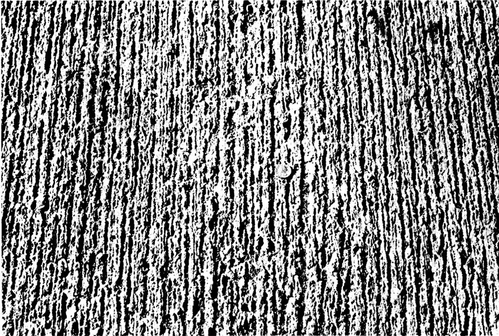
Figure 7. Scoring on deck of Route 220 NBL bridge over Route 419.
