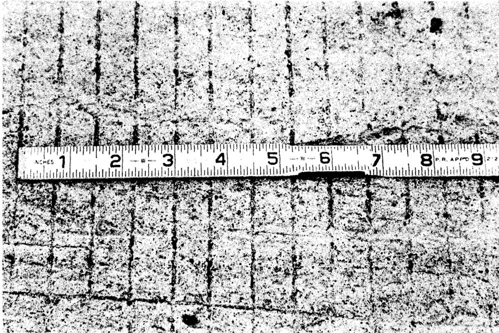
Figure 5. Close view of striations produced by beveled metal wheels.
