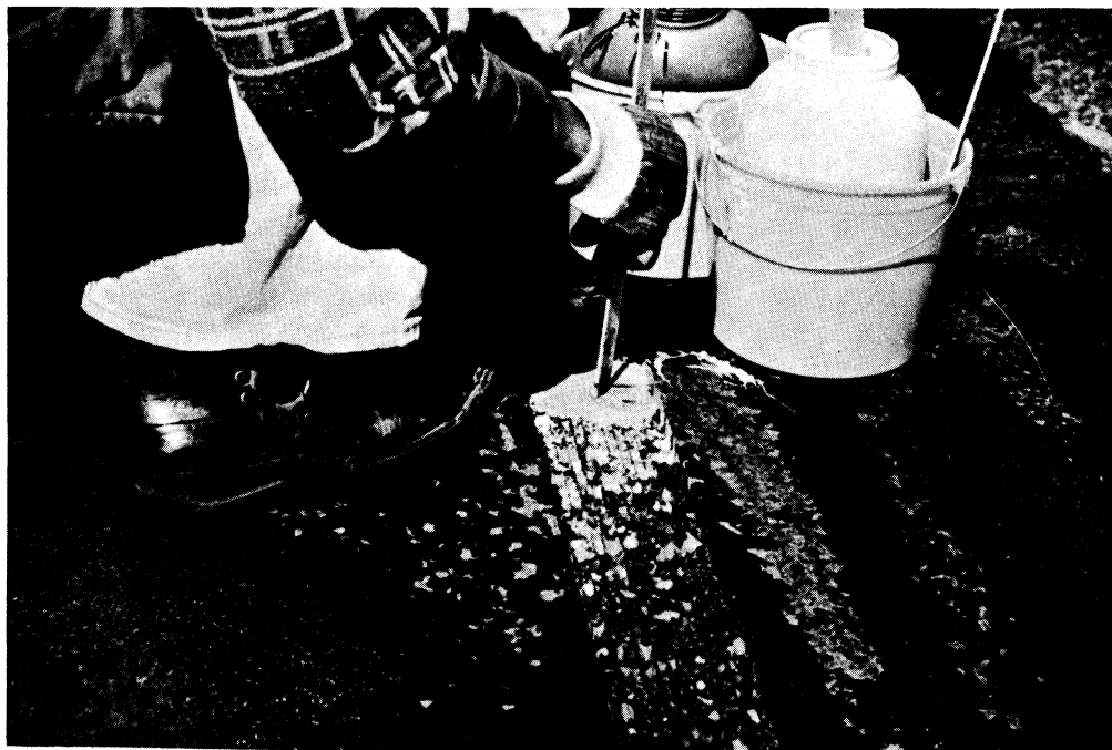
Figure 4. Epoxy adhesive being applied.
