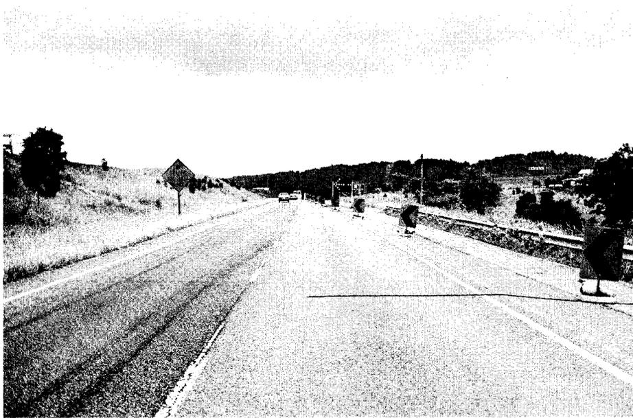
Figure A-8. Large chevron with black arrow — standard mount with 80-ft. (24.4-m) taper spacing.
