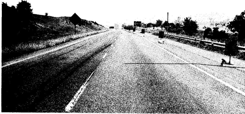
Figure A-3. Chevron with a black arrow — 40-ft. (12.2-m) taper spacing.
