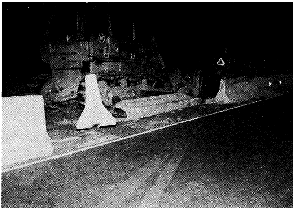
Figure 6. Two compact cars impacted the PCTB system at high speeds and large angles and caused the system to fail. (Virginia Department of State Police photo.)
