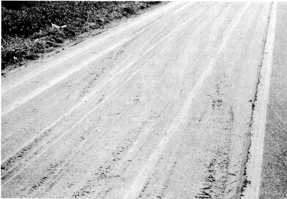
Figure 4. Mix showed good stability under rubber-tired roller.
