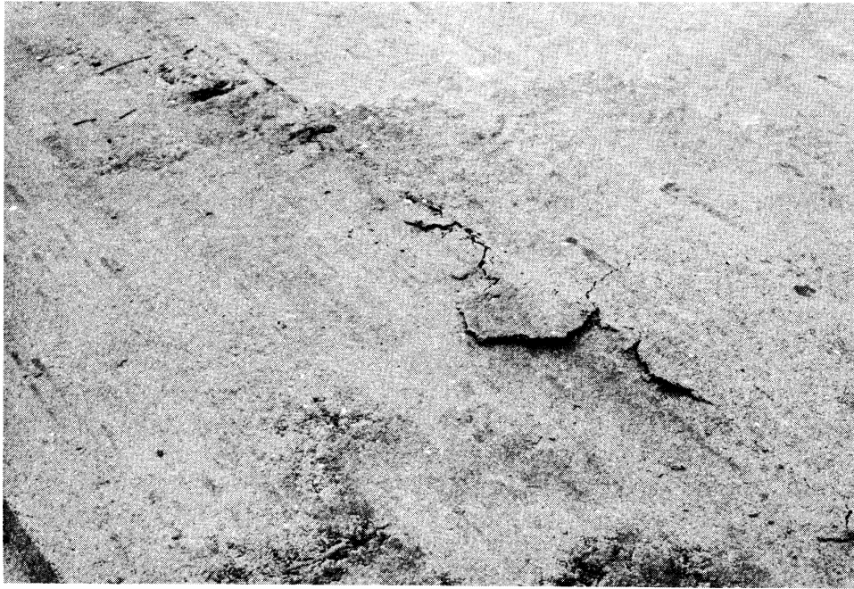
Figure 3. Flaking of mix under steel-wheel roller.
