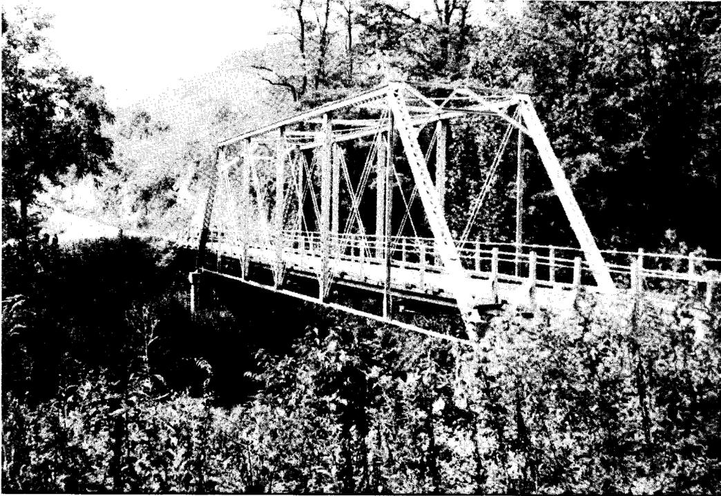
Figure 10. A single-span Pratt through truss built by the Penn Bridge Company of Beaver Falls, Pa.
