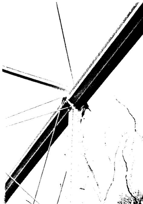
Figure 5. A detail of an upper joint on Bland County's second Phoenix Pratt truss.
