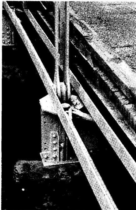
Figure 15. Lower joint connection detail of metal truss in Figure 14.
