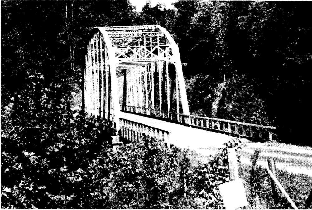
Figure 12. Parker truss, a variant of the Pratt truss, located in Lee County over the Powell River.
