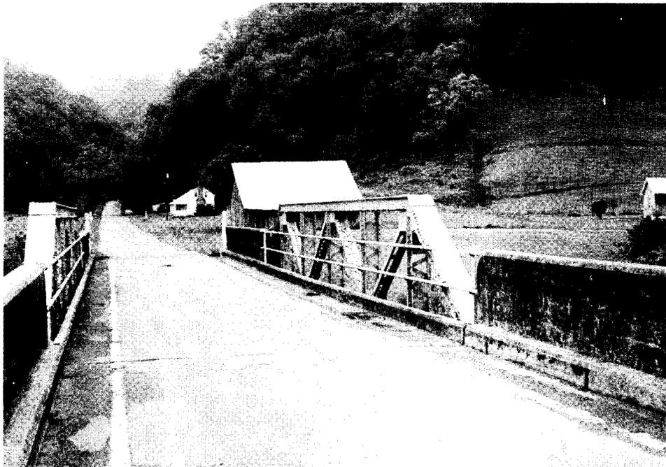
Figure 13. Pony truss span combined with two concrete spans in Scott County, over the Clinch River.
