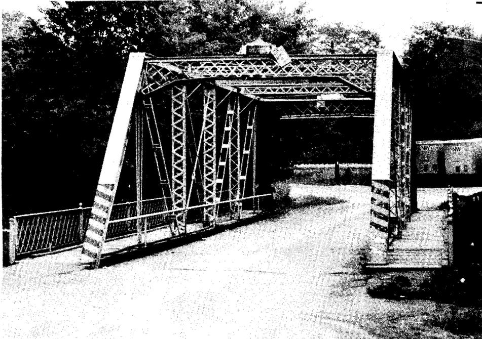
Figure 6. King Iron Bridge Company Pratt truss with bridge plate intact, built in 1885.
