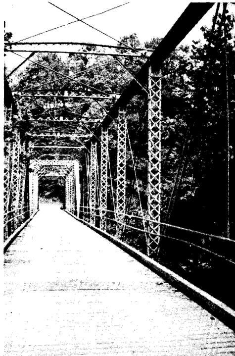
Figure 7. Groton Bridge & Manufacturing Company built this two-span Pratt truss in Russell County in 1889.
