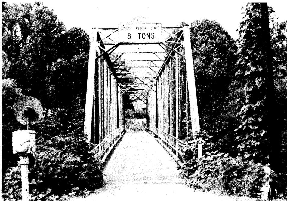
Figure 9. The Chicago Bridge Company built this two-span Pratt through truss in Russell County in 1891.
