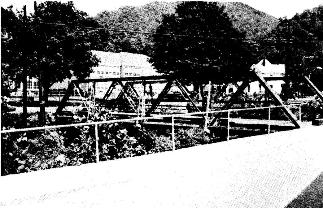
Figure 11. A typical twentieth century pony truss with riveted connections built by HIPCO Steel Bridges in 1925.
