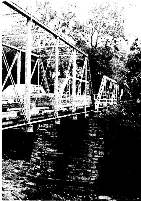
Figure 8. A two-span Pratt through and pony truss bridge built by the Pittsburgh Bridge Company in 1881. This is the district's earliest documented bridge.
