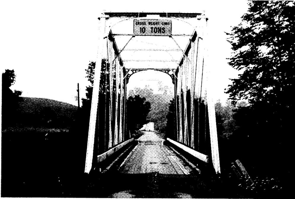
Figure 2. A Wythe County Pratt through truss attributed to the Phoenix Bridge Company.
