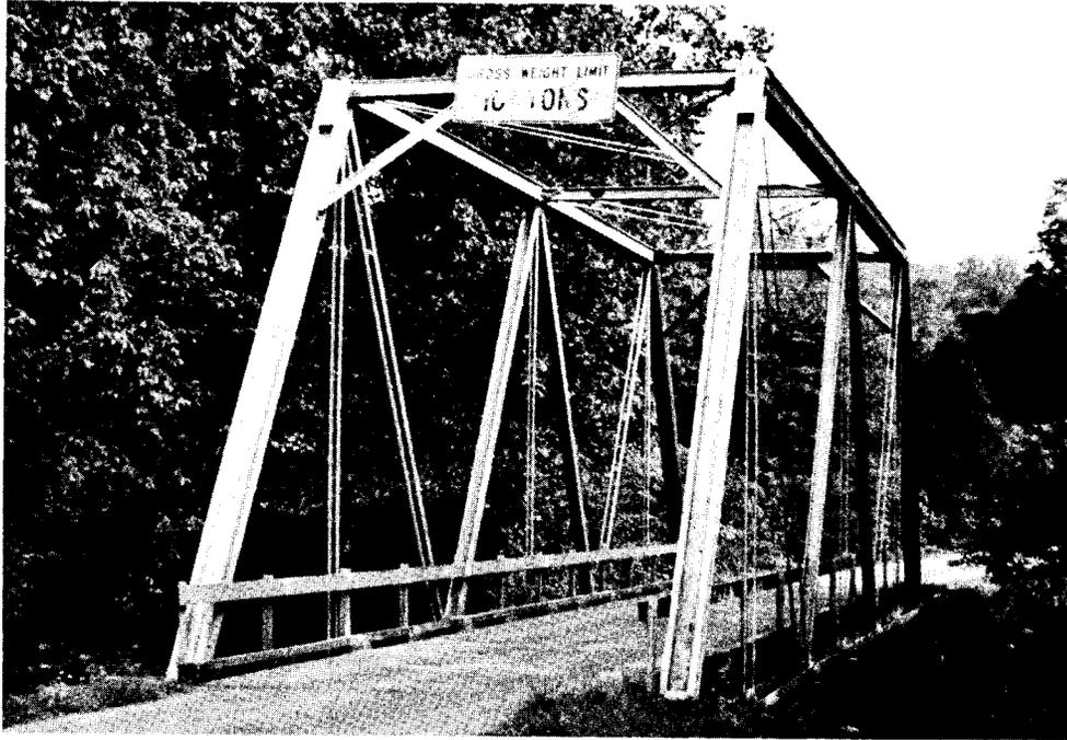
Figure 14. A heavily structured triangular with verticals through truss in Lee County.
