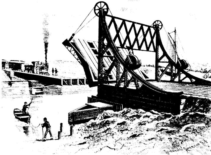
Figure 3. An example of an early counterweighted bascule bridge.
