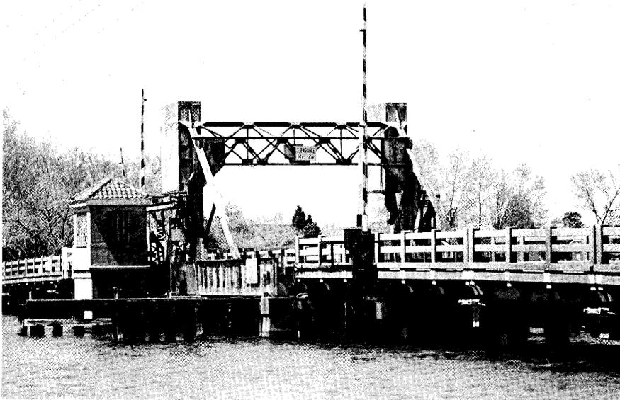
Figure 4. The Hodge's Ferry bascule bridge in Portsmouth, Virginia, is the only known Scherzer rolling-lift highway bridge in Virginia.
