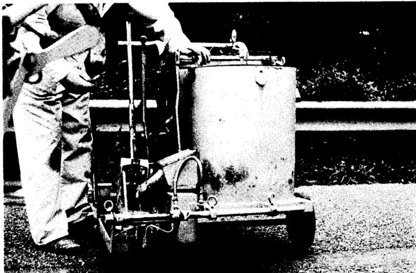
Figure 6. Machine for applying thermoplastic.
