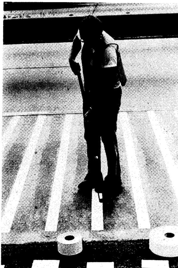
Figure 8. Applying preformed tapes.
