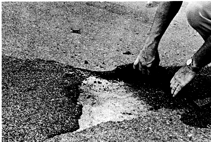
Figure 2. Disbonding prior to fabric installation, Route 81, Pulaski County.
