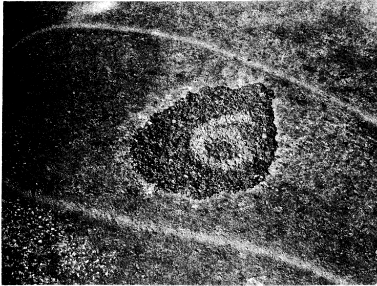
Figure 4. Distress 3 months after fabric installation, Route 81, Pulaski County.
