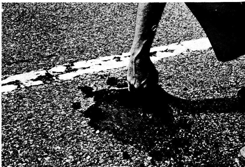
Figure 7. Disbonding of surface prior to installation of membrane, Route 460, Dinwiddie County.
