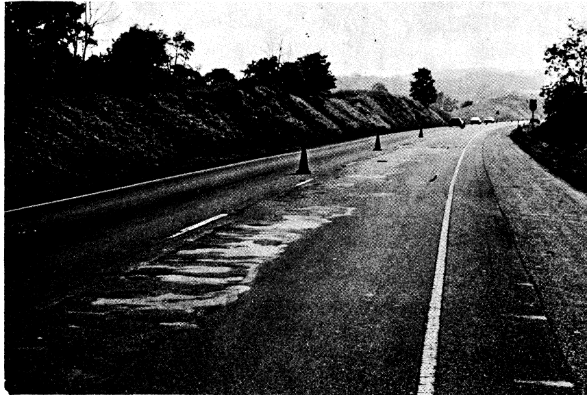
Figure 1. Distress prior to fabric installation, Route 81, Pulaski County.
