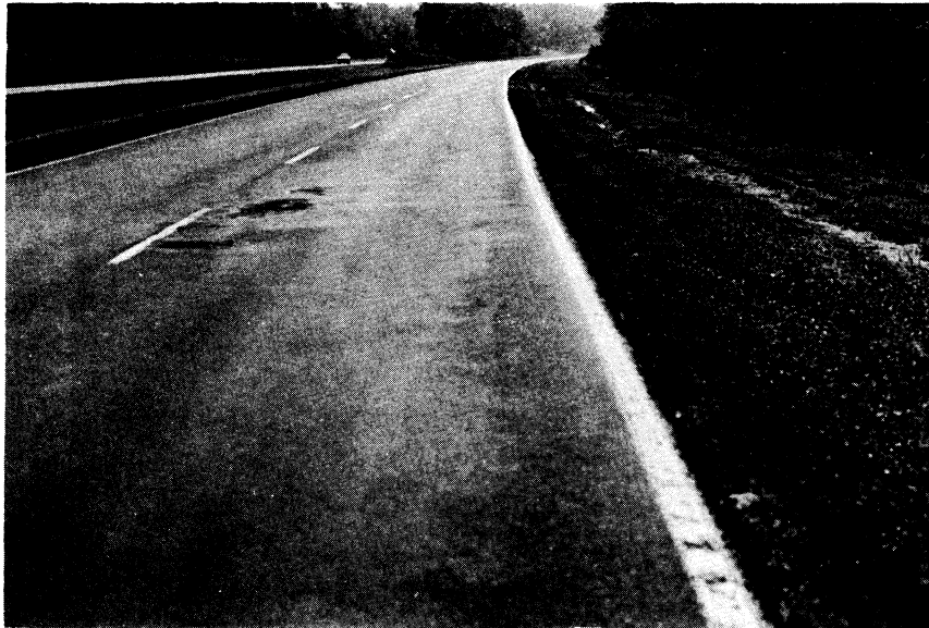
Figure 6. Distress prior to installation of membrane, Route 460, Dinwiddie County.
