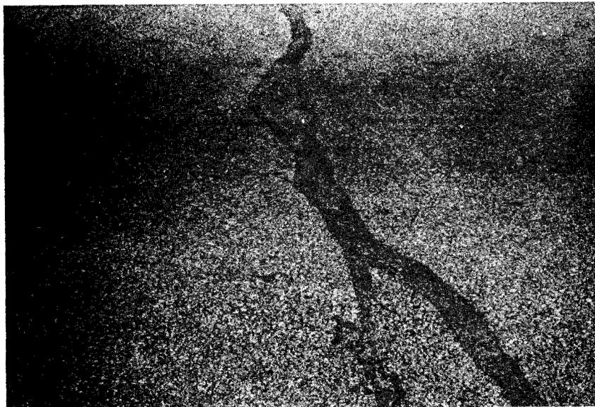
Figure 4. Severe transverse cracking (sealed) on section B of Project 7.
