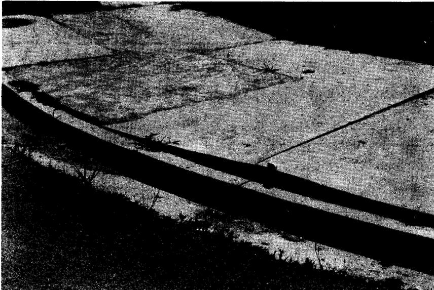
Figure 2. Sidewalk distortion due to undermining.
