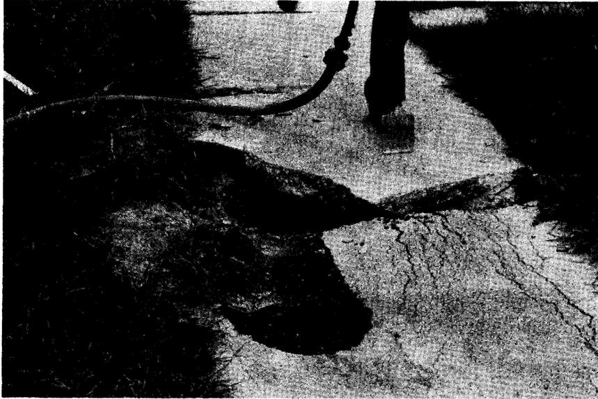
Figure 1. Severe sidewalk undermining.
