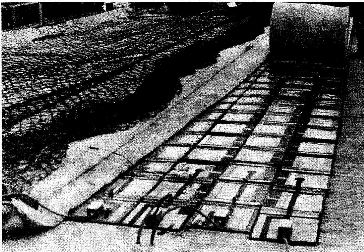
Figure 20. Heating blankets on deck with insulation and netting.
