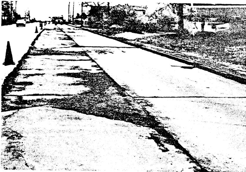
Figure 8. Road mix material in passing lane at same elevation as traffic lane.
