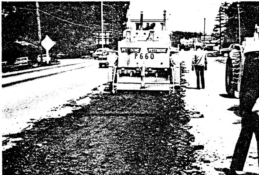
Figure 4. Pettibone pulverizer in use.
