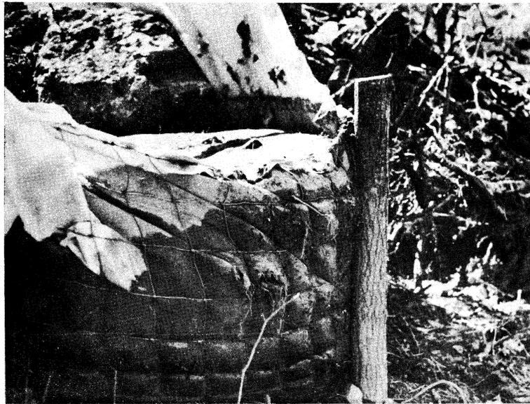
Figure 1. Silt fence filter barrier filled with sediment. Trap efficiency is greatly reduced.
