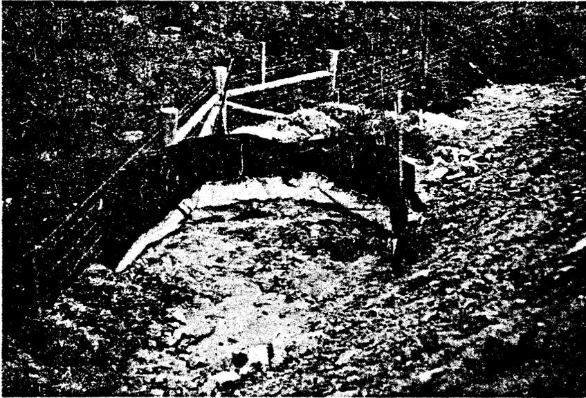
Figure 3. Filter fabric silt fence working well. However, lack of access for equipment will likely make cleaning of fence difficult and costly.
