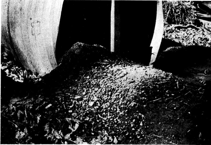
Figure 7. Accumulation of sediment in drain pipe at outlet end. Placing pipe at a slightly higher elevation would help eliminate this harmful buildup of sediment.
