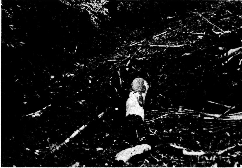
Figure 6. Brush and root mat barrier windrowed at the toe of a fill.
