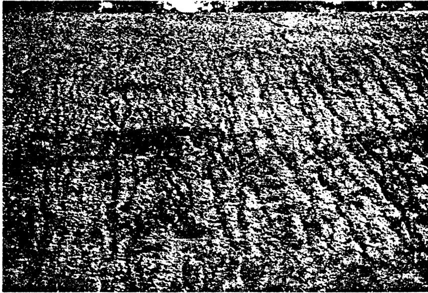
Figure 4. Rill erosion on a cut slope resulting from lack of vegetative cover. Early seeding will usually eliminate this type of slope erosion.
