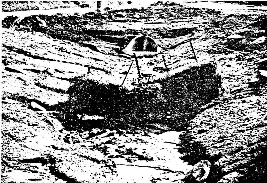
Figure 5. Severe erosion and sediment loss caused by undercutting of a straw bale barrier. Proper installation of this type of barrier will minimize failures of this type.
