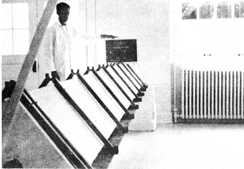
Figure 3. Stiffeners for girder mounted on mandrel prior to winding tension elements.
