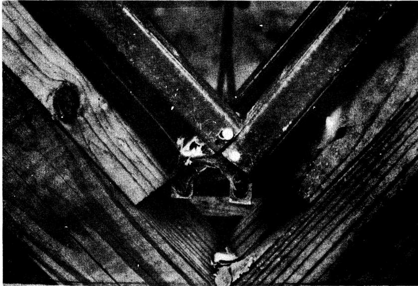
Figure 8. End view of girder showing failure of a joint at a lower chord connector due to seat bearing load.
