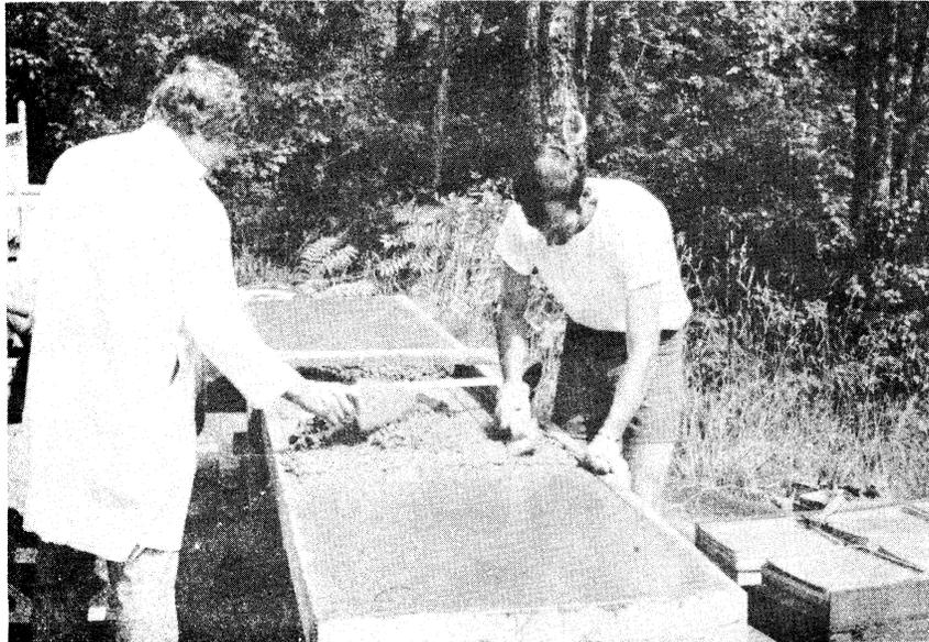
Figure 5. Placing the concrete deck on top flange plate.
