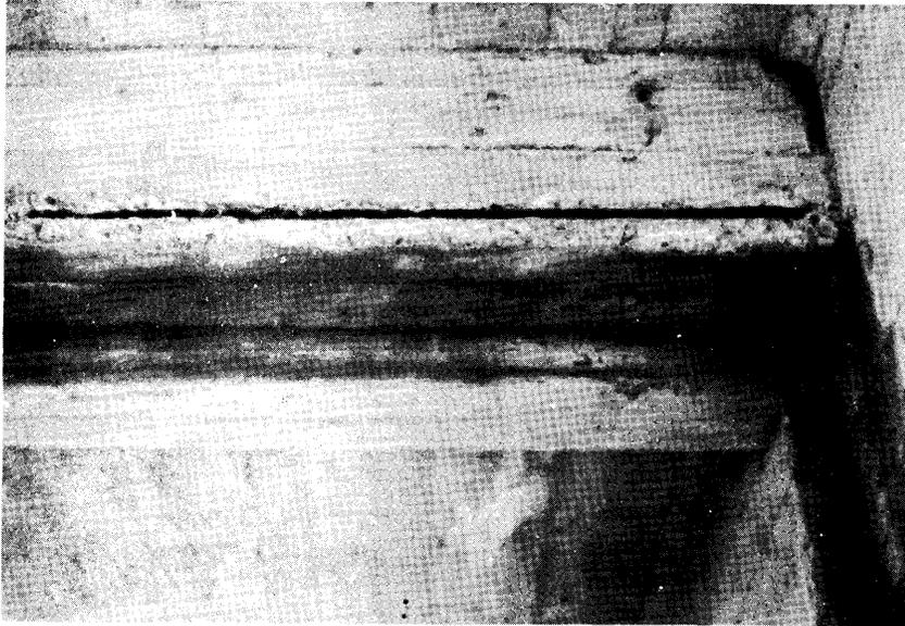
Figure 8. Spalling of concrete on the end diaphragms baring reinforcing steel.
