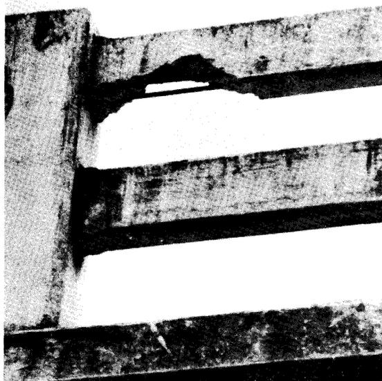
Figure 10. Deterioration of concrete railing baring reinforcing steel.
