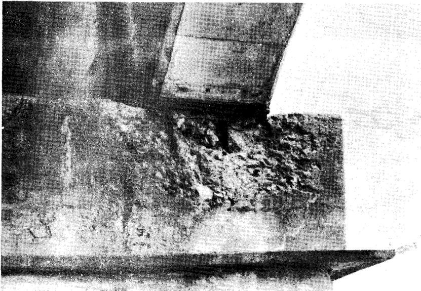
Figure 9. Spalling of concrete on the pier cap baring reinforcing steel.
