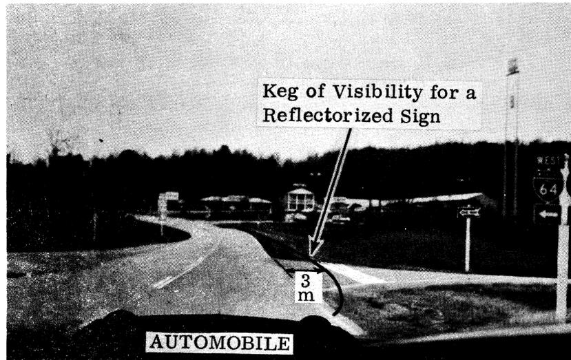
Figure 5. The zone of keg of visibility shows that the one-way sign and stop line would not be visible at night and hence both are redundant. (1 m=3.3 ft.)
