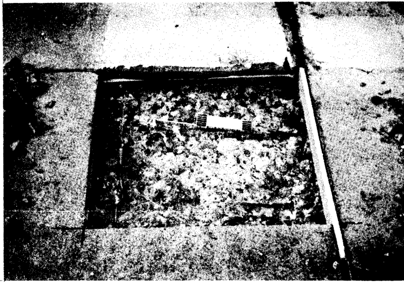
Figure 5. Proper insertion of styrofoam to form transverse joint (right) and polyethylene strip to form centerline joint (top).
