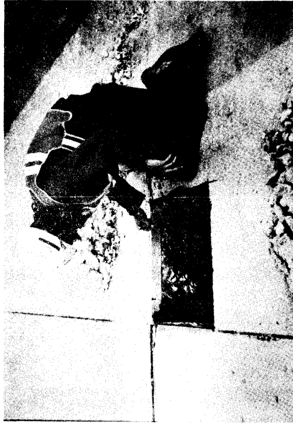
Figure 17. Thin coating of cement paste improves early bond development between repair concrete and pavement.
