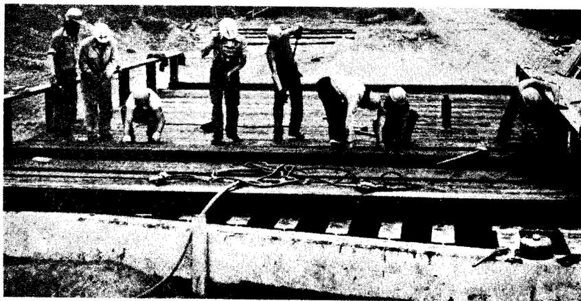
Figure 25. Timbers placed and connected to steel stringers over Elkhorn Creek on Rte. 686 in Pittsylvania County.
