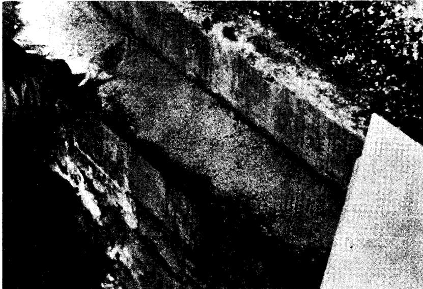
Figure 19. Epoxy and shims placed on building paper to correct for nonuniform bearing between slab and abutment.
