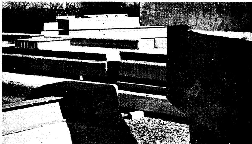
Figure 11. Exterior beam with curb cast in slab. Guardrail and post are attached in field.
