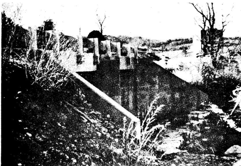
Figure 4. Two-span precast slab bridge on Rte. 724 near Harrisonburg.
