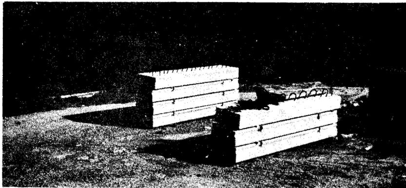
Figure 10. Exterior beam with a few large parapet bars cast in slab.
