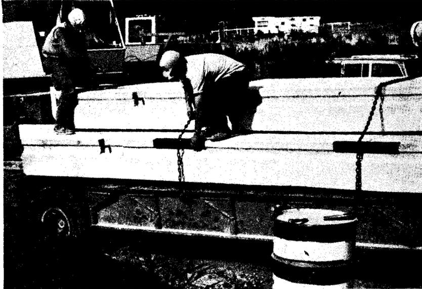
Figure 18. Three slabs properly secured to lowboy trailer.
