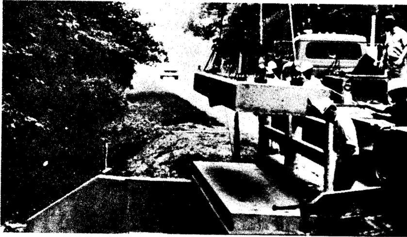
Figure 23. Precast slab being installed by Suffolk District bridge crew to widen Rte. 58 over Spivy Swamp.
