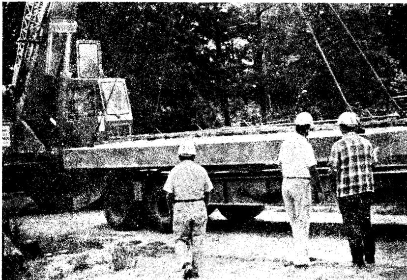
Figure 15. Truck crane lifting precast slab.
