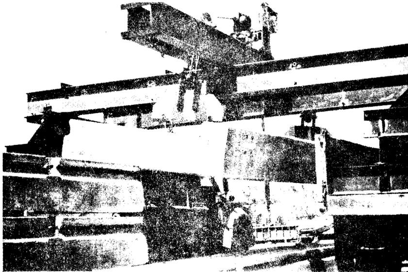
Figure 16. Gantry crane moving precast slab from storage area to trailer.
