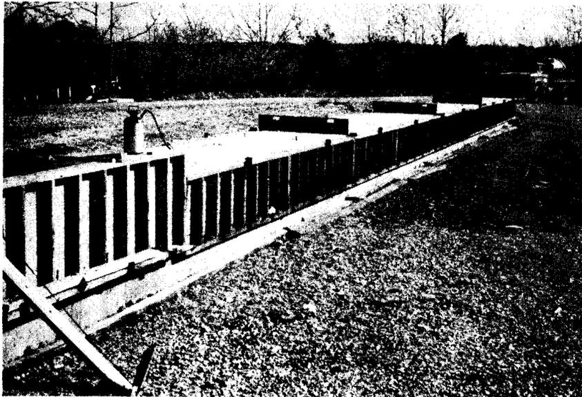
Figure 8. Staunton District casting form with concrete bed.
