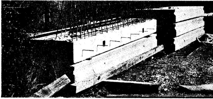
Figure 9. Exterior beam with all the parapet steel cast in slab.
