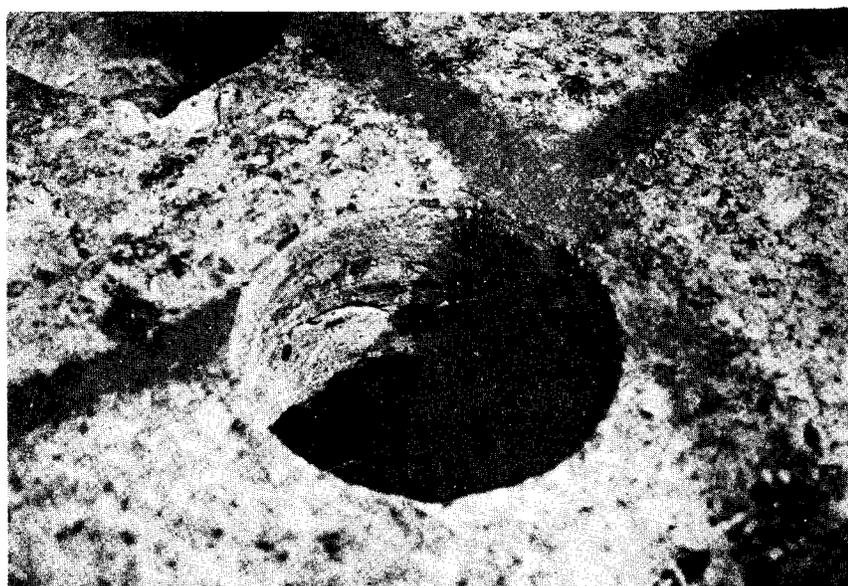
Figure 6. Close-up of incipient spall in Figure 5.
