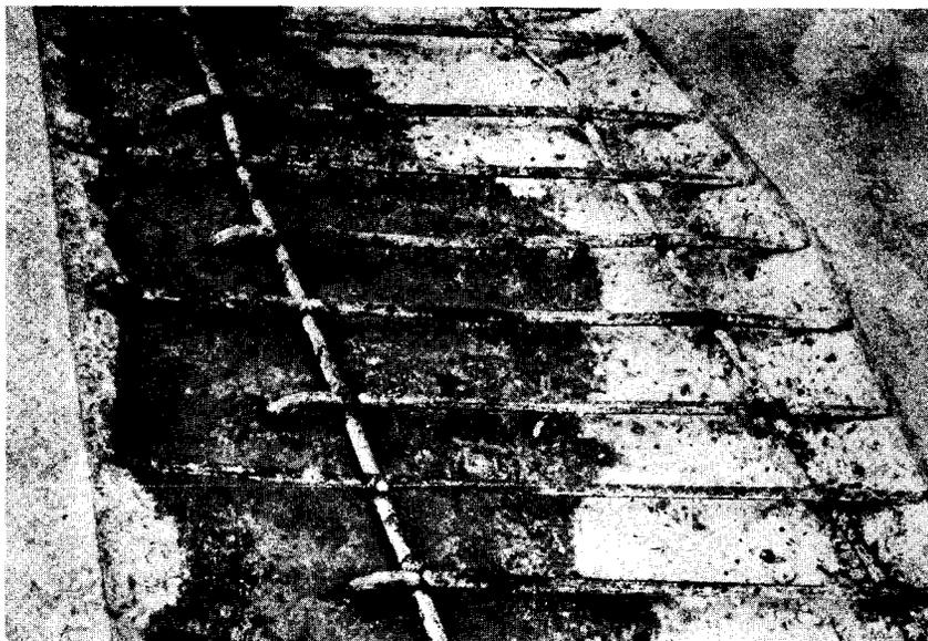
Figure 8. Close-up of reinforcement showing variable corrosion.
