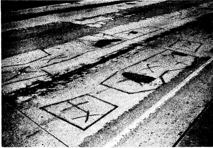
Figure 4. Area of moderate to severe spalling.
