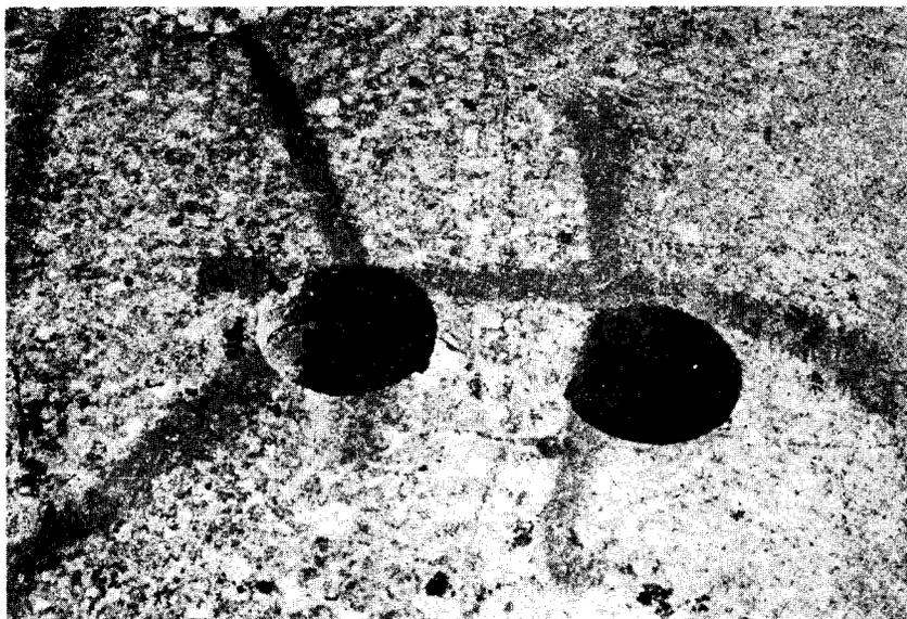
Figure 5. Core holes showing incipient spall.
