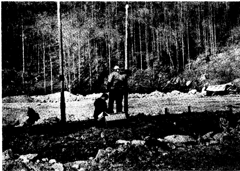
Figure 29. Four arrays of plastic tubes being installed.
