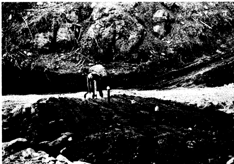
Figure 30. Backfill around the four arrays of tubes.
