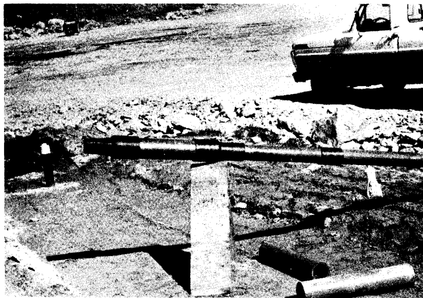
Figure 28. Plastic tubing, connecting sleeve, and rubber boots.
