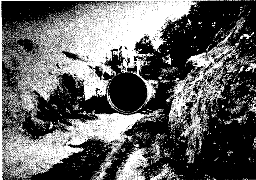
Figure 15. Backfilling and straw placement around concrete culvert.
