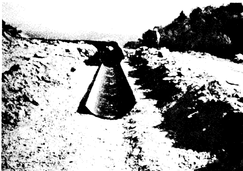
Figure 10. Invert sections in place.
