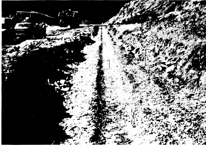
Figure 9. Prepared bedding for steel culvert.
