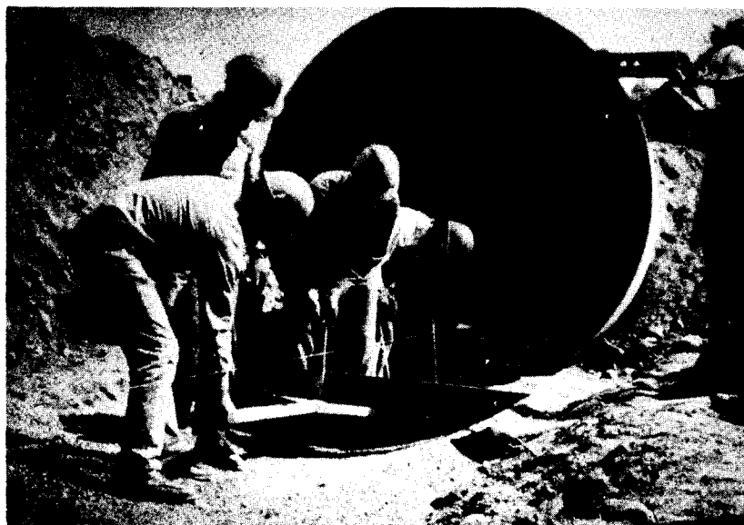
Figure 14. Preparation of bedding for concrete culvert.
