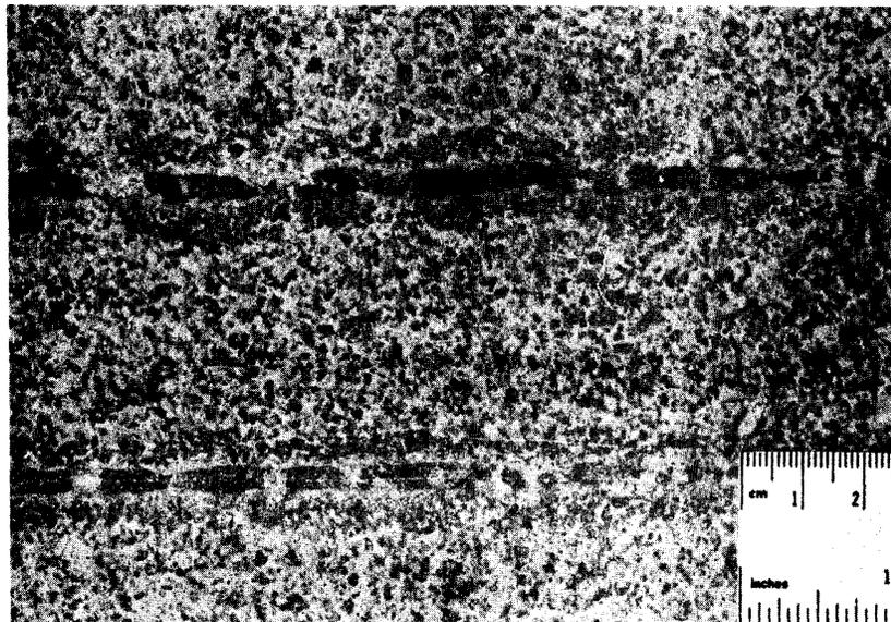
Figure 14. Transversely tined texture with grooves on 38 mm (1 1/2 in.) centers. Site 9.
