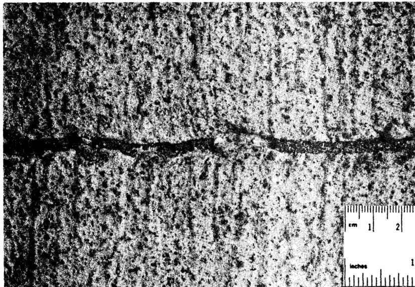
Figure 7. Transversely tined texture, grooves spaced on 76 mm (3 in.) centers. Site 2.
