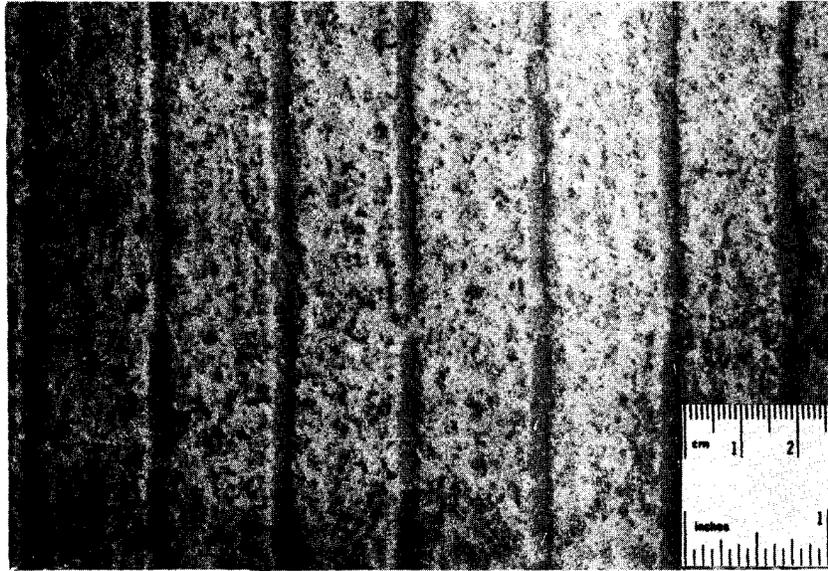
Figure 6. Longitudinally tined texture, grooves spaced on 19 mm (3/4 in.) centers. Site 1.
