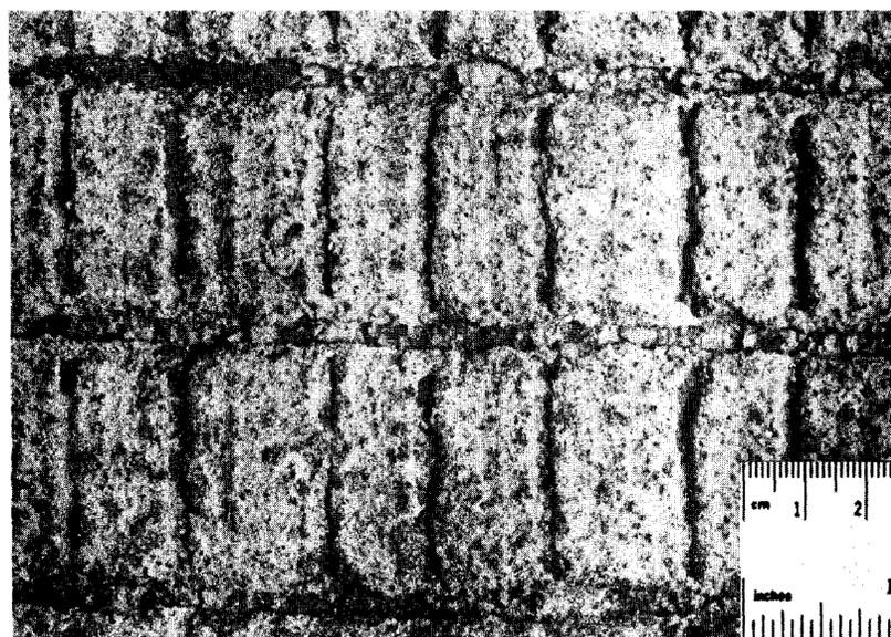
Figure 15. Tined texture with grooves spaced on 19 mm (3/4 in.) centers longitudinally and 38 mm (1 1/2 in.) centers transversely. Site 10.
