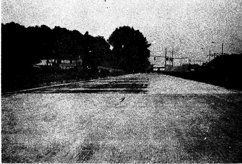
Figure 16. Contrast during rain between tined texture with grooves on 19 mm (3/4 in.) centers longitudinally (background) and tined texture with grooves on 19 mm (3/4 in.) centers longitudinally with 76 mm (3 in.) centers transversely (foreground).
