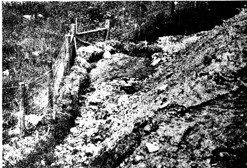
Figure 8. Construction area before installation of first silt fence.
