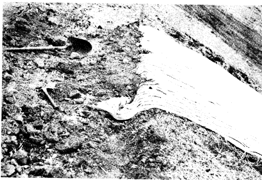
Figure 2. Anchoring Hold/Gro in the trench.
