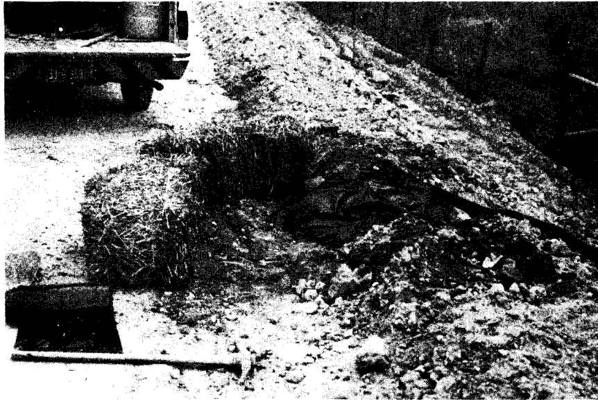
Figure 6. Inlet end of temporary downdrain.
