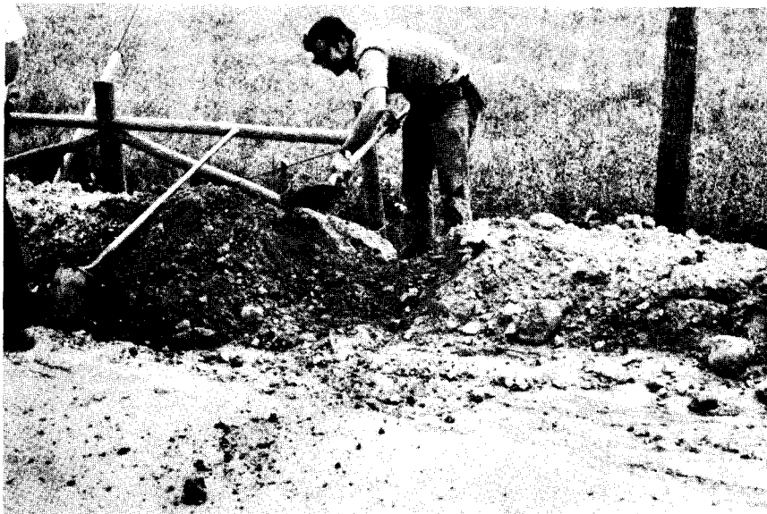
Figure 5. Temporary downdrain channel.
