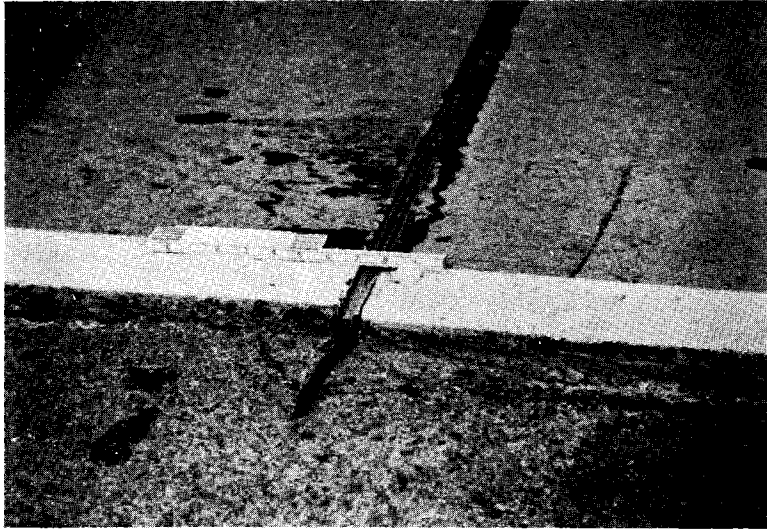
Figure 12. Joint faulting.
