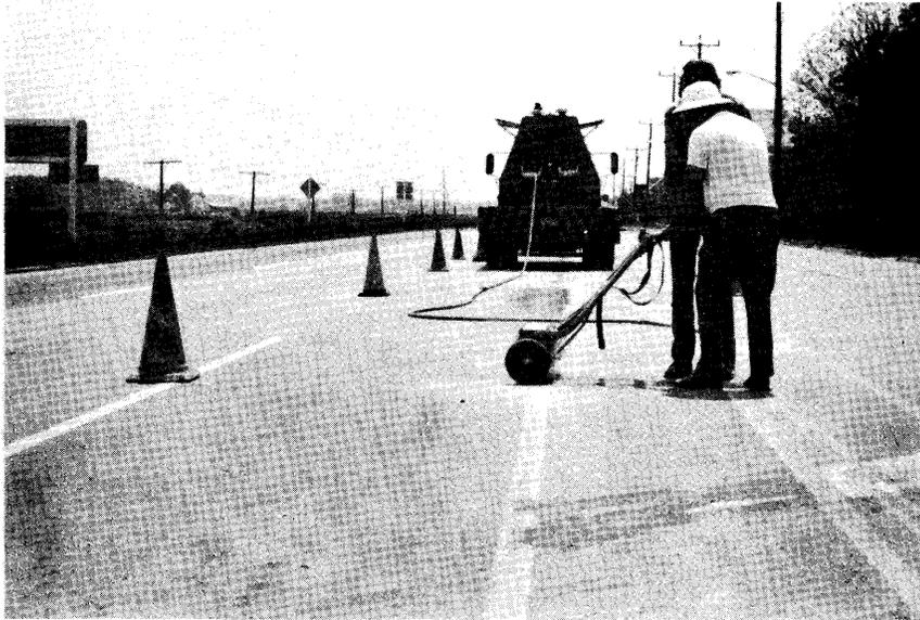
Figure 6. Removal of paint markings from bituminous pavements on Route 13 in Accomac County, Virginia.
