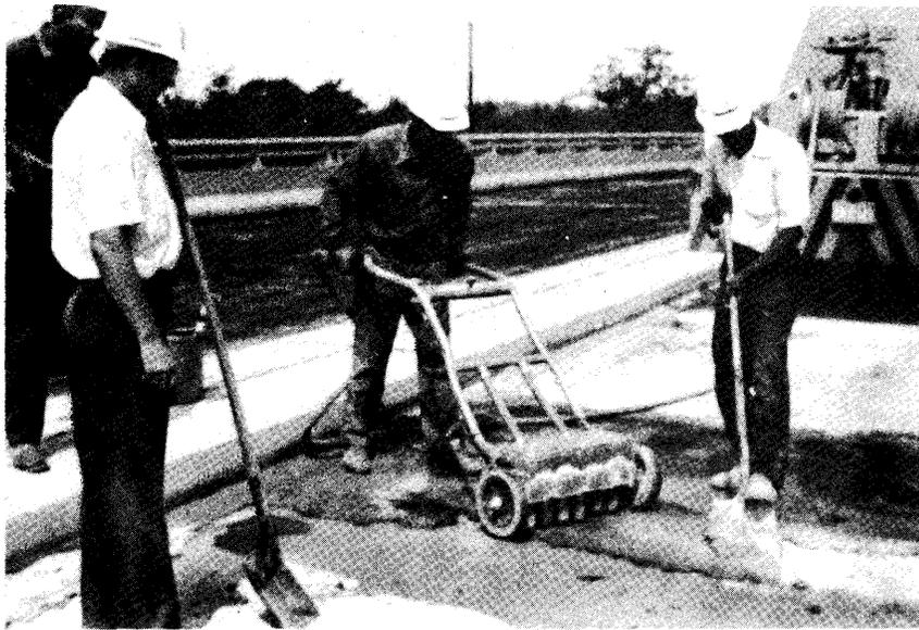
Figure 9. Cleaning operation on the Route 58 bridge. Note that the loose material must be removed with a shovel.
