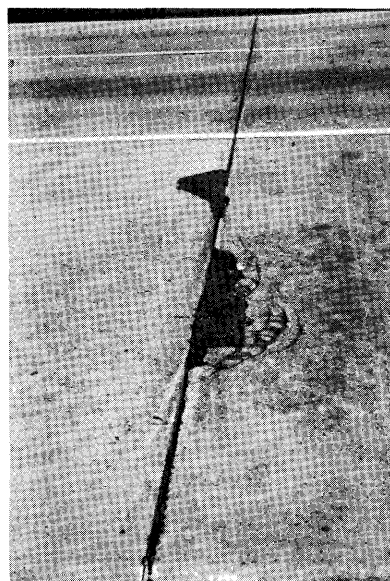
Figure 9. Semicircular (half-moon) spall caused by insert corrosion.
