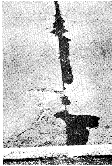
Figure 11. Corner break in left foreground with extensive spall and probable full-depth deterioration extending from corner break.
