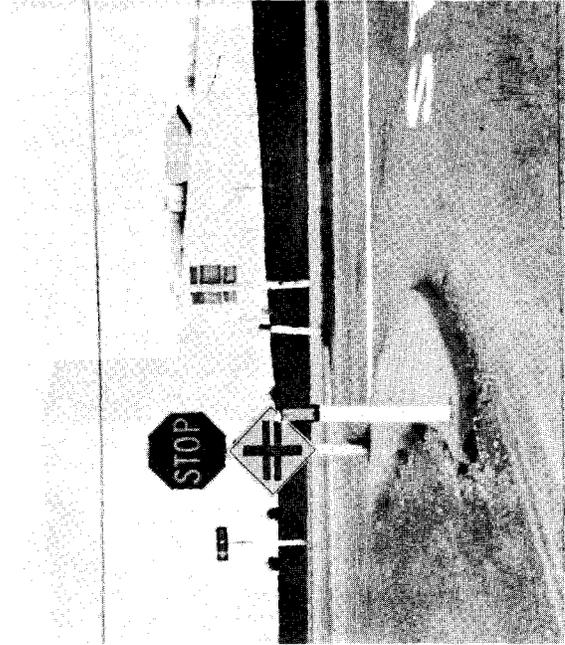
Figure 18. Suggested improvement to interchange shown in Figure 17 by addition of crossroad sign. If found desirable, left turn sign could be added.
