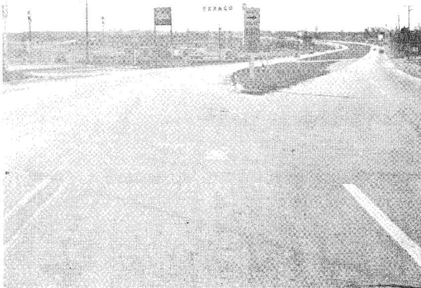
**Figure 19.** Route 58 at South Hill. Day photograph of transition from 3-lane undivided highway to a 4-lane divided highway with no transitional pavement marking.
