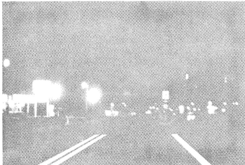
**Figure 20.** Route 58 at South Hill. Night photograph of the transition from 3-lane undivided highway to a 4-lane divided highway with no transitional pavement marking. Site of wrong-way entry.
