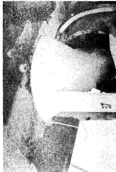
(c) Second vibrating chute being inserted into ready-mix truck drum.
