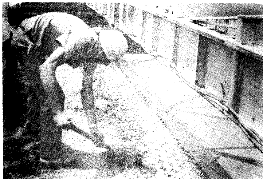
Figure 15. Rapid depositing of overlay concretes (above). Some handwork required ahead of screed to maintain maximum overdepth of approximately 2 inches (below).
